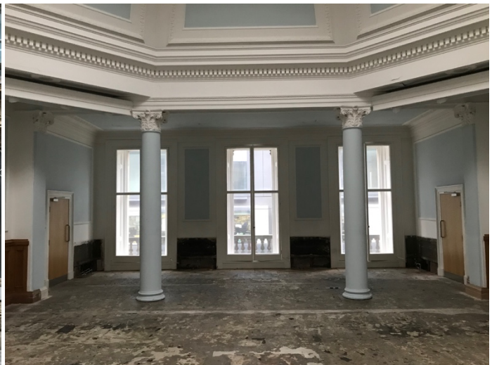
Figure 3: Picture of Second Floor domed room
