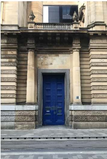
Figure 4: Existing roof terrace photo from street level
