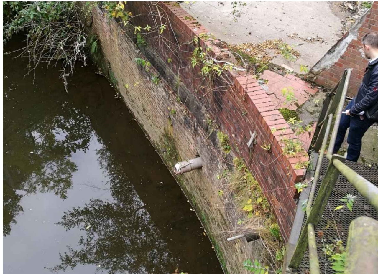
Figure 5-1 Existing Outfall Observed During Site Visit
