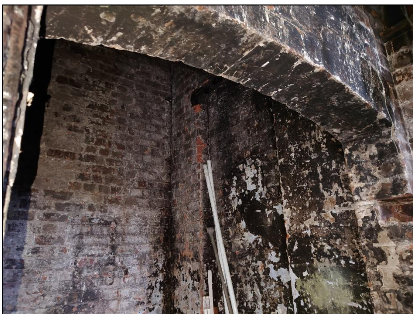
Photograph 6 showing the internal brickwork
