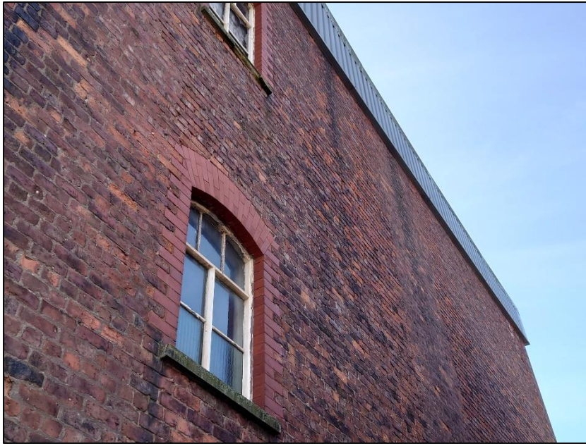
Photograph 2 showing the rear elevation of the property
