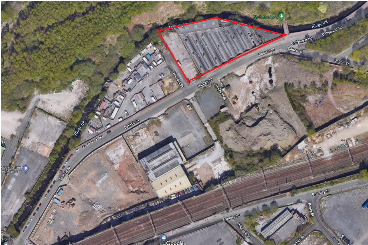
Figure 2 – Theos Timber Yard, Dantzic Street – Consolidation Centre
