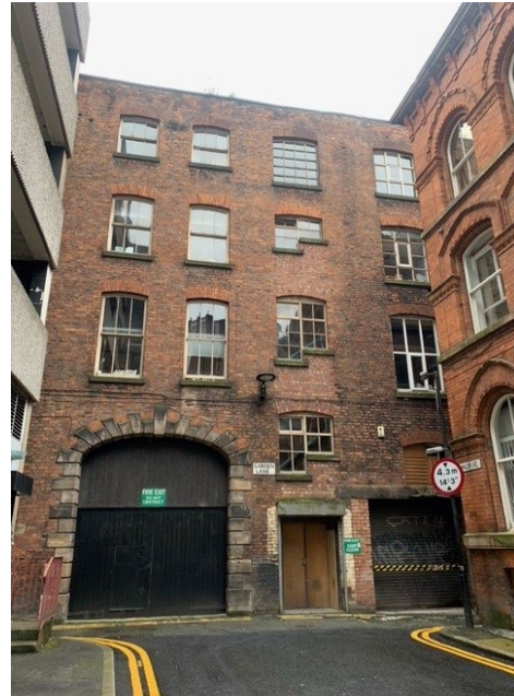
^ Figure 2.4 – View along Dunlop Street
