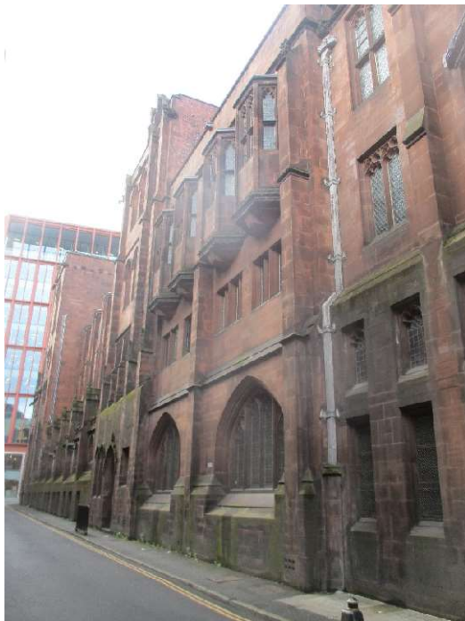
Wood Street (north) elevation viewed from the north-west
