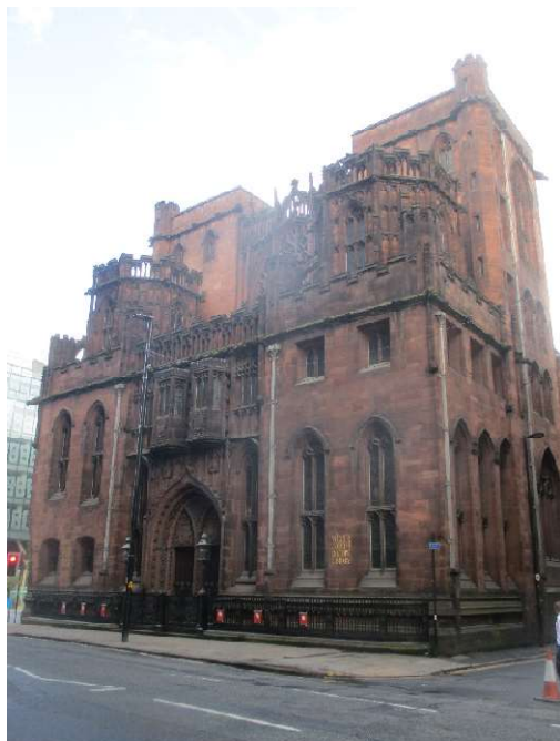
Deansgate (east) elevation viewed from the north-east
