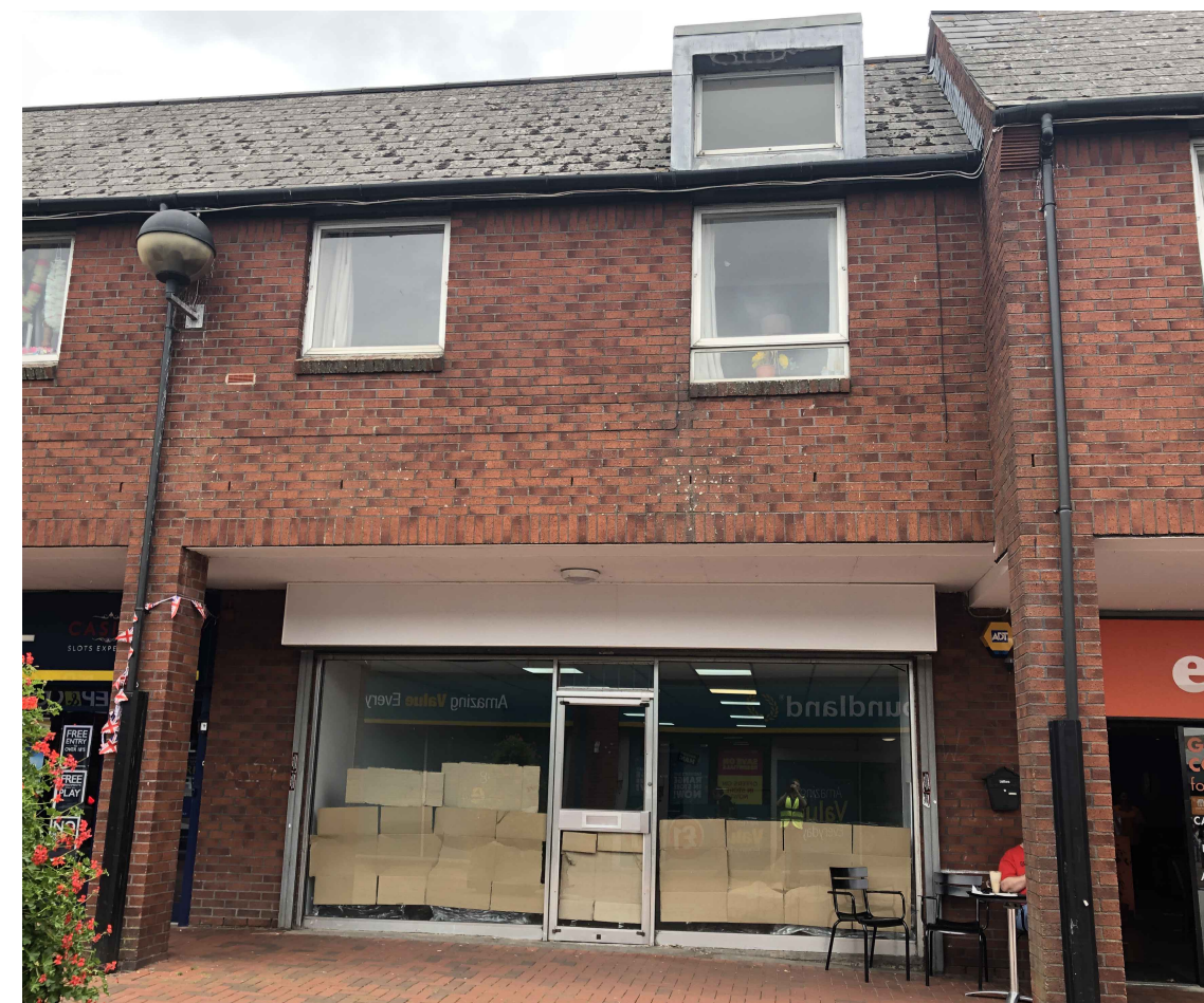
Existing Shop Front - Photo
