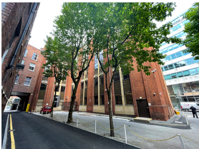
Image 5: Photograph showing proposed location of extension to rear of 125 Portland Street. To the left hand side is the rear and less significance elevation of neighbouring listed building at 127-133 Portland Street.
