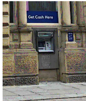
6 EXTERNAL PHOTO EXISTING
