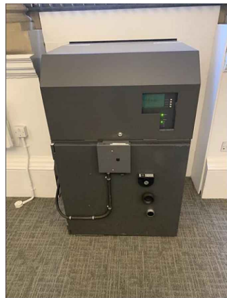
7 INTERNAL PHOTO EXISTING
