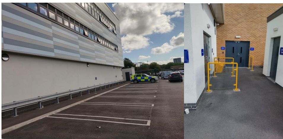
Fig. 1 – The application site and returning section to the north-east elevation
