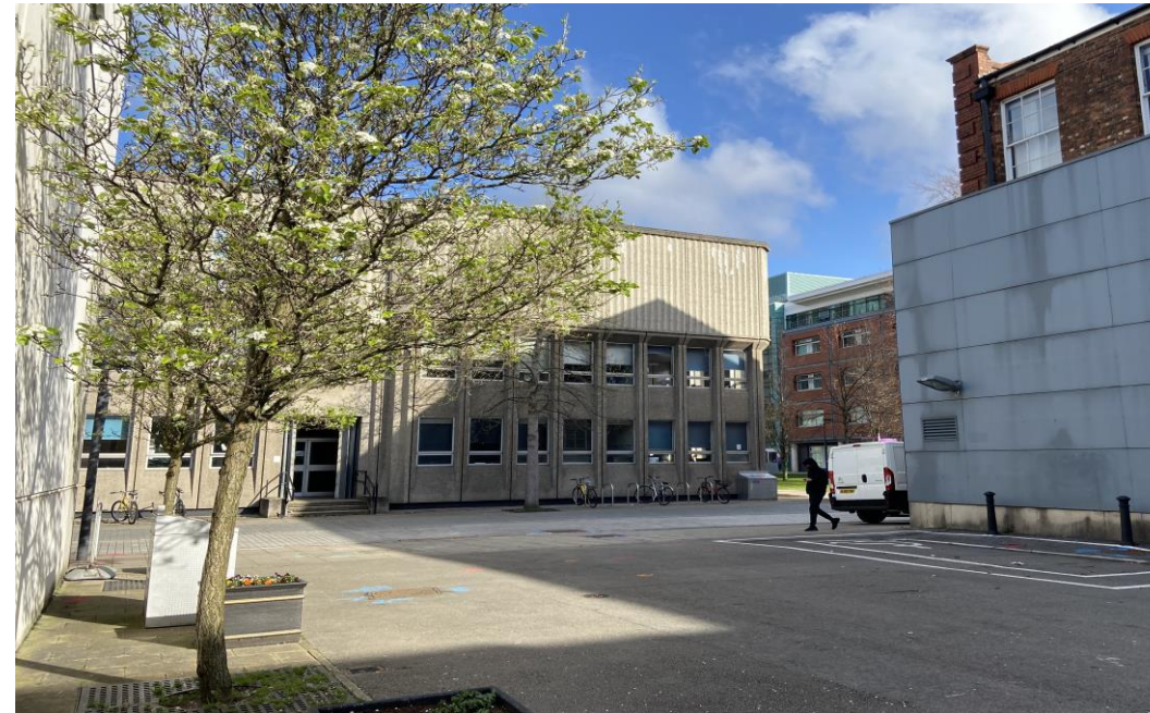
View 3 – Looking north from within the site (MHMC courtyard)
