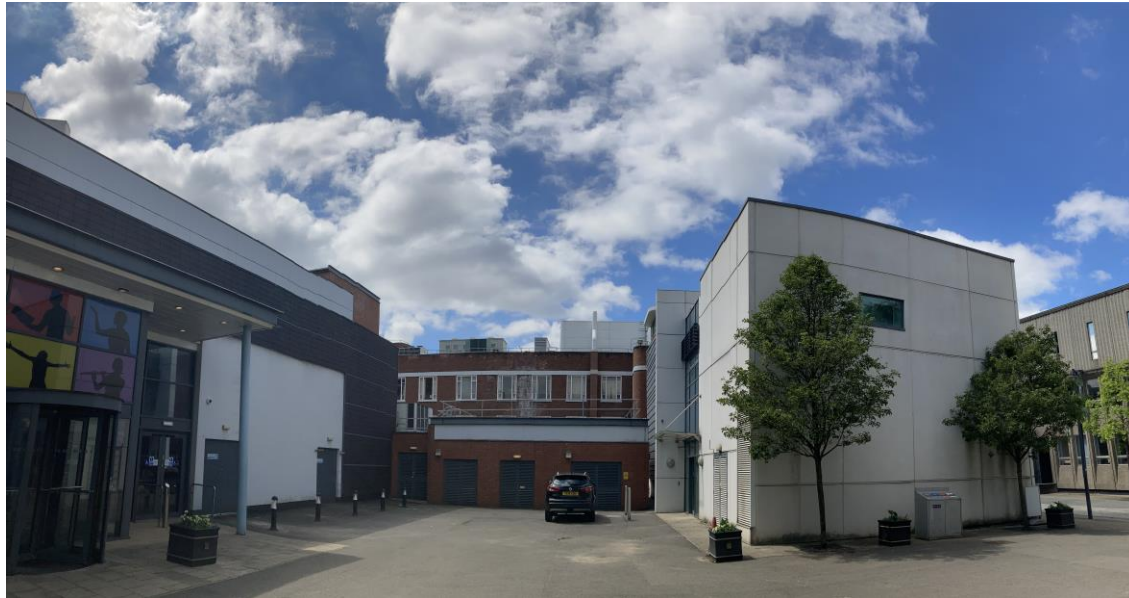
View 1 – Panoramic view looking west to the site courtyard
