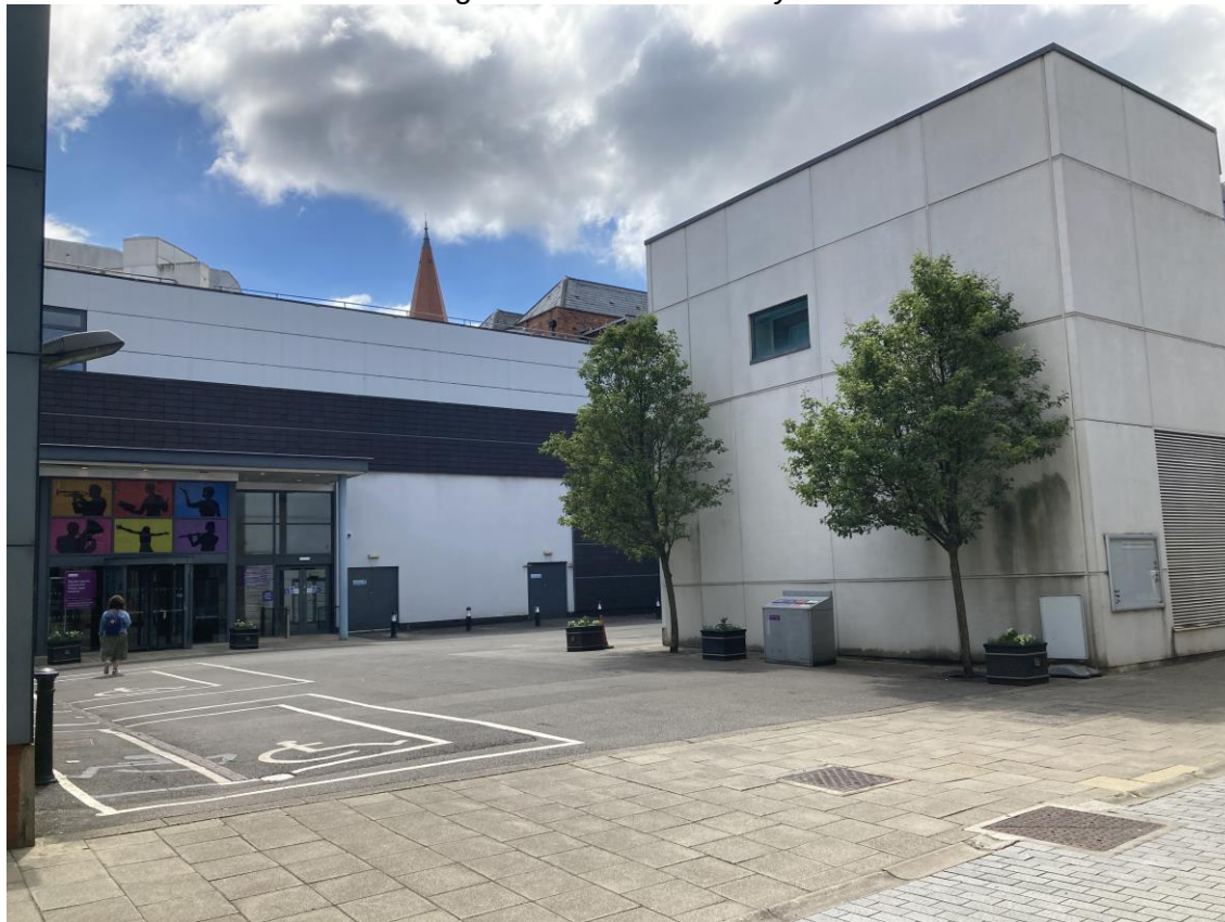
View 2 – View of the site access point and existing disabled parking bays
