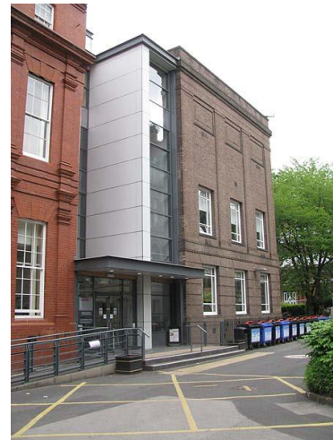
The New Physics Laboratory (View 3)
