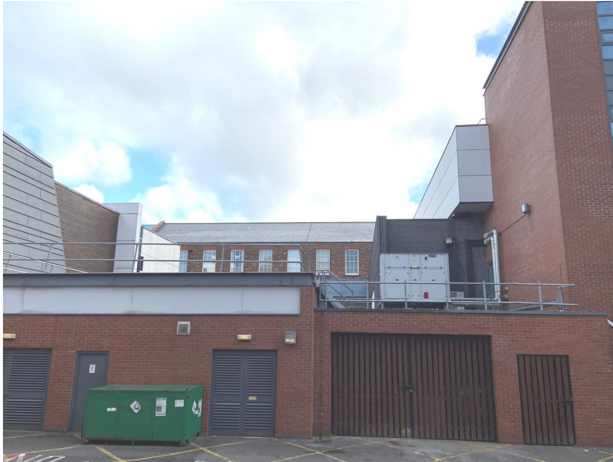
View 5 – View looking east from outside the site from the other side to the substation (Higher Chatham Street)
