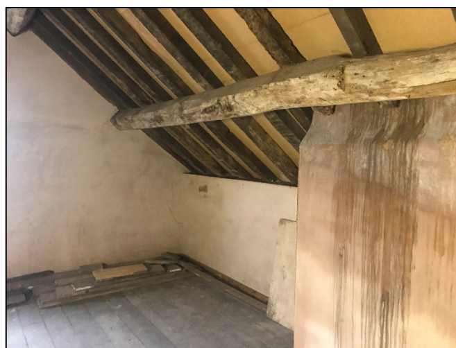
Figure 7: Location of where the aspirating unit will be attached to the wall.
