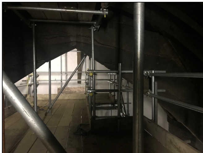
Figure 3: Roof space in the main hall.
