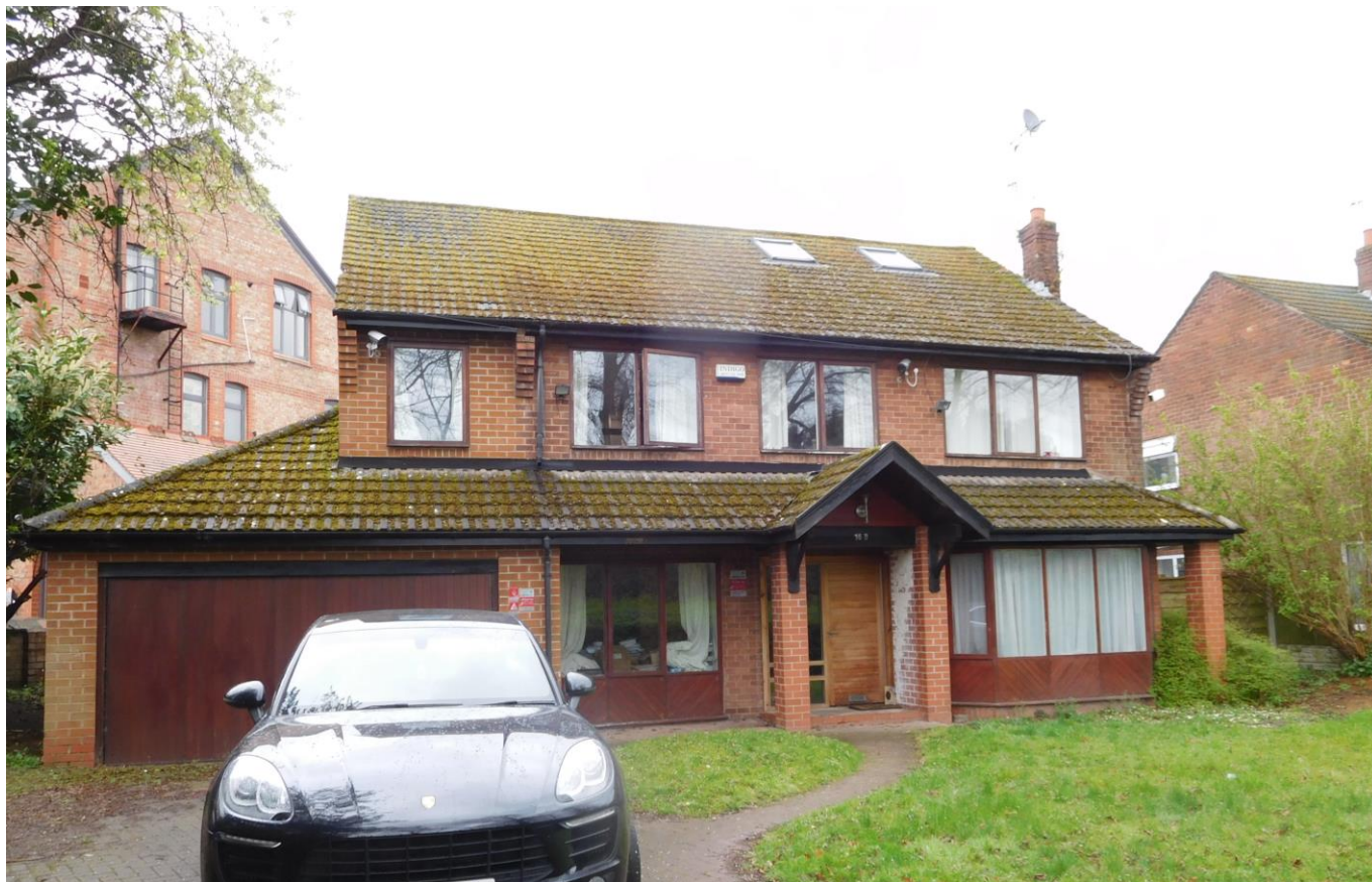
Photograph 1 Front Elevation of dwellinghouse as viewed from Darley Avenue, site photograph as taken 5 th April 2020
