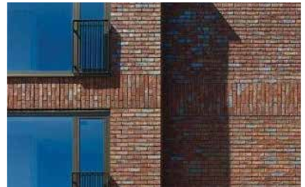
Header course feature bands
