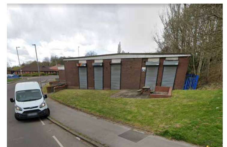
Existing building from White Moss Road
