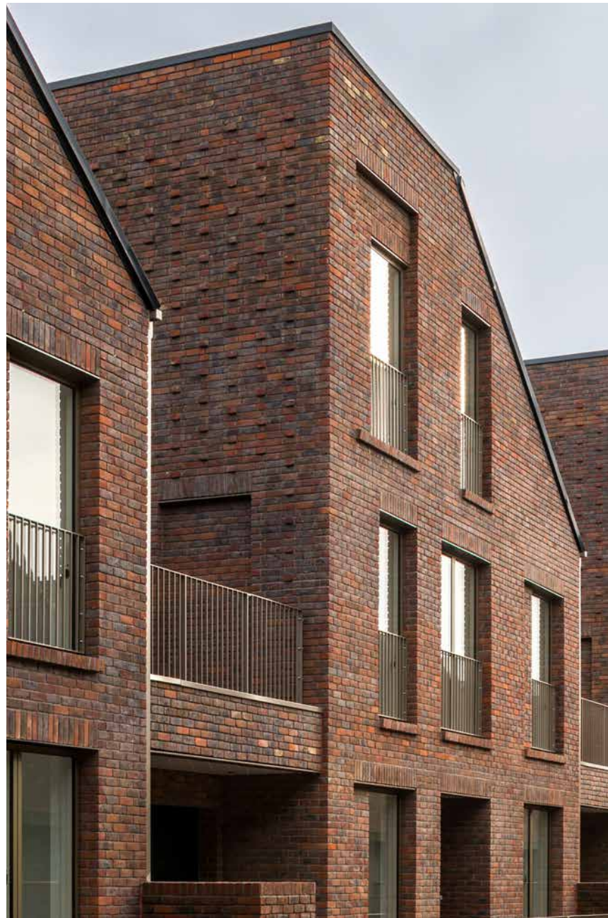
Red Brick with recessed header panels
