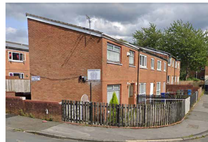
East of site - Dam Head Drive
