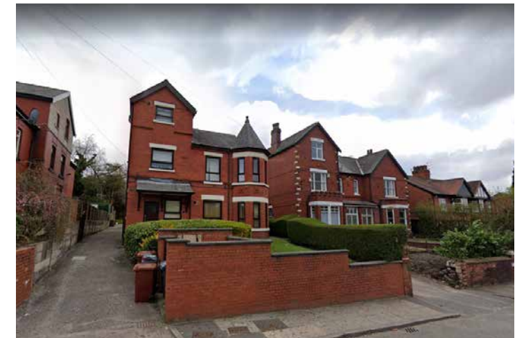
West of site - Rochdale Road
