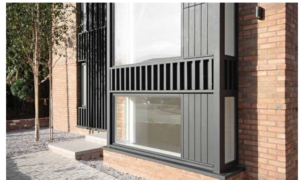
Projecting bay windows
