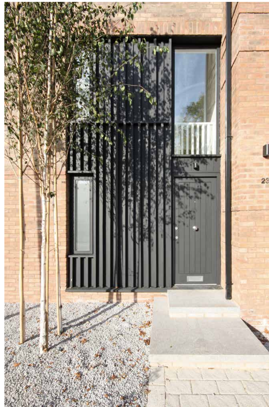
Double storey brick opening heights to front elevations
