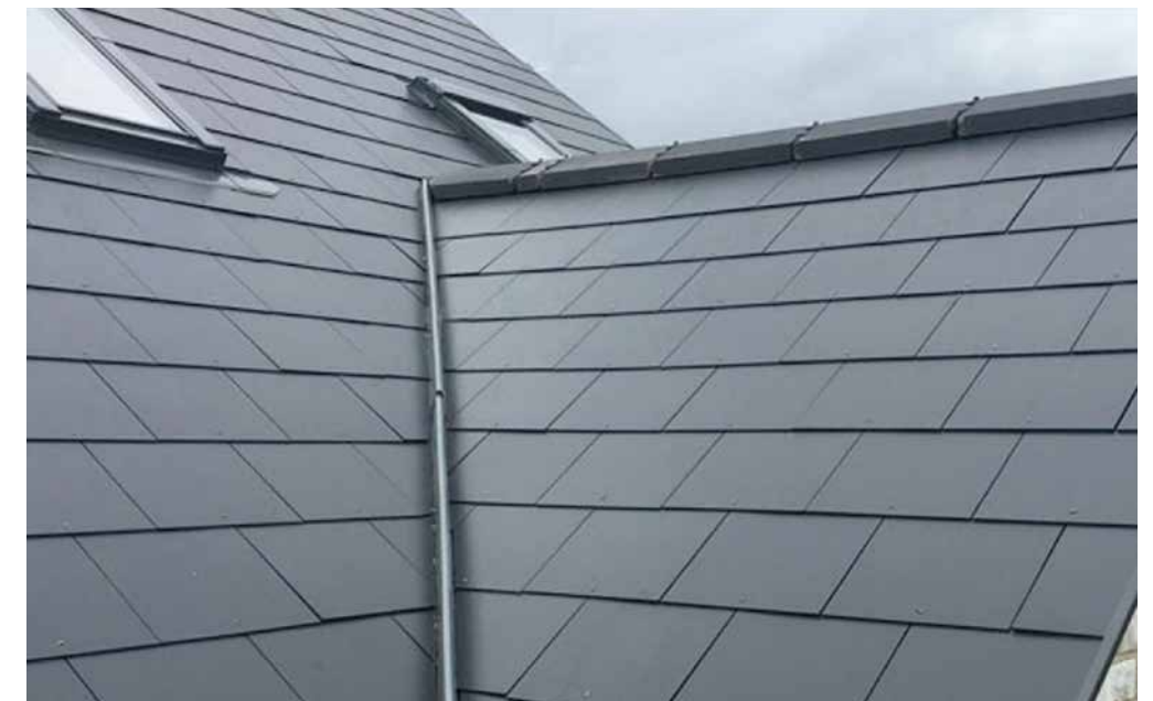
Gutters and Downpipes - half-round galvanized effect downpipes and gutters on rise and fall brackets
