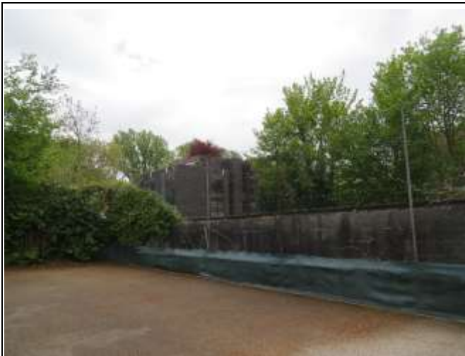
South Boundary to Parkfield Lodge Garages
