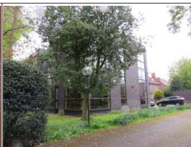
Modern Development on Elm Road
