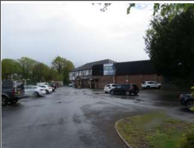
Access Road to Car Park with Squash Courts and Clubhouse to Right
