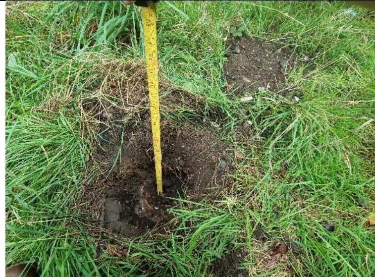
PLATE 06 – Hand Pit Excavation – HP101.
