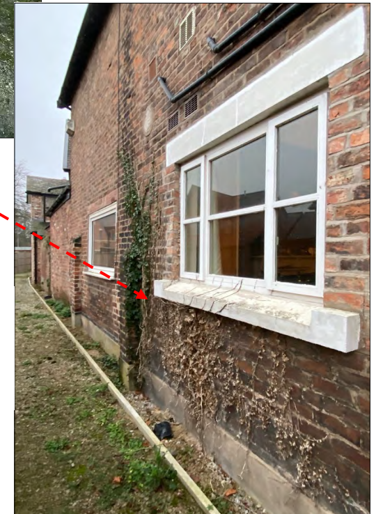
Figure E: Western aspect of 11 The Grove showing approximate location of maintenance strip gate
