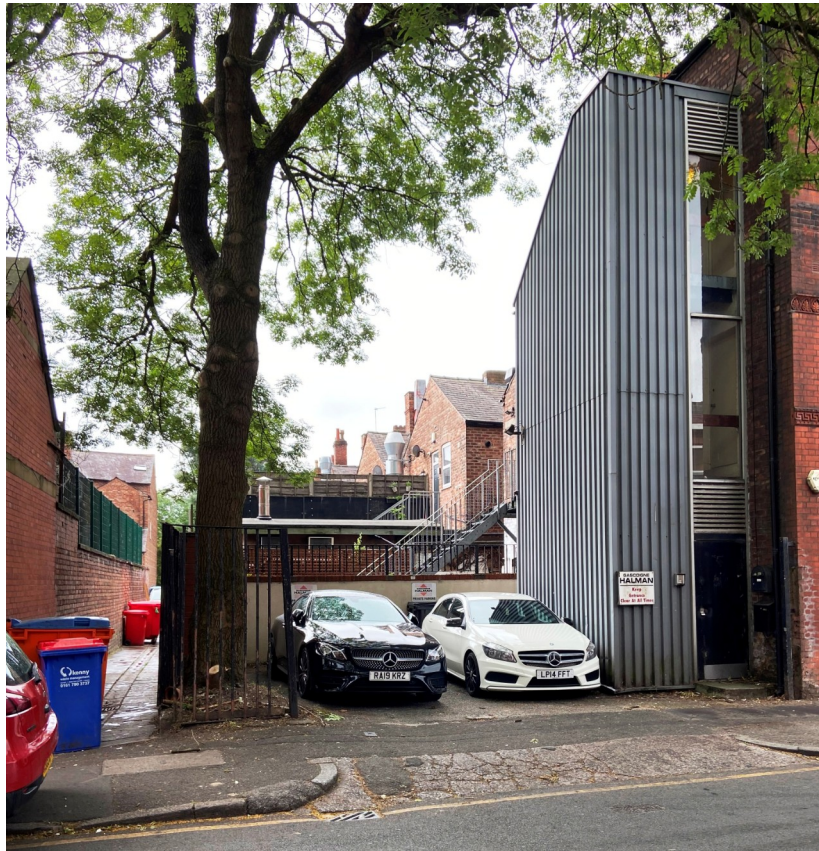
View of the rear of properties on Wilmslow Road from Elm Grove
