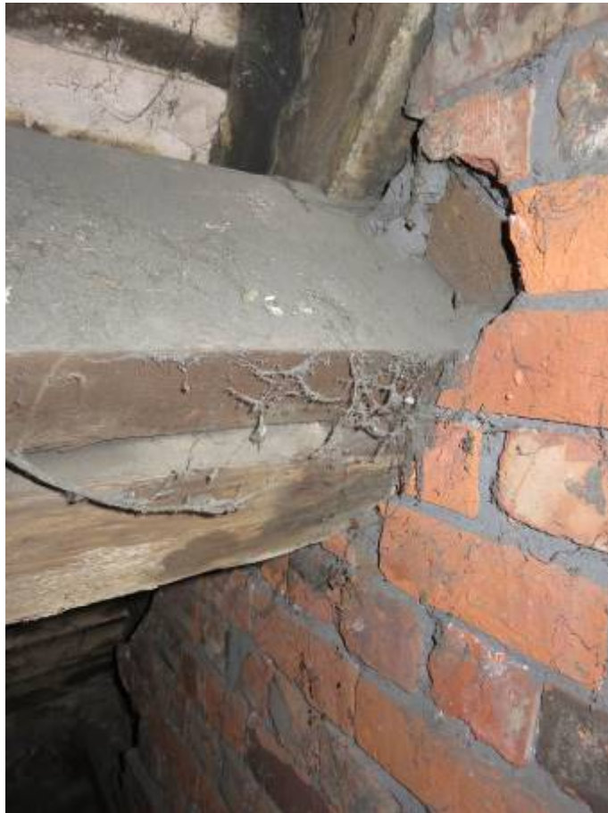
Photograph 10: Purlin to south gable to east side with repair timber
