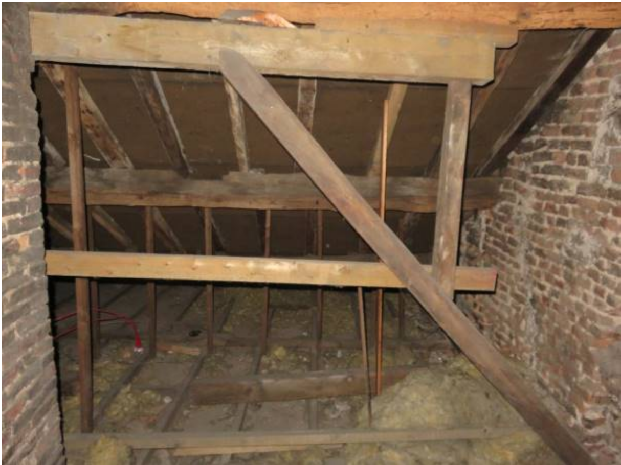
Photograph 50: Strut to purlin to east side at southern end of northern roof structure
