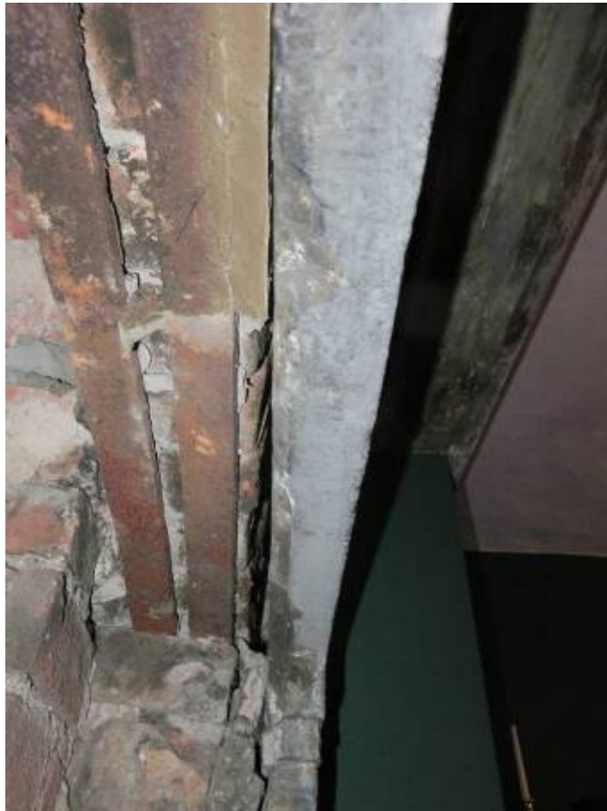
Photograph 57: Thin stone veneer to front of fireplace
