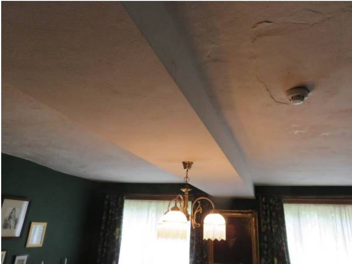
Photograph 55: Wide downstand beam in Dining Room
