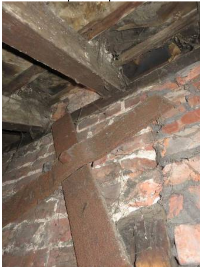
Photograph 27: Cross pattress plate to south end at eaves as seen from western corridor attic
