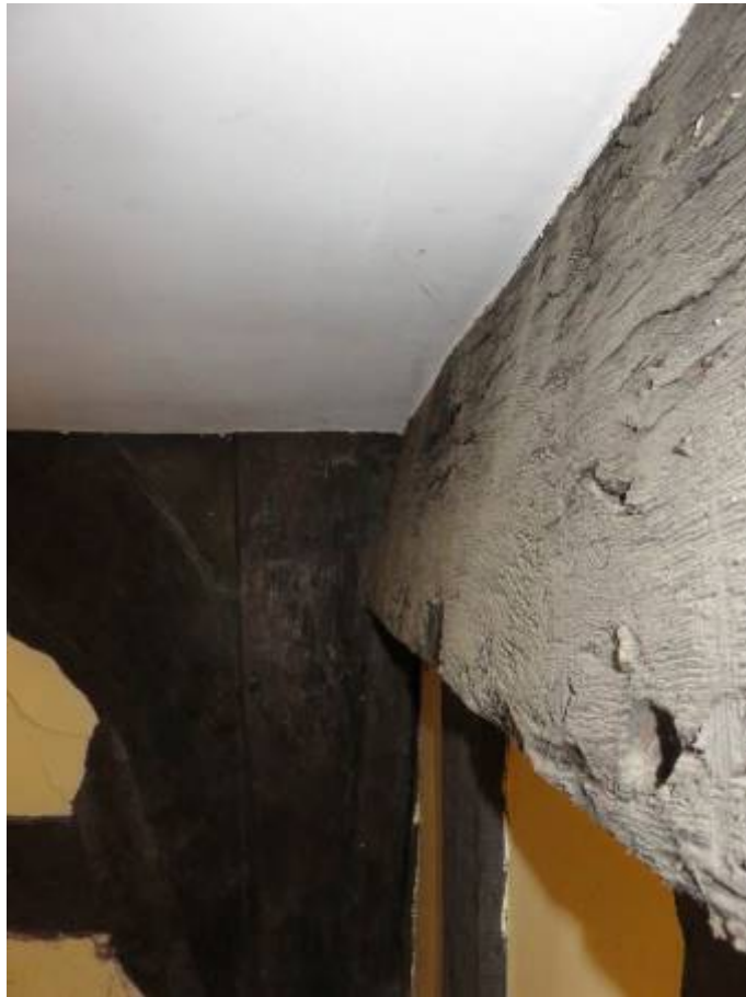
Photograph 14: Rotated eaves plate with finishes unaffected
