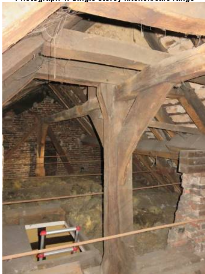
Photograph 5: Central crown post between north and south bay
