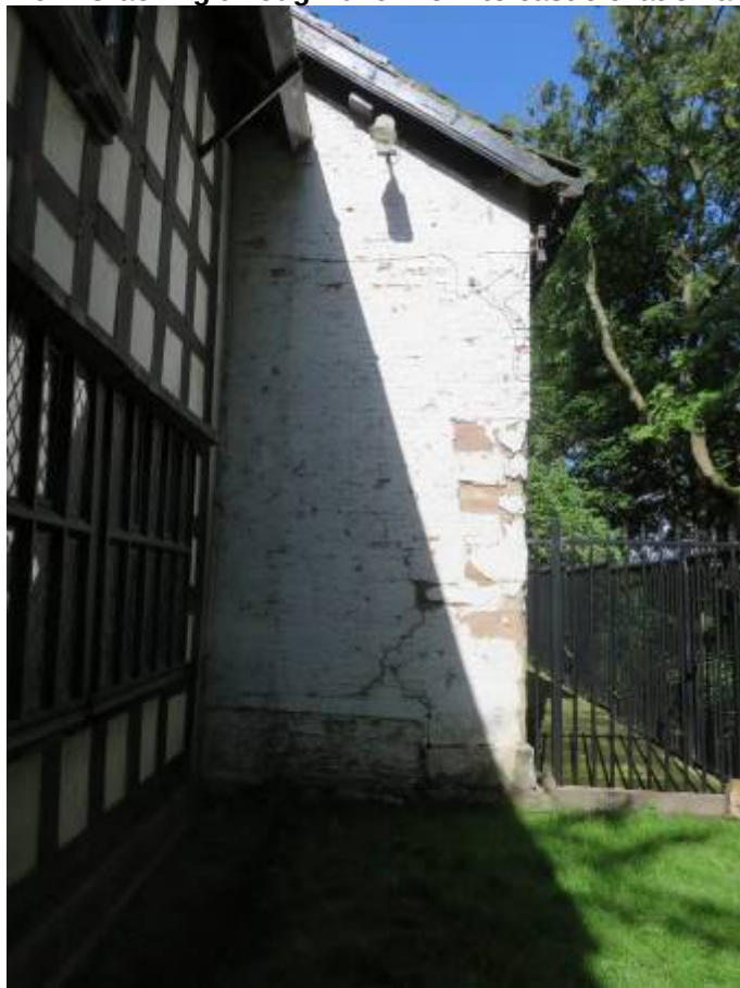
Photograph 47: South section of gable to northern range
