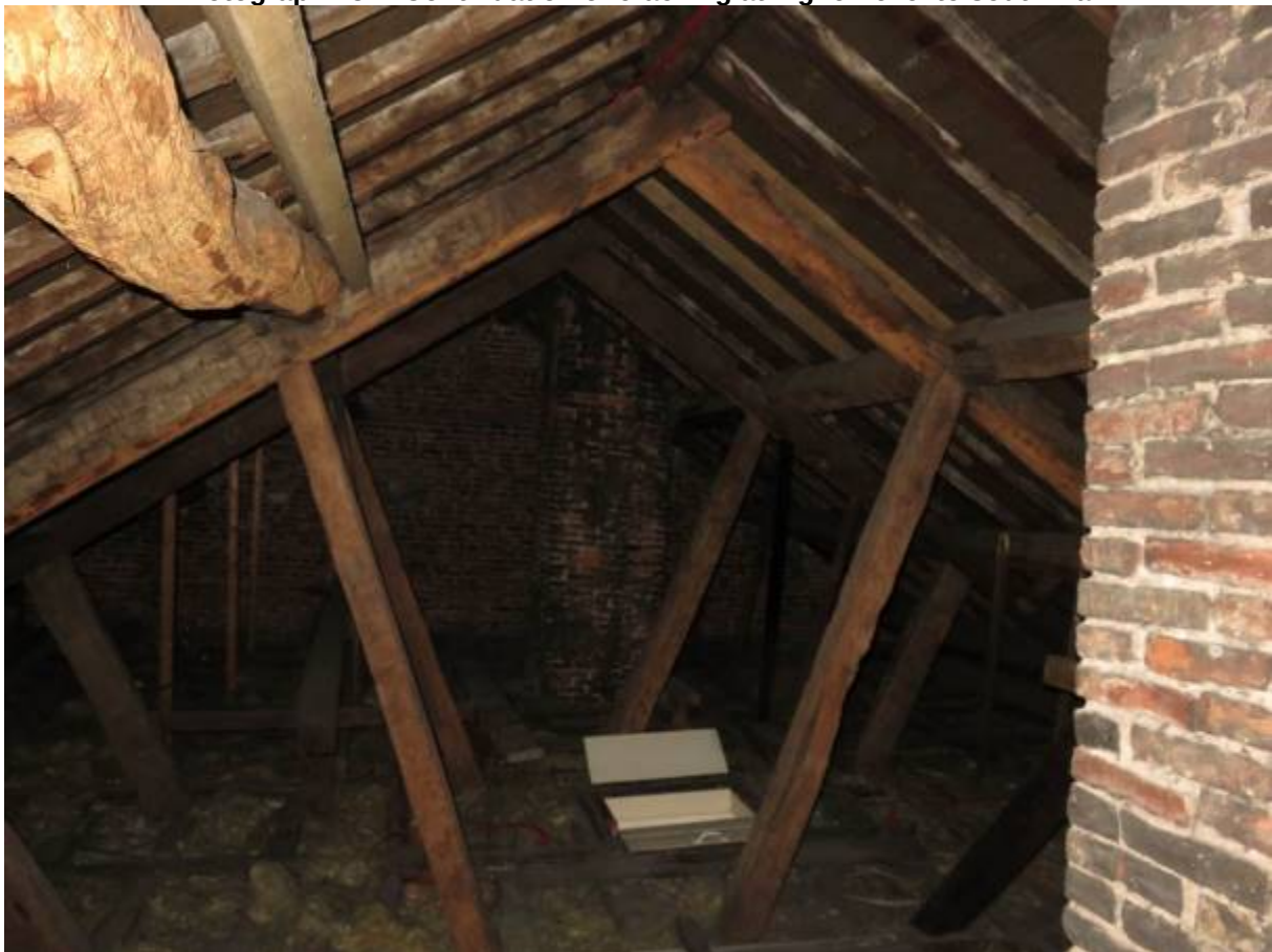
Photograph 49: Roof structure to northern range
