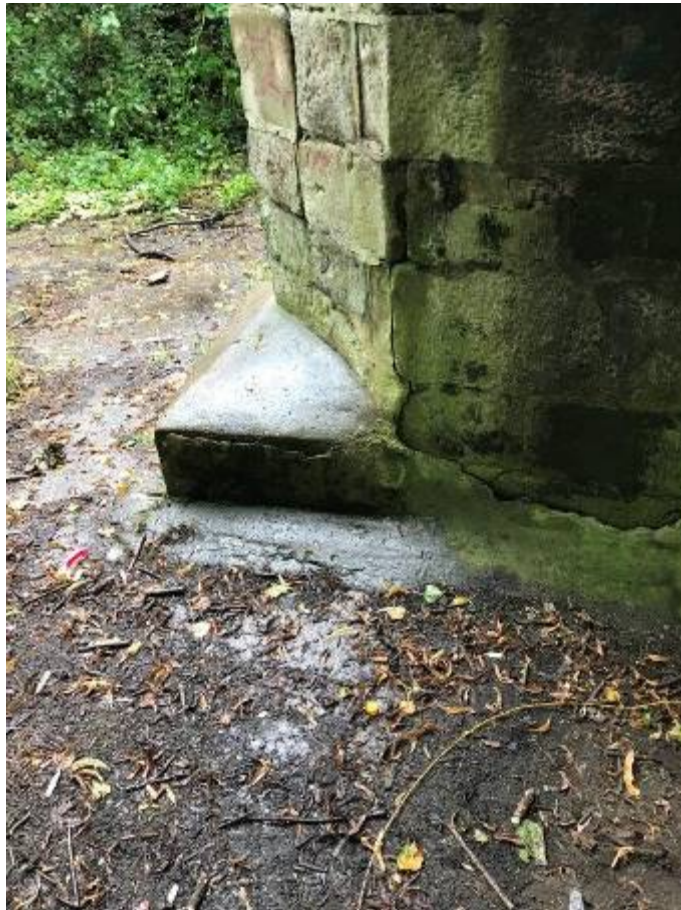
Photograph 70L: Cement Skirt to base of pier and projection of cut water to east
