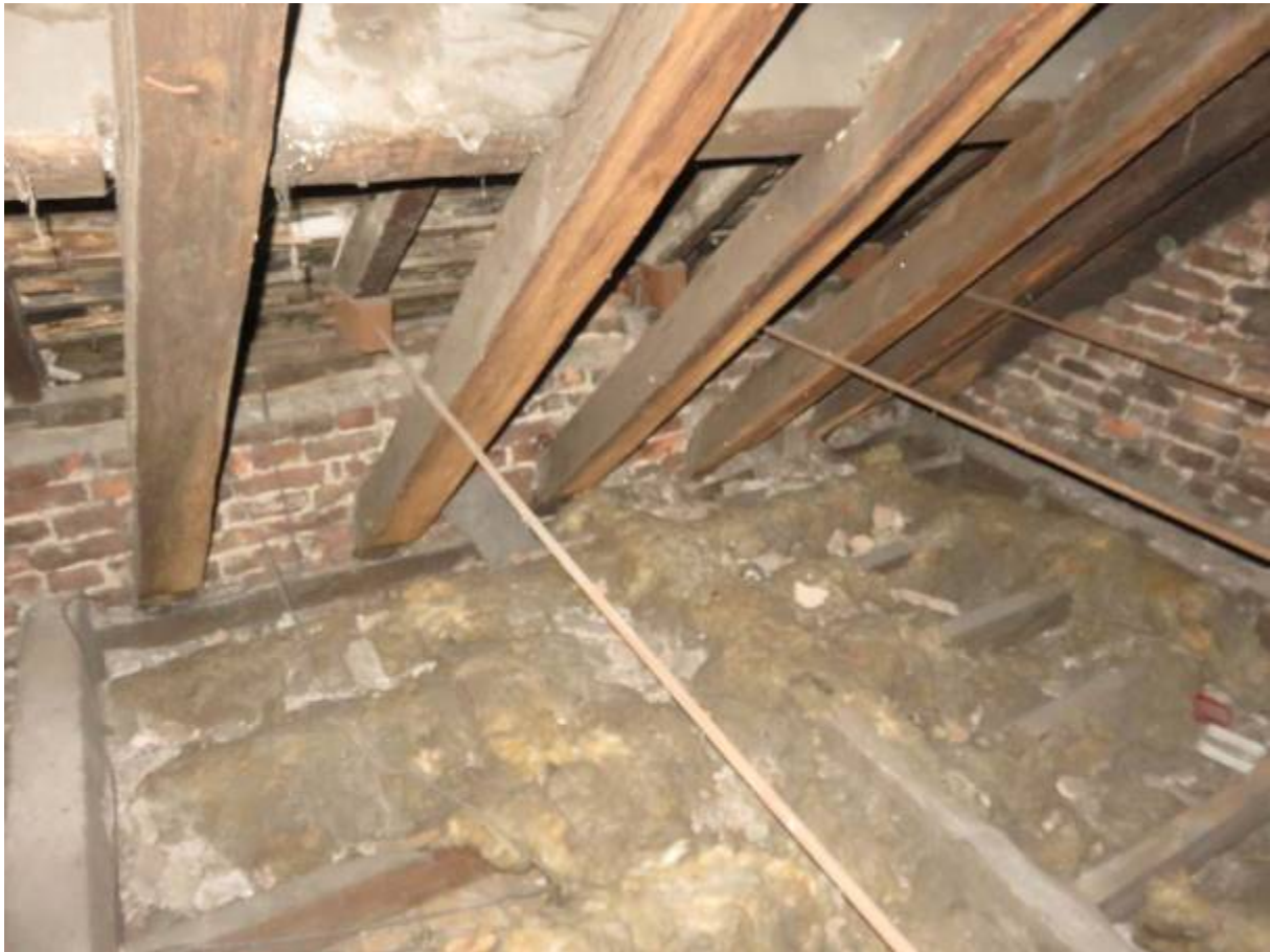
Photograph 8: Eaves to west side raised with added brickwork and further rafters
