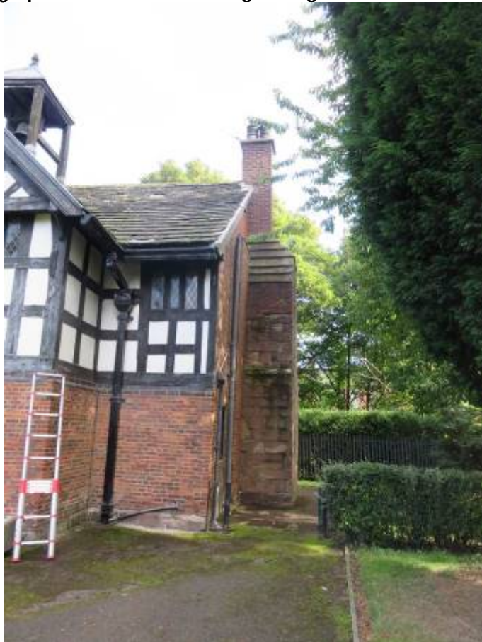
Photograph 41: South end of west elevation
