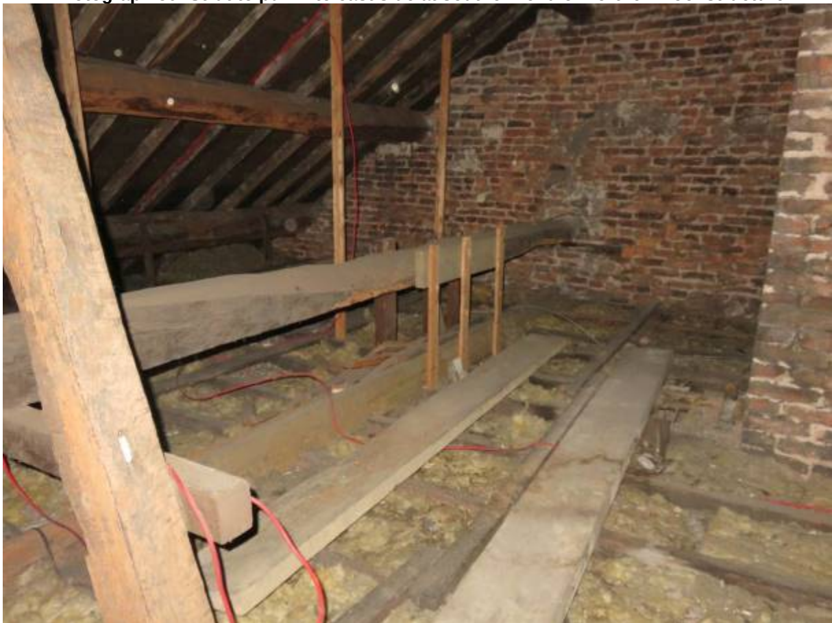
Photograph 51: Hangers to ceiling
