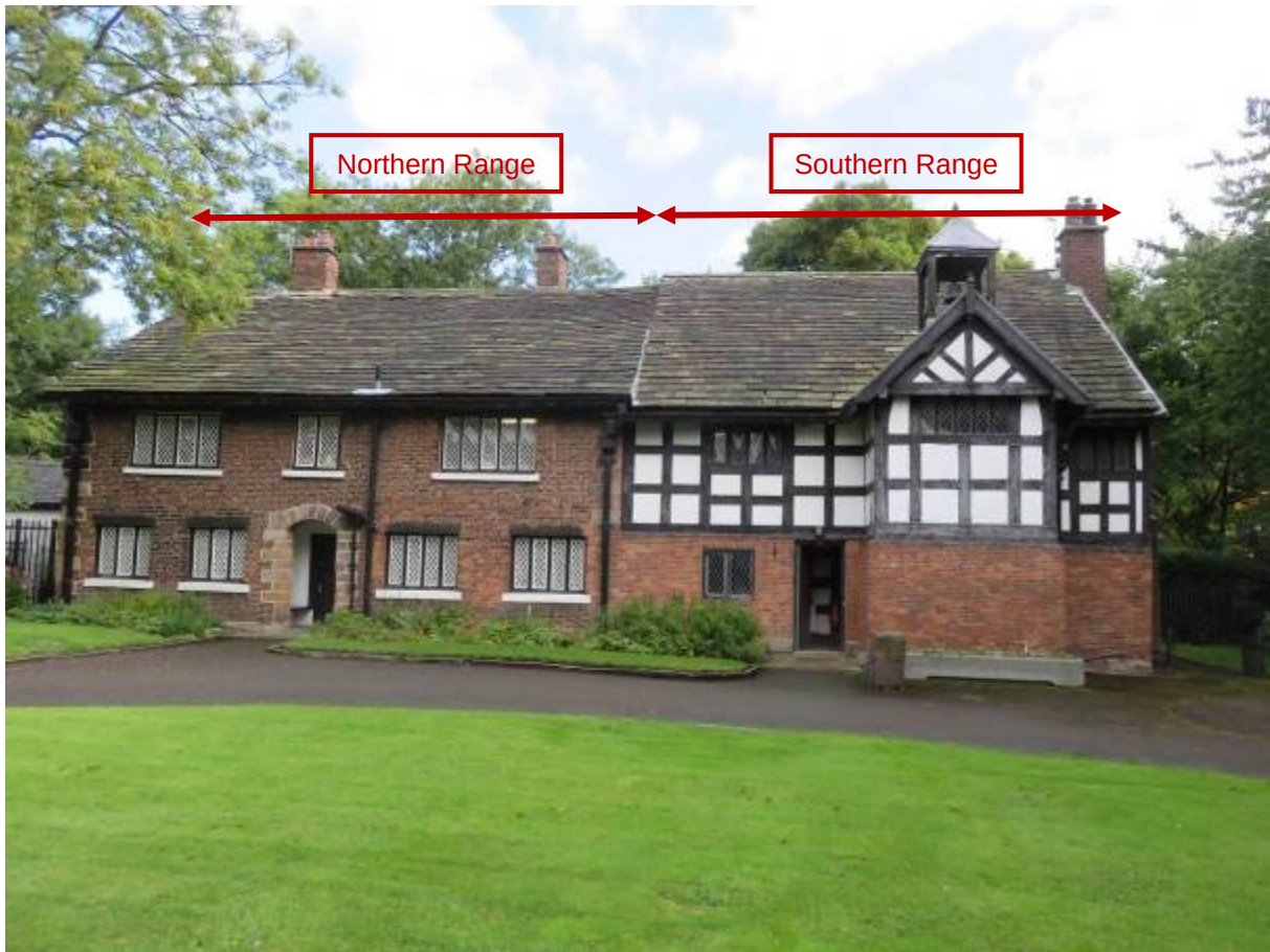
Photograph 1: Clayton Hall West Elevation
