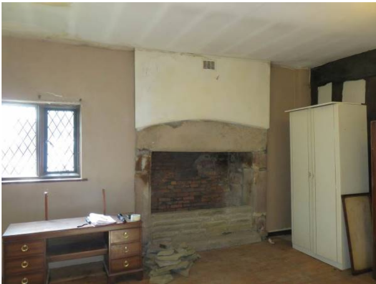
Photograph 23: First floor inglenook to south gable wall
