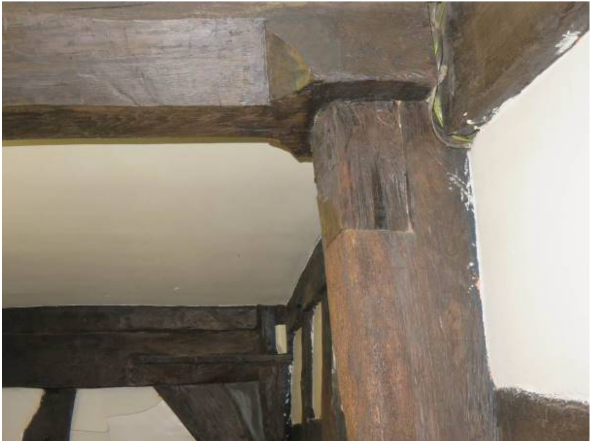
Photograph 29: Timber blocking piece to cross beam
