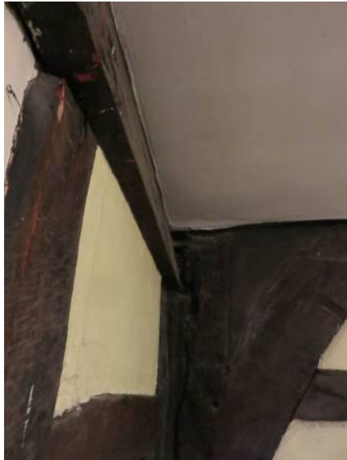
Photograph 19: Rotation of western eaves plate to north bay
