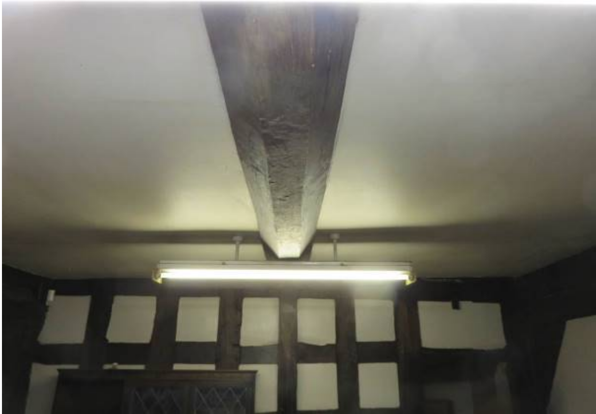
Photograph 20: Chamfered spine beam to north bay as seen from underside
