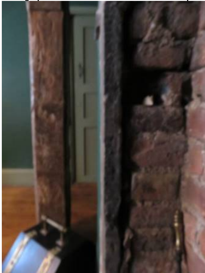
Photograph 58: Stone veneer to fireplace surround
