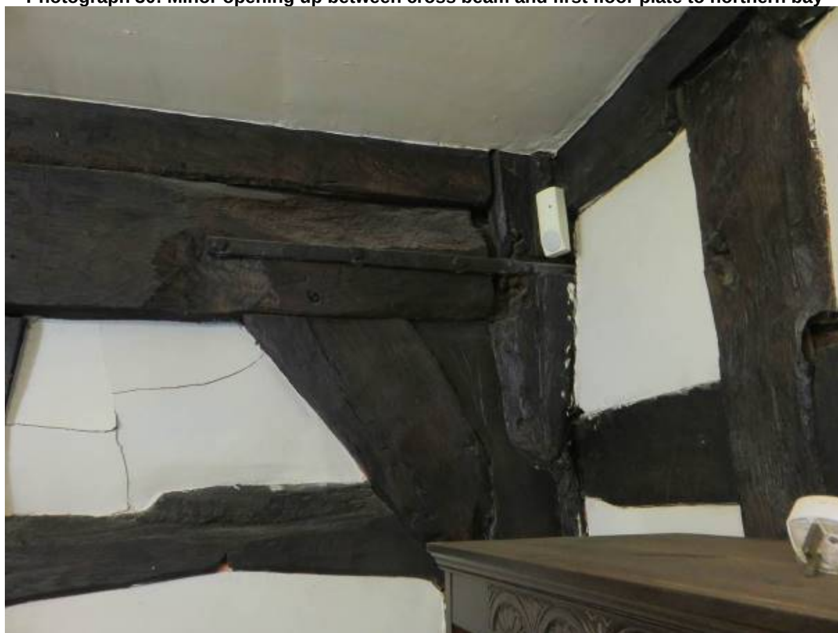
Photograph 31: Main beam on frame to west end between bays
