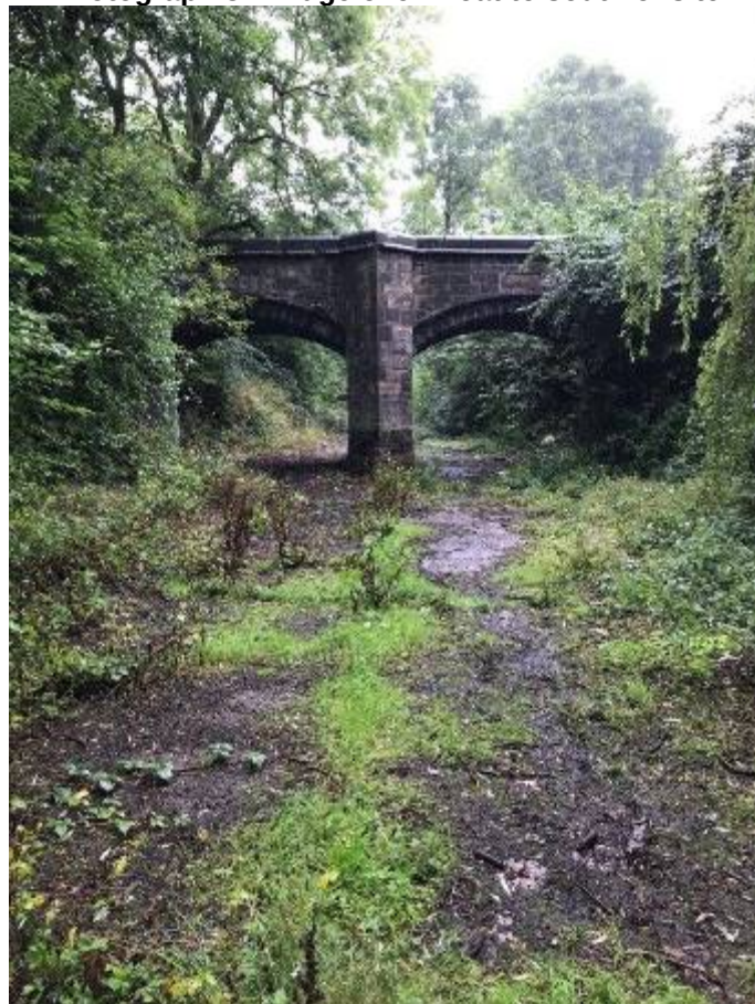
Photograph 3A: Double arch masonry bridge across former moat
