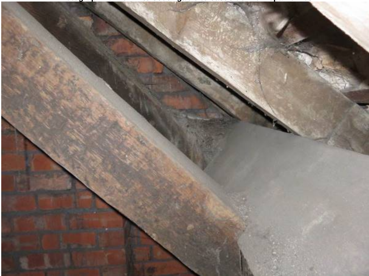
Photograph 11: Added plate supporting upper later rafter from western corridor
