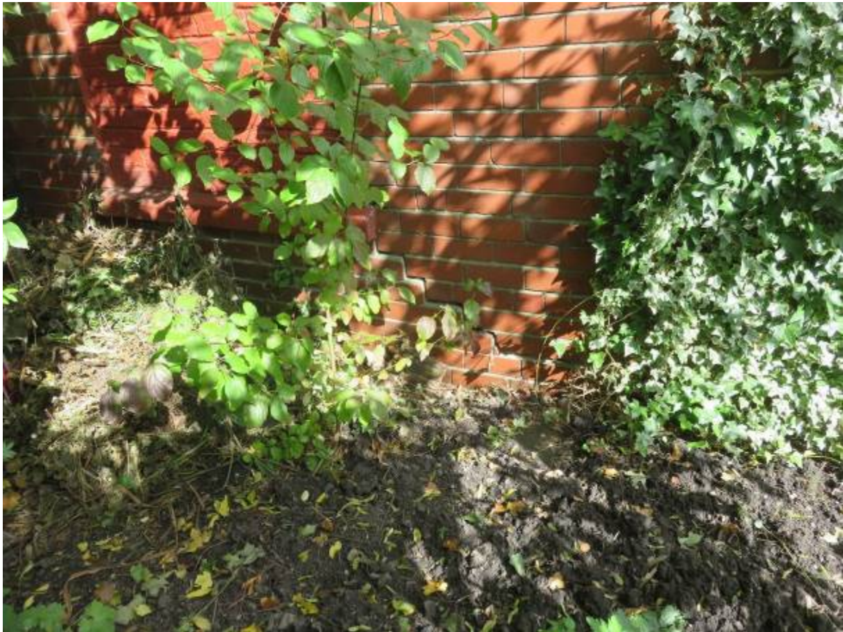
Photograph 68: Cracking to low level to west elevation
