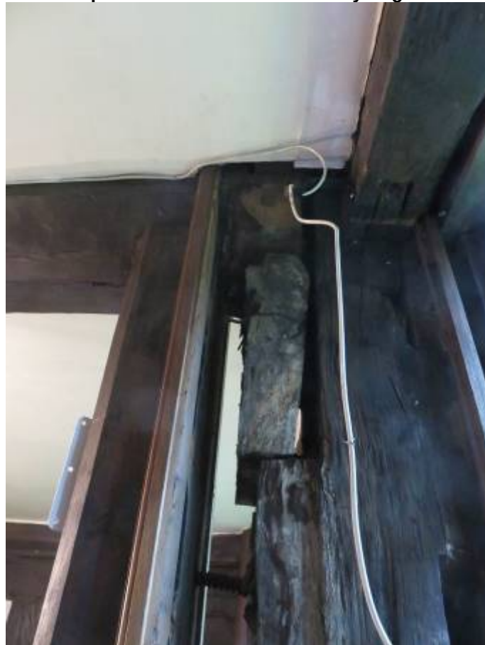
Photograph 33: Added post to centre of southern bay to ground floor to east side
