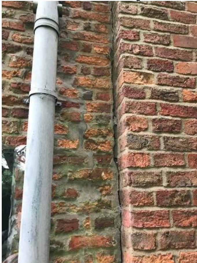
Photograph 42B: Opening up between stack projection and west wall hinging at base point
