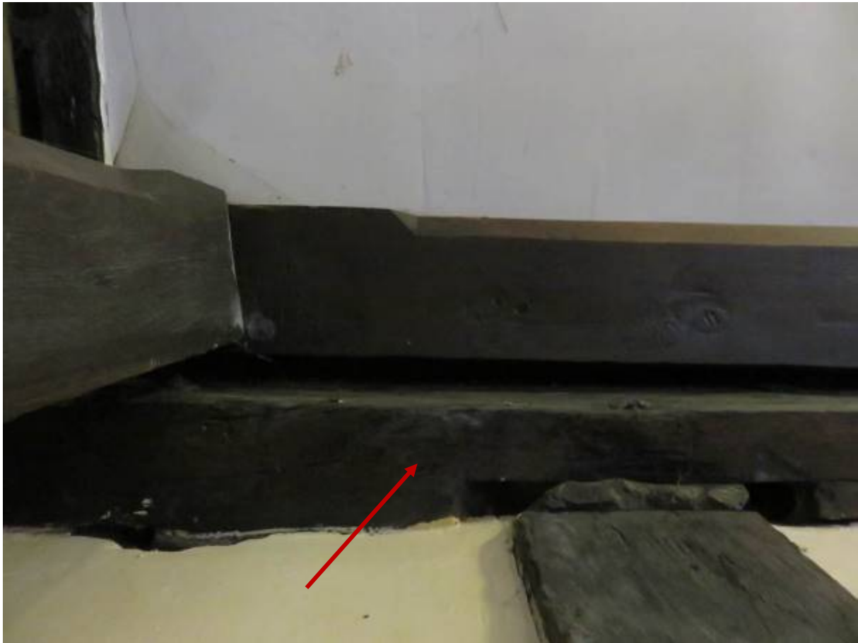
Photograph 22: Original eaves plate rotated (highlighted) and new plate alongside
