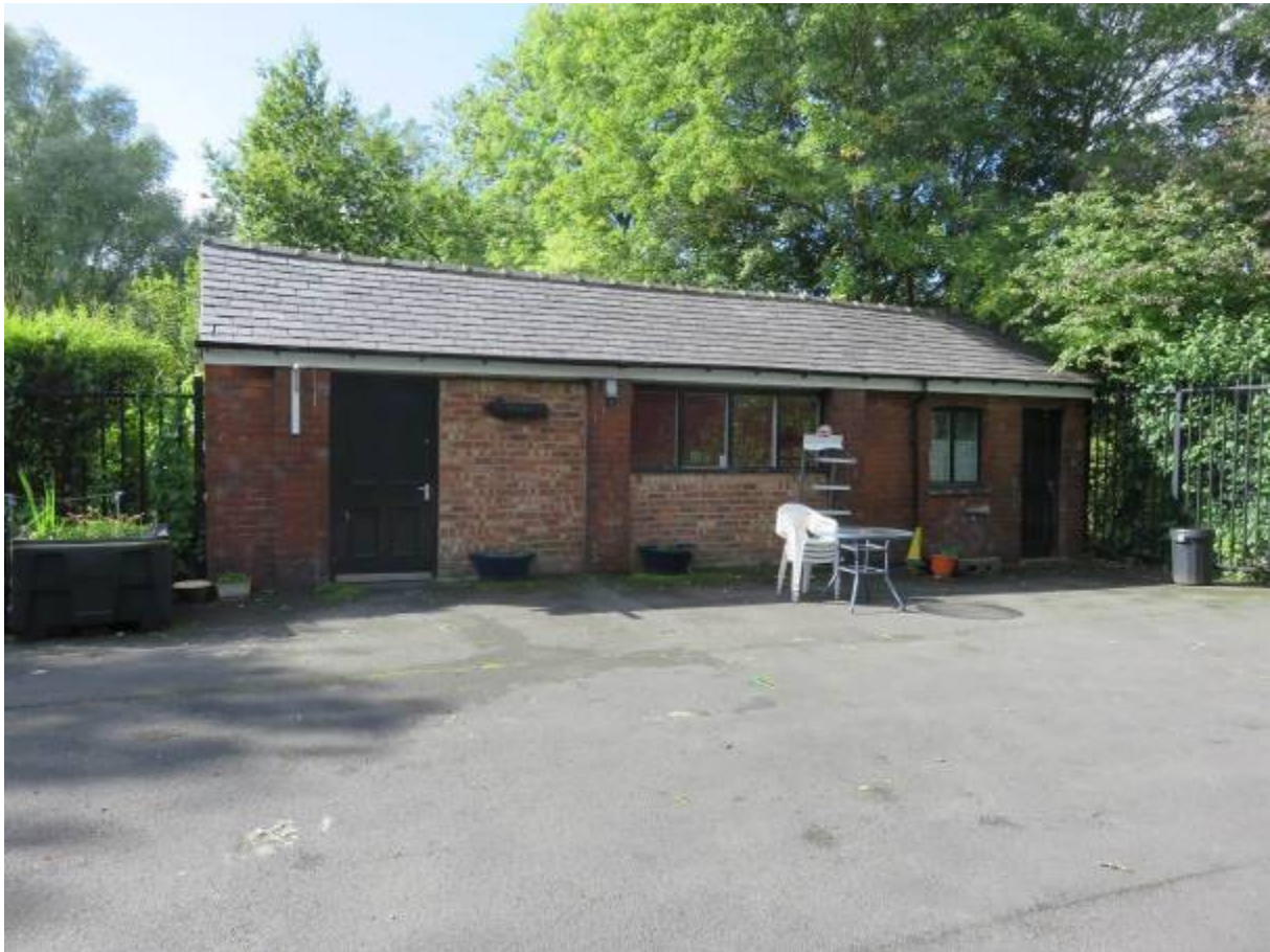
Photograph 4: Single storey kitchen/café range
