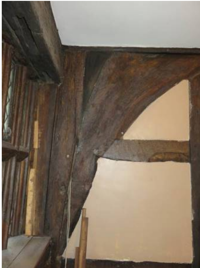
Photograph 17: Junction of east bay at central frame position and cross partition
