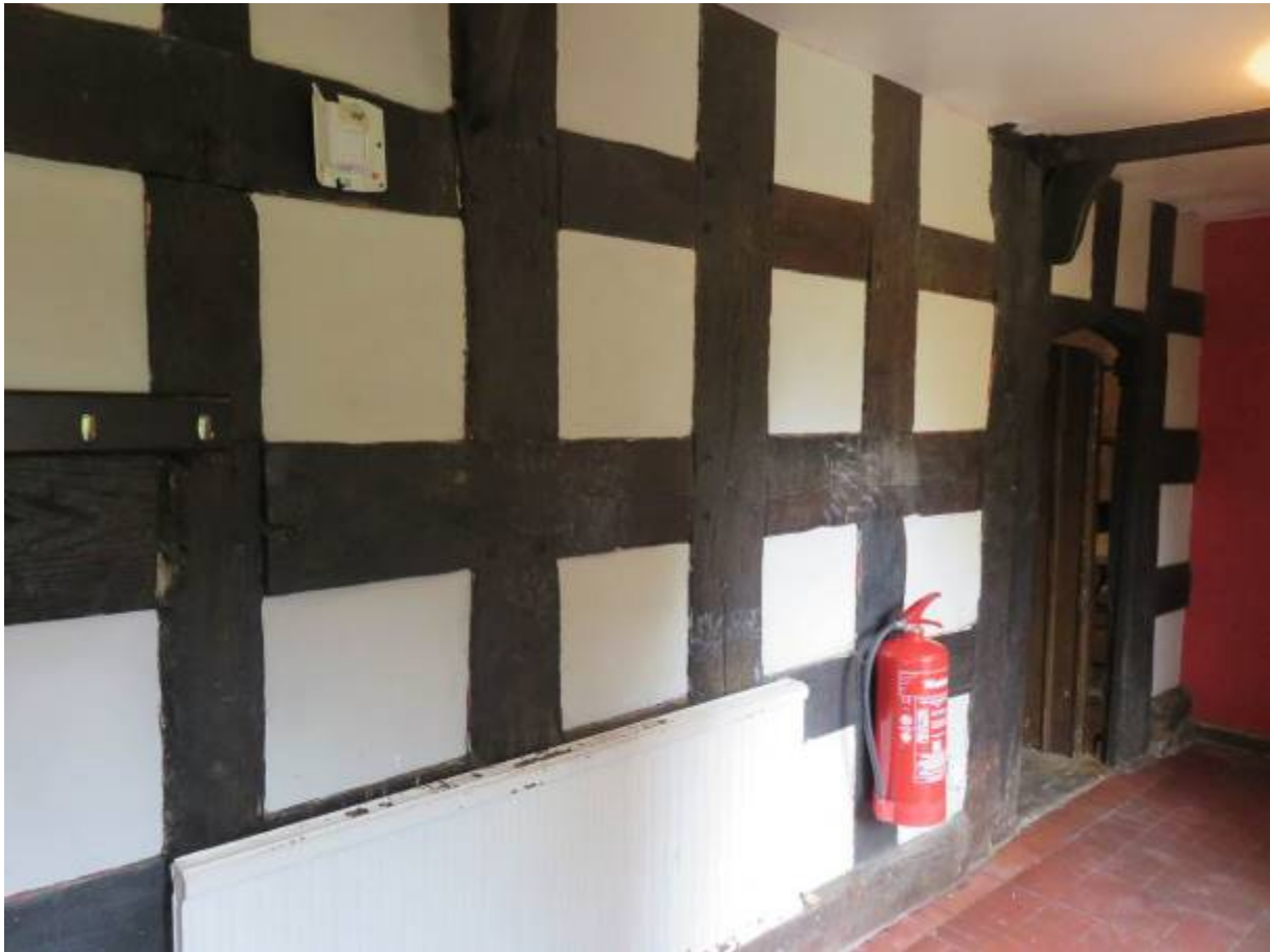
Photograph 34: West wall of south bay
