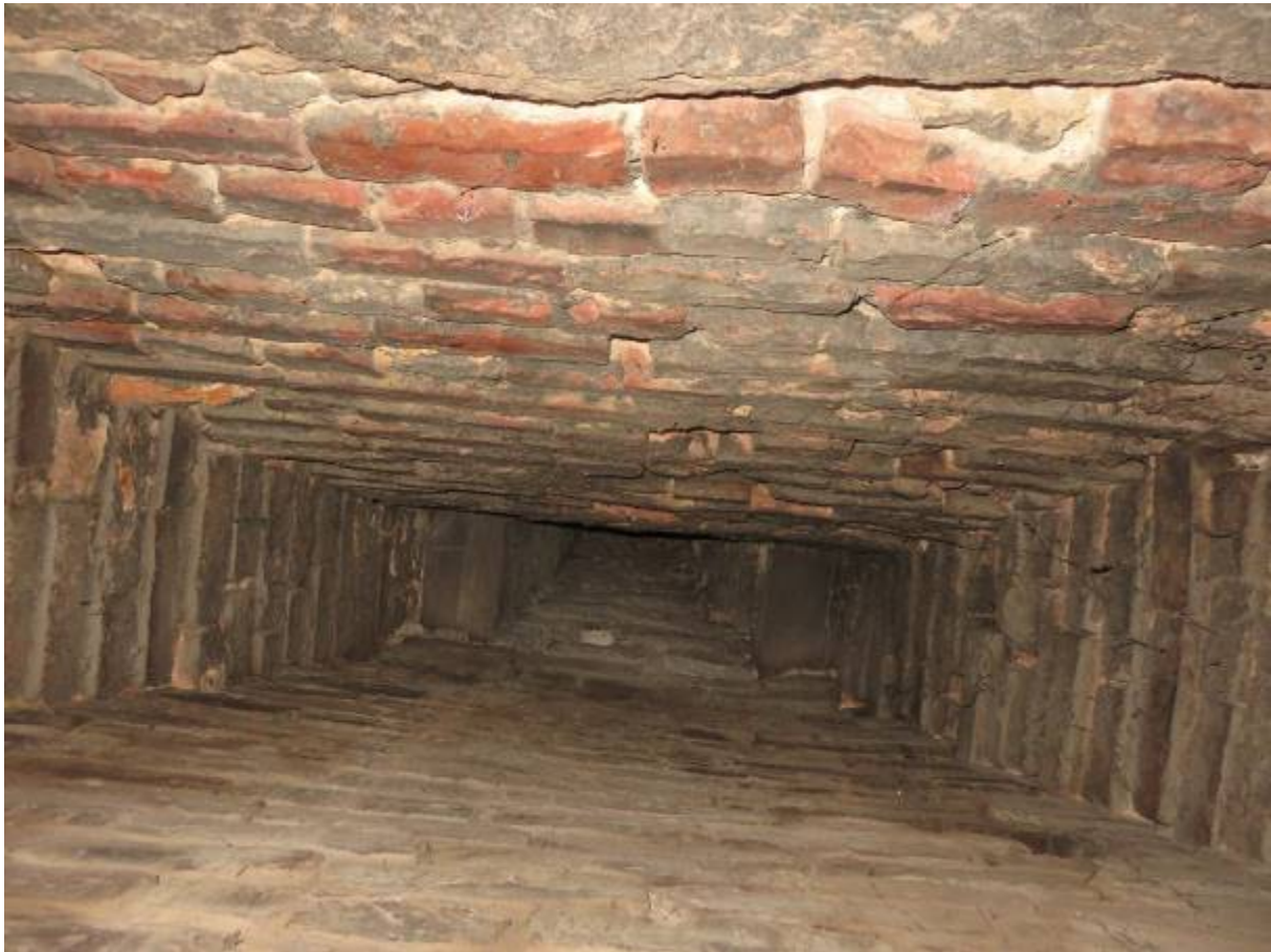
Photograph 24: View up inglenook fireplace to south gable at first floor
