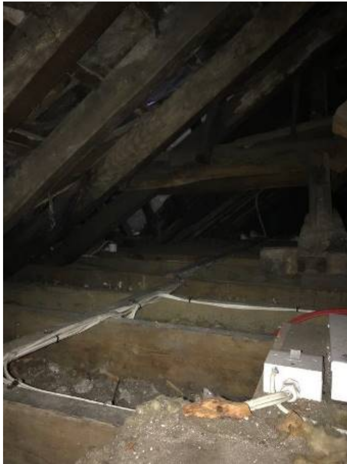
Photograph 28A: General view of roof space in satisfactory condition
