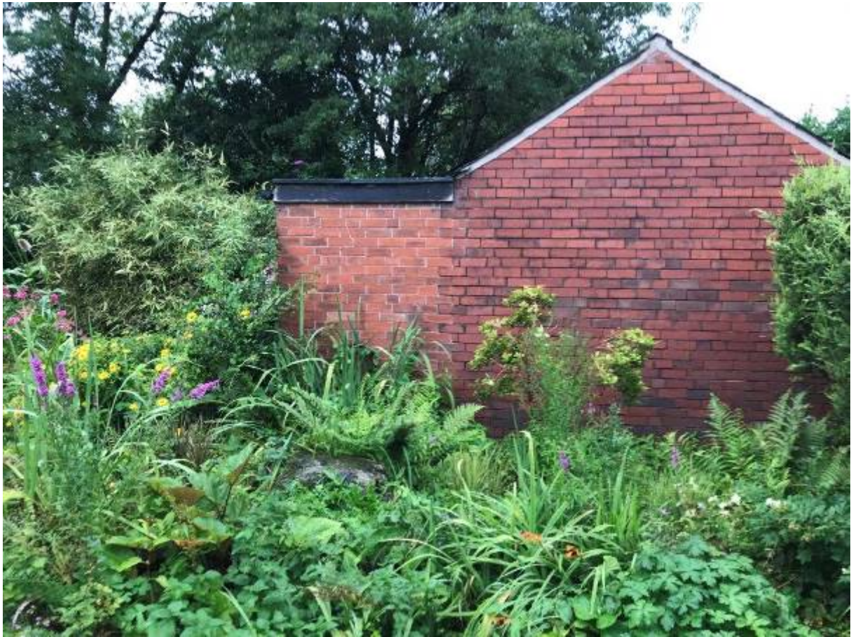
Photograph 65A: General arrangement of outbuilding to its south elevation
