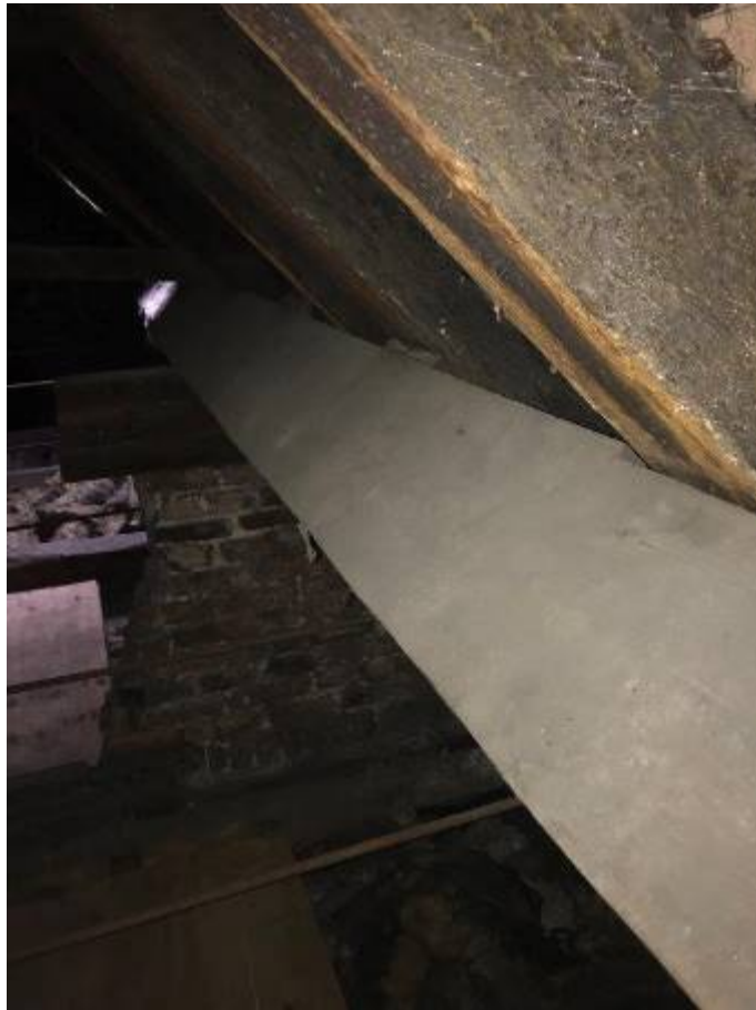
Photograph 12A: Notched and packed purlin to common rafter interface
