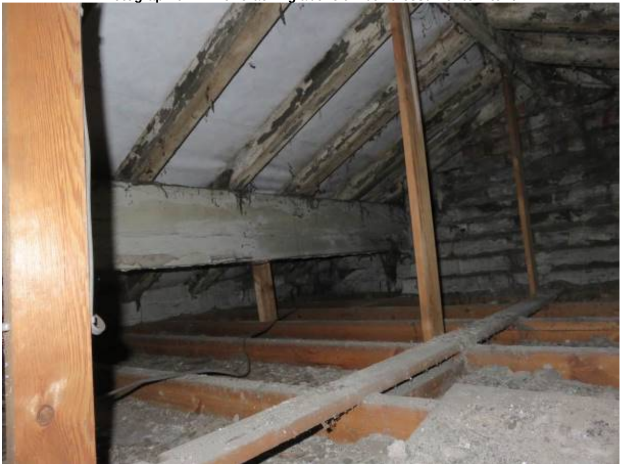
Photograph 63: Roof structure over Wash House
