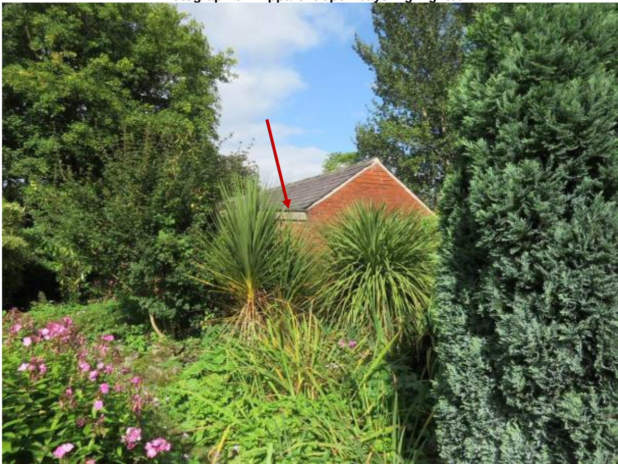
Photograph 65: West elevation of café and kitchen with part flat roof highlighted
