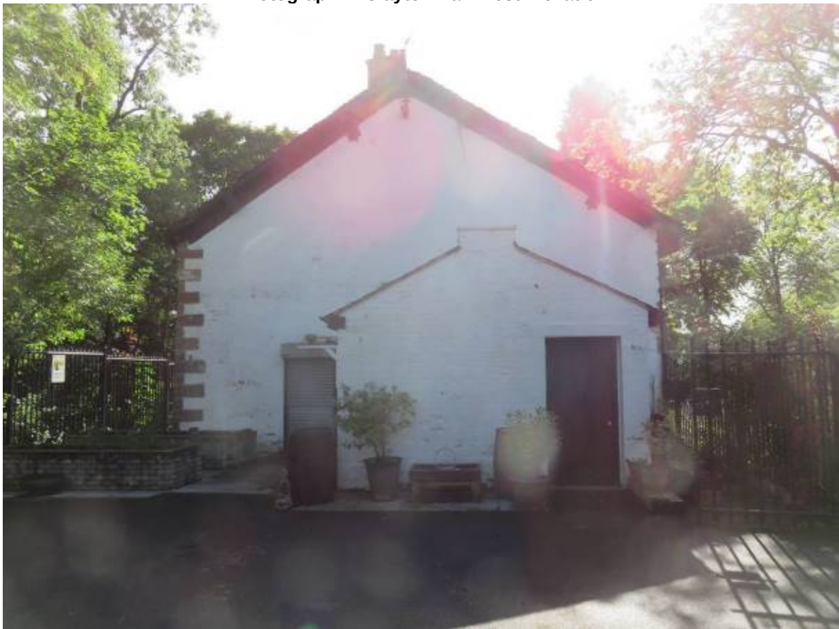
Photograph 2: Single storey service building to north of northern range
