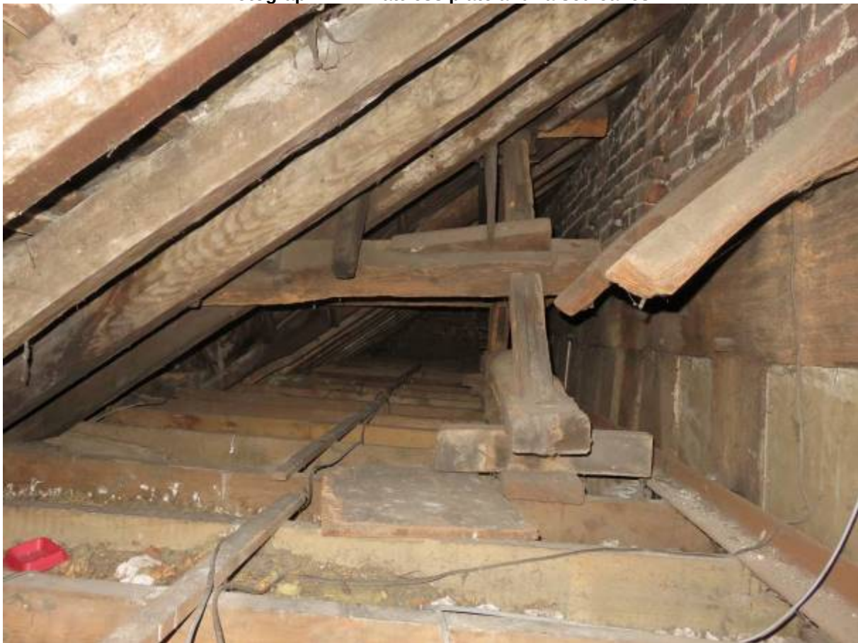
Photograph 28: View along western corridor roof looking north
