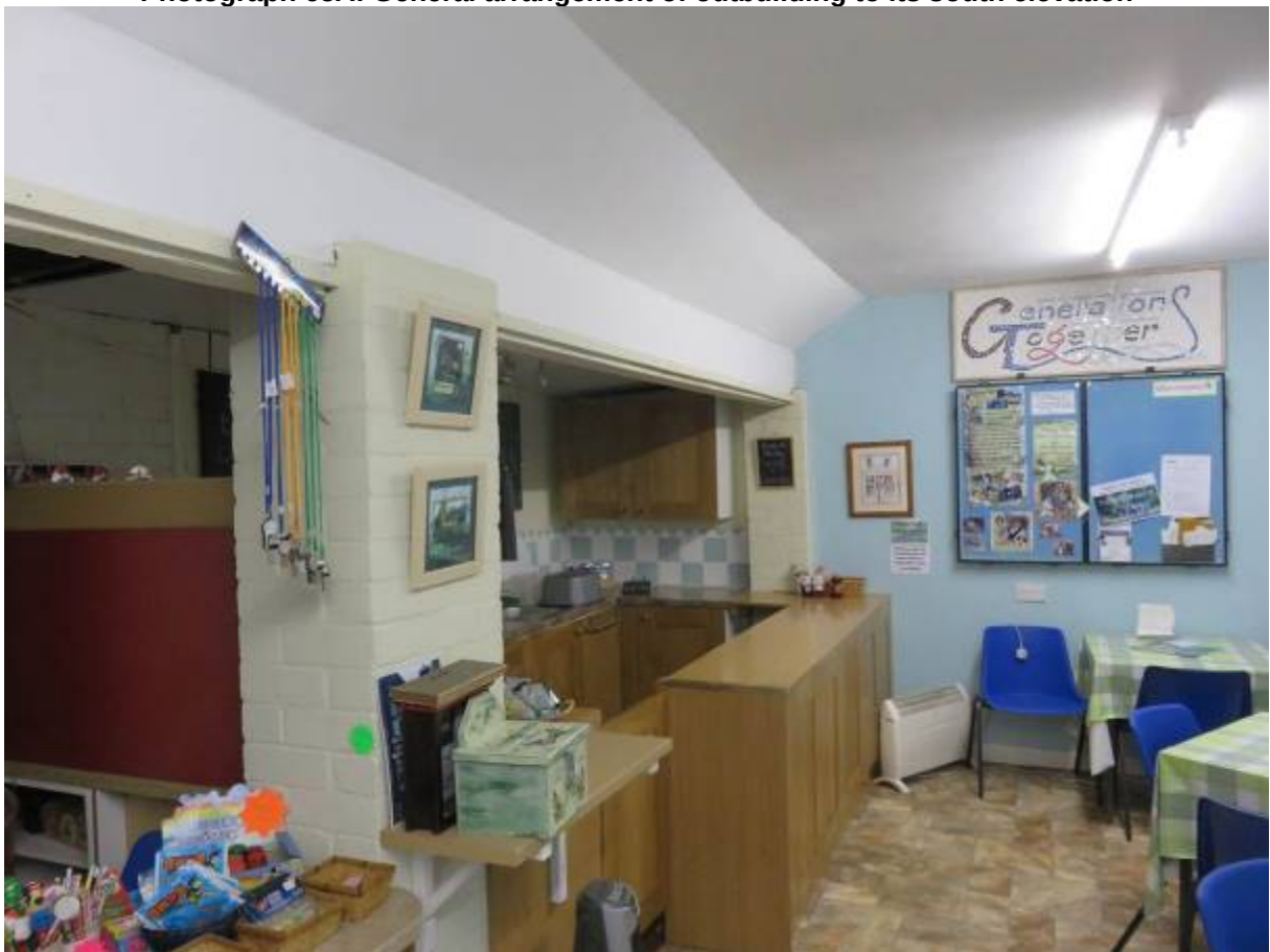
Photograph 66: Opening to rear west wall with piers supporting beams and then roof
