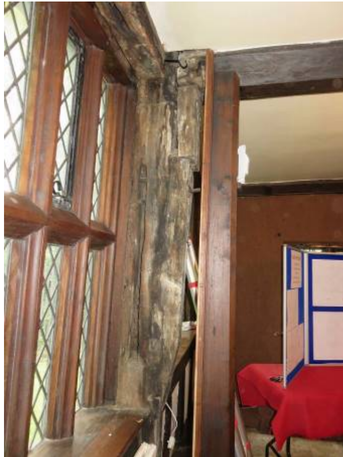
Photograph 32: Added post to centre of southern bay to ground floor to east side
