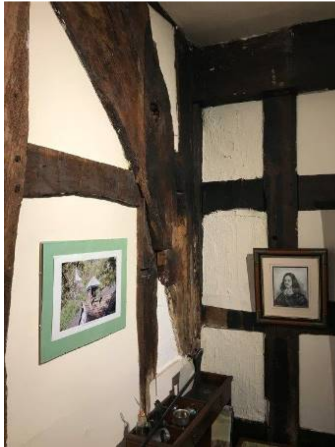
Photograph 18A: Repairs undertaken to finishes and infill panels. West wall still has minor movement
