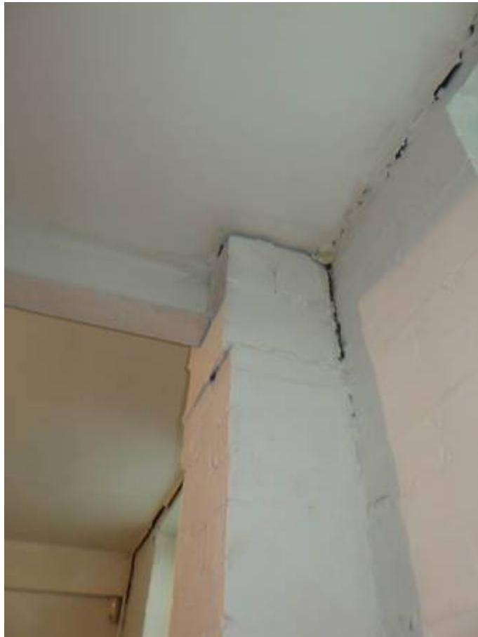
Photograph 59: Movement of added brick pier to west side of larder and steel beam
