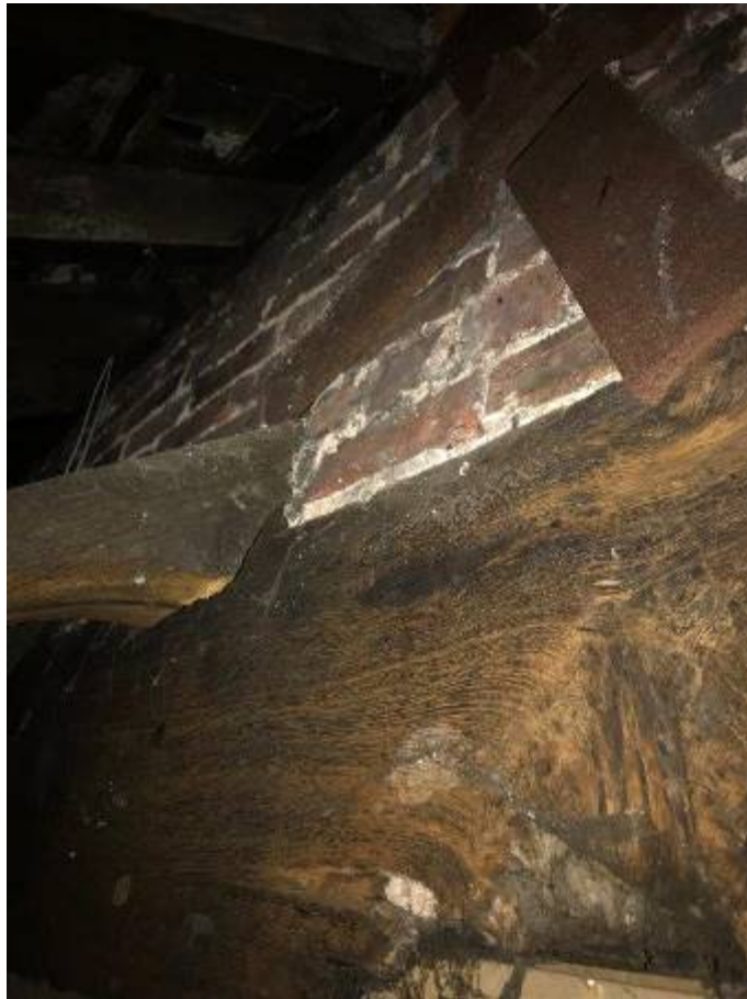
Photograph 27A: Patten plate and raised eaves
