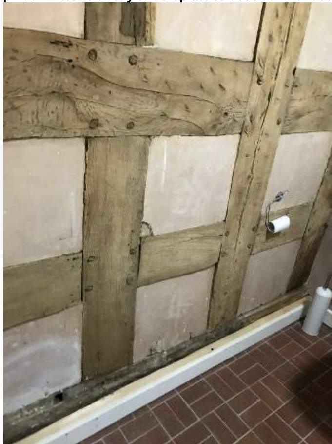
Photograph 36A: Spliced end to soleplate cleaned timberwork
