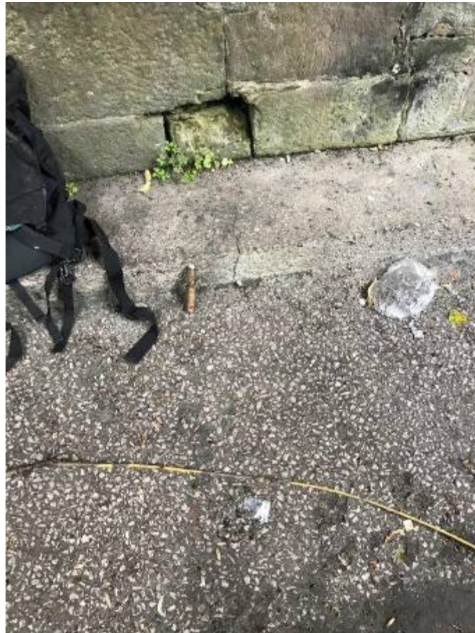
Photograph 70H: Concrete upstand to moat at north abutment
