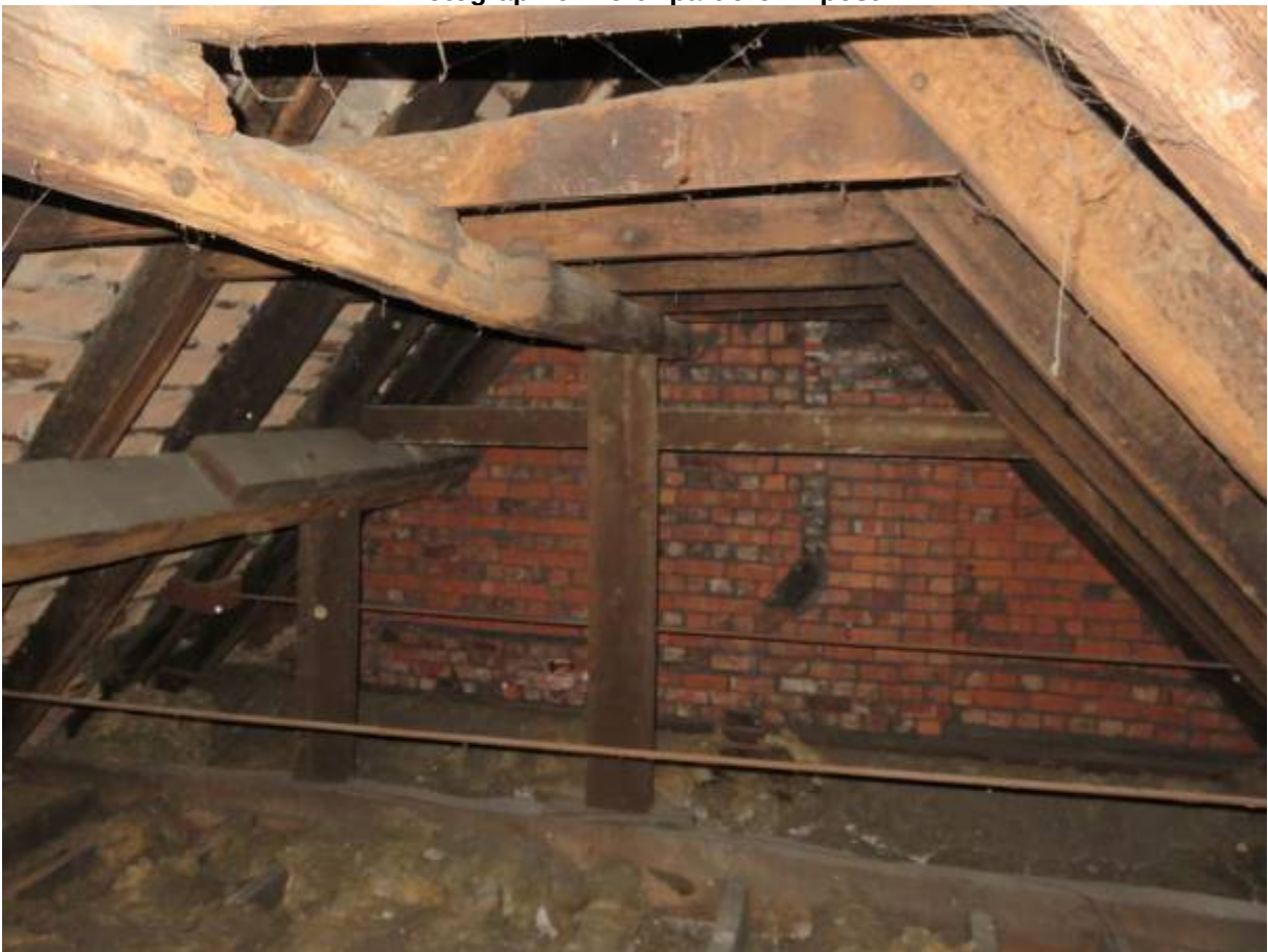
Photograph 7: South end of roof with brick gable
