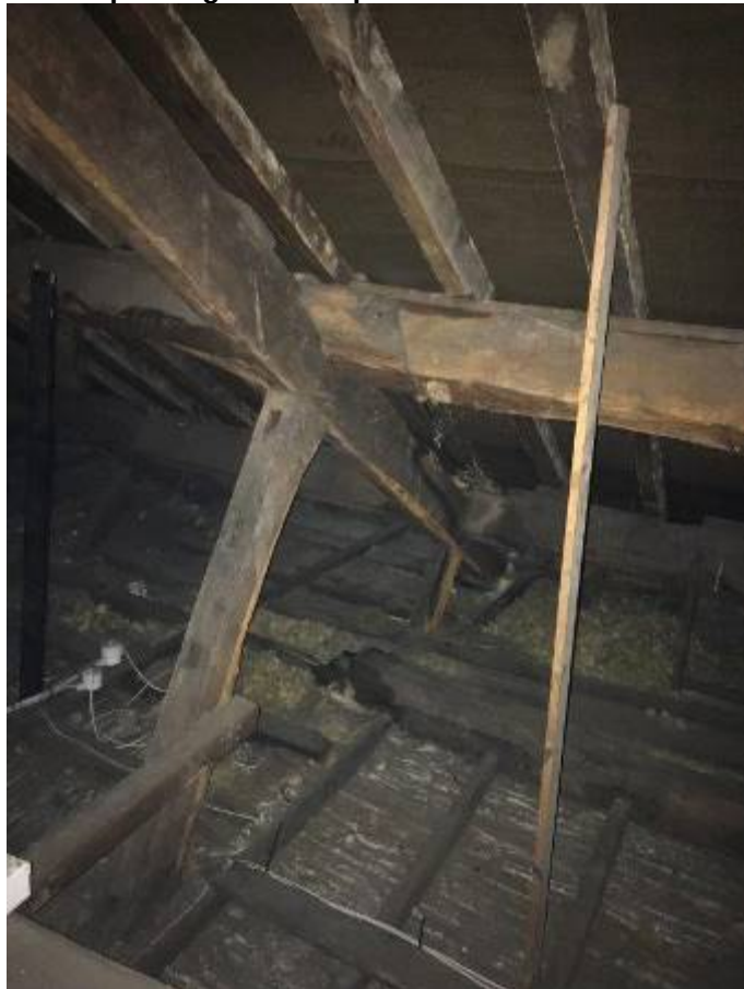
Photograph 49B: Packing timbers upon purlin to level roof in previous re-roofing works
