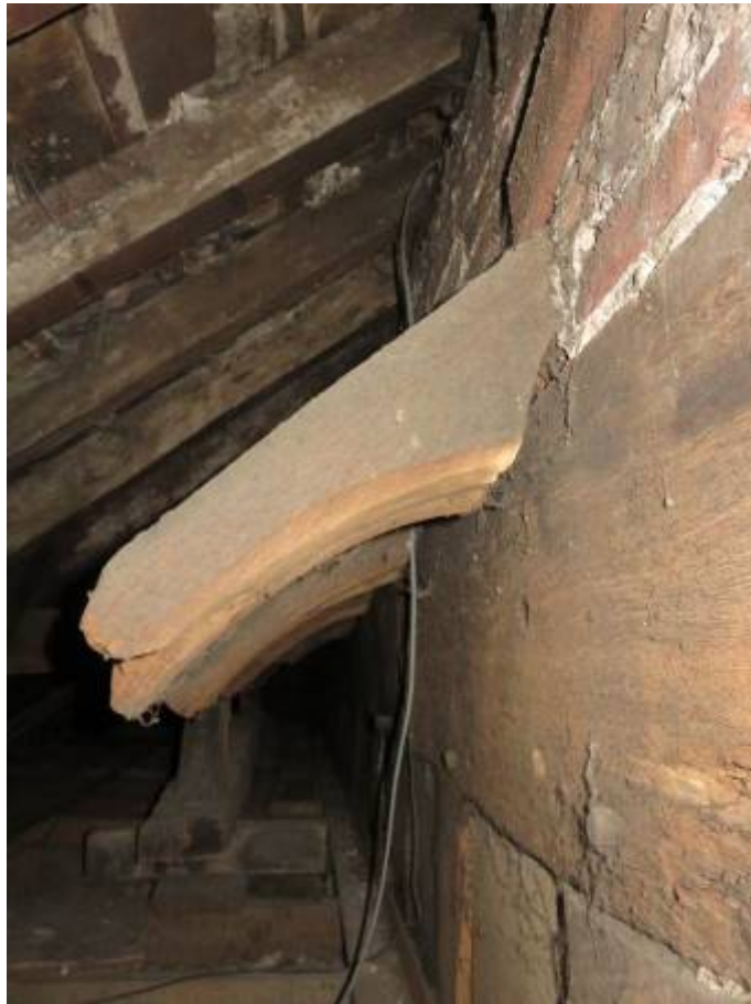
Photograph 26: West elevation eaves plate and sprockets to rafters seen in west corridor attic
