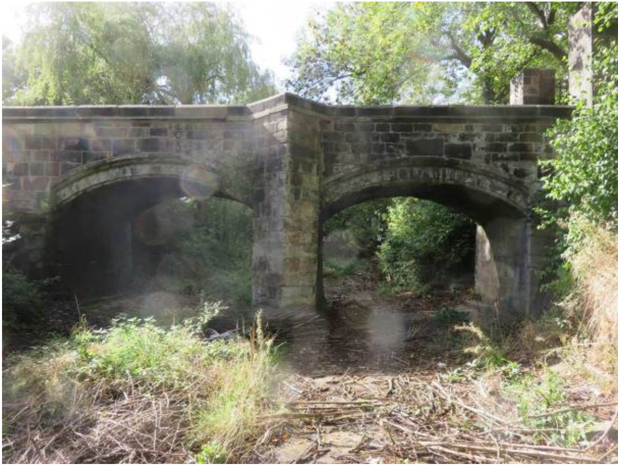
Photograph 3: Bridge over moat to south of site
