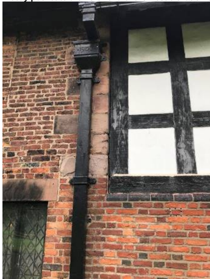
Photograph 39A: Opening up between timber frame panel and adjacent masonry wall structure
