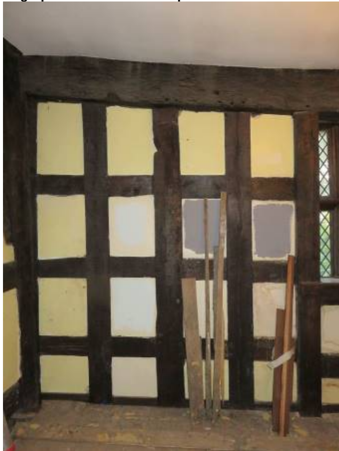
Photograph 15: North wall panel to north bay to east side with clear later introduced timbers
