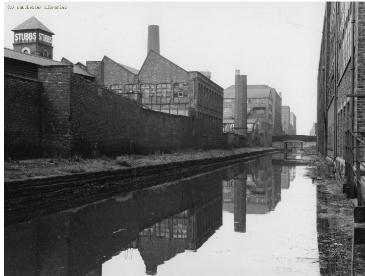
Plate 2: Stubbs Iron Foundry c.1960, looking southeast from the canal. Manchester Libraries
