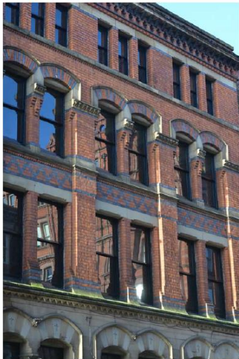
Fig. 6: Architectural detail on the Dale Street elevation
