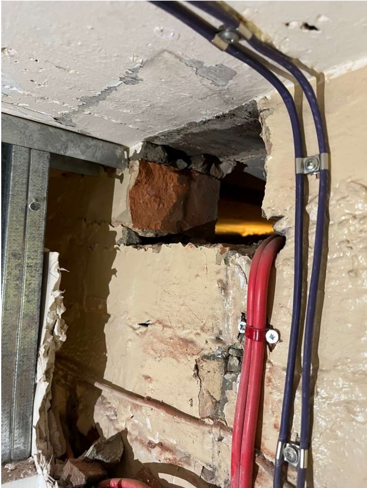
Photo 1 – Position [1] - View of the partition wall's opening works.
