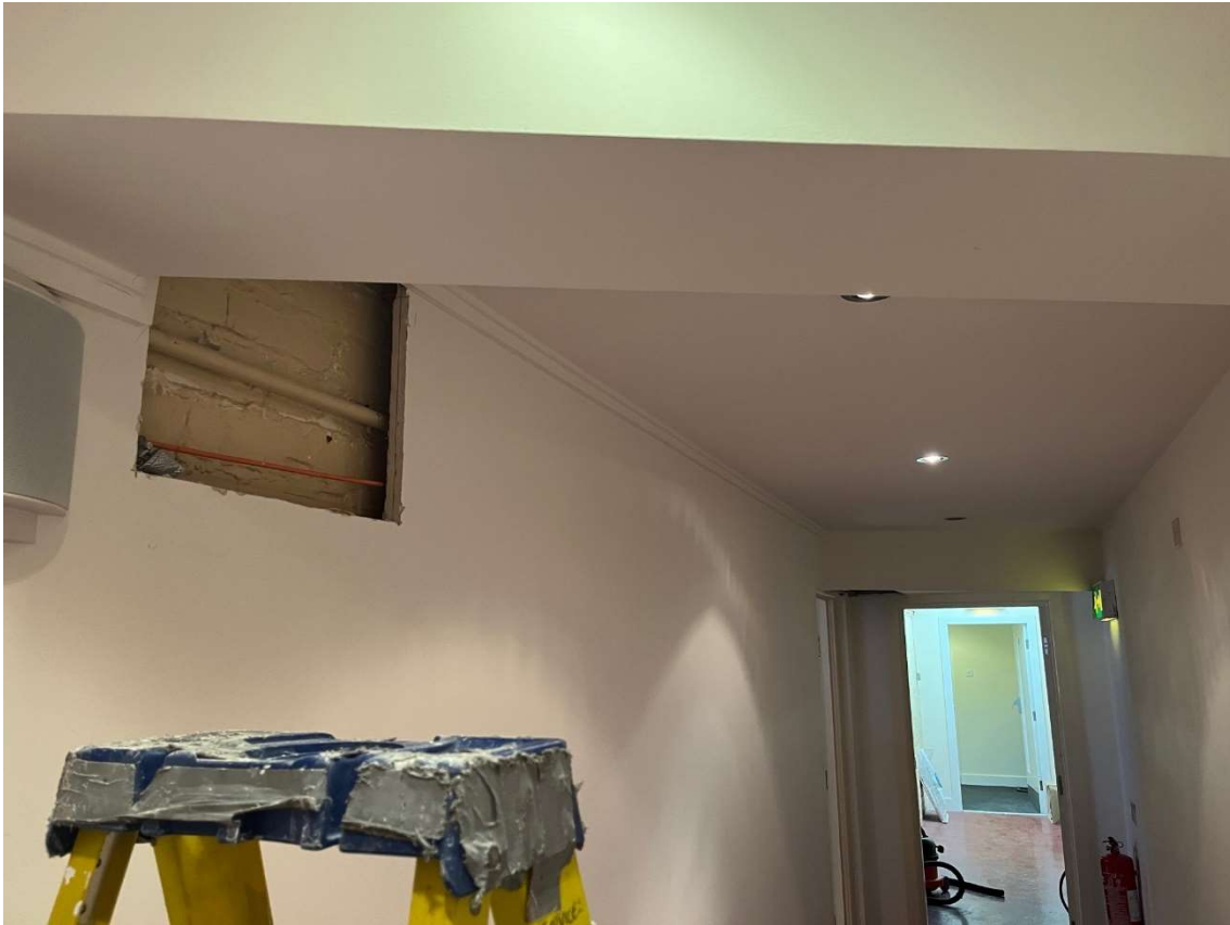
Photo 2 - Corridor for the far end to show both of the opening up works completed to expose downstand beams and wall.
