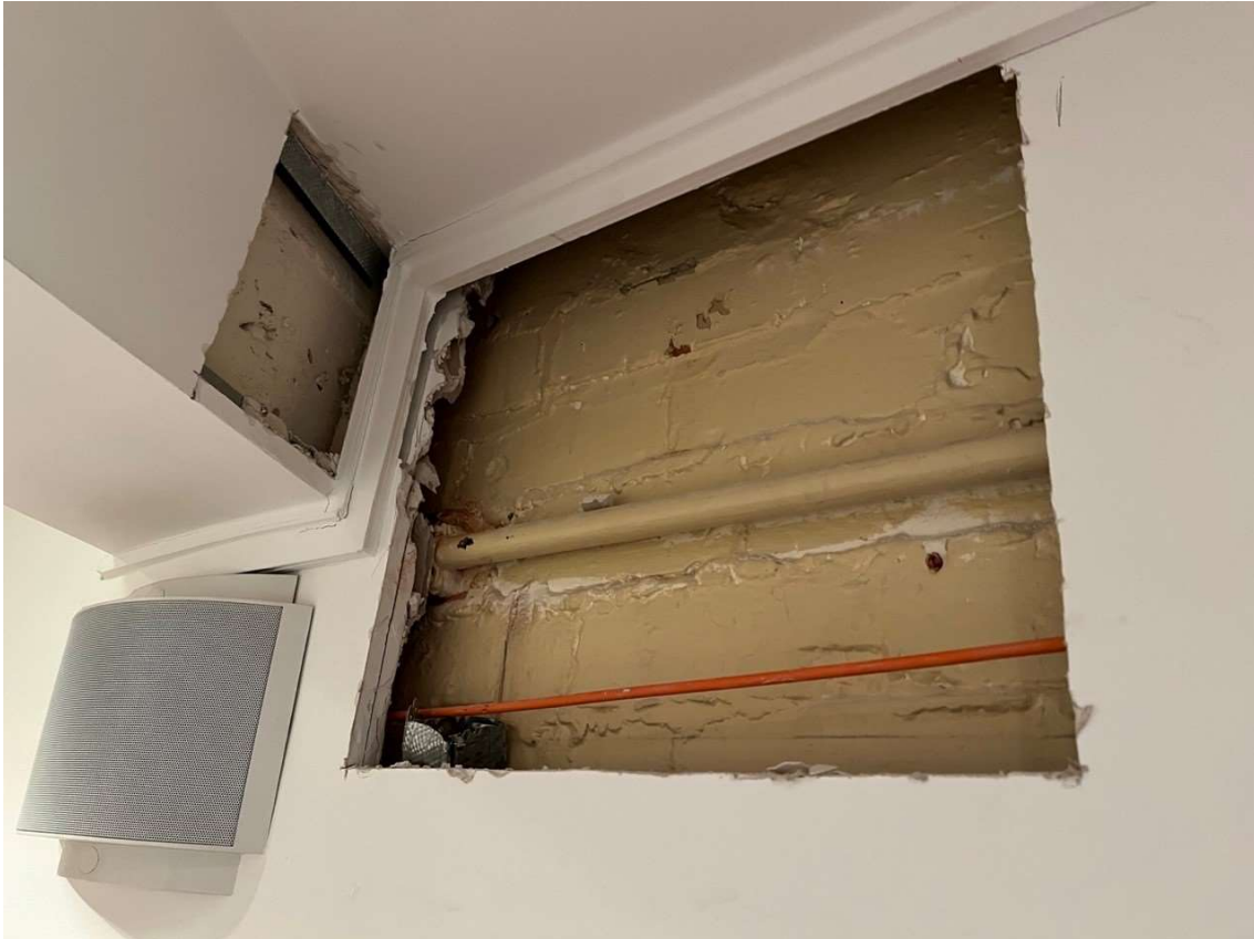
Photo 3 – Position [2] – Exposure of partition brickwork wall and downstand beam.
