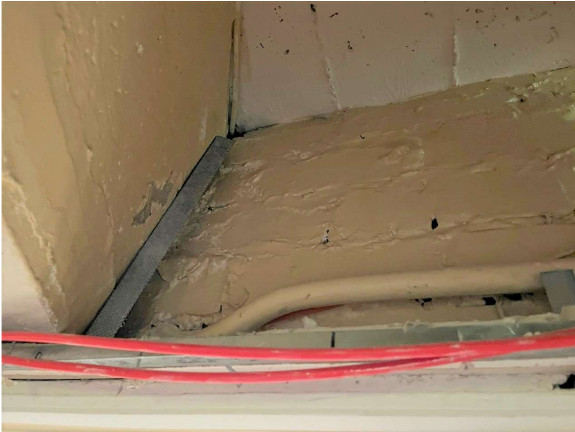
Photo 4 – Position [2] – link between RC downstand beam and brickwork wall.
