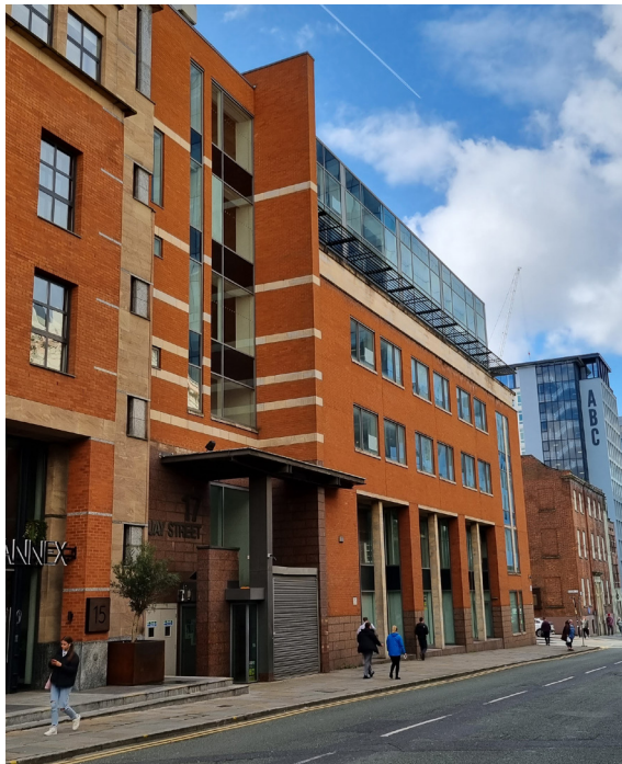
QUAY STREET ELEVATION AND ENTRANCE AREA
