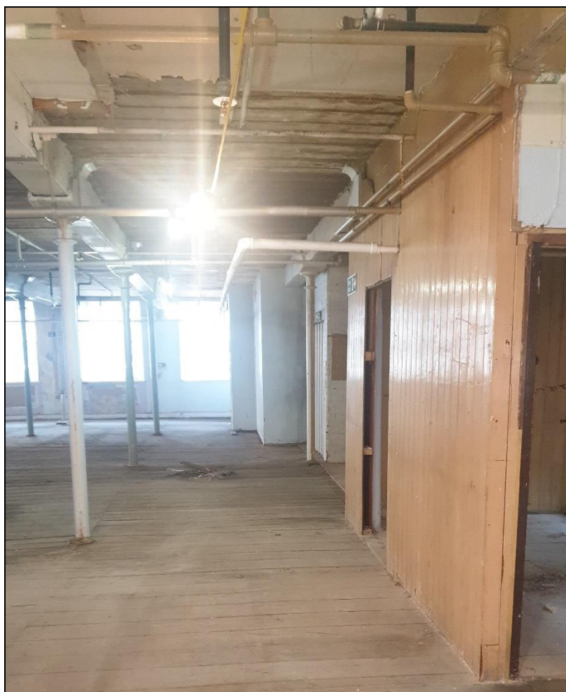
Example of timber panelling found on third floor
