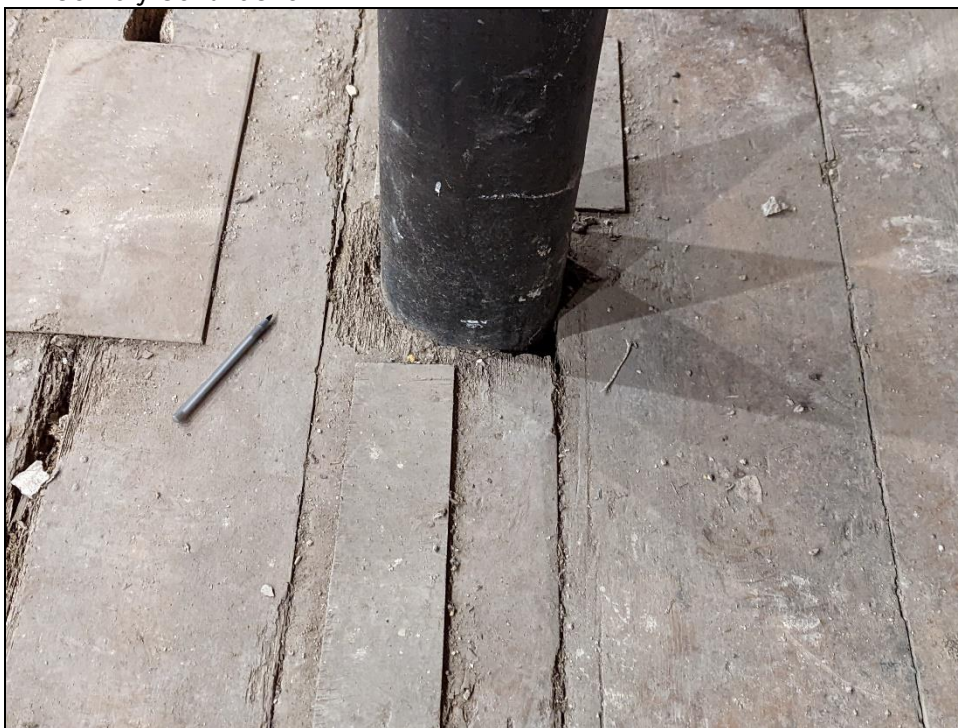
Floorboard finish around stanchion
