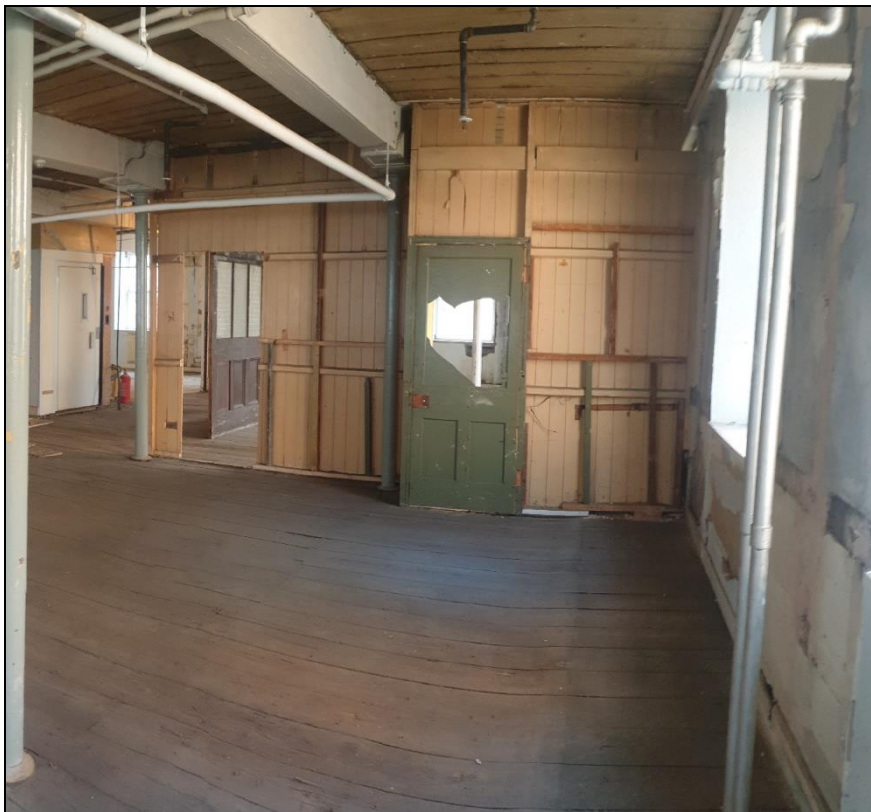
Panelling / partitions on second floor
