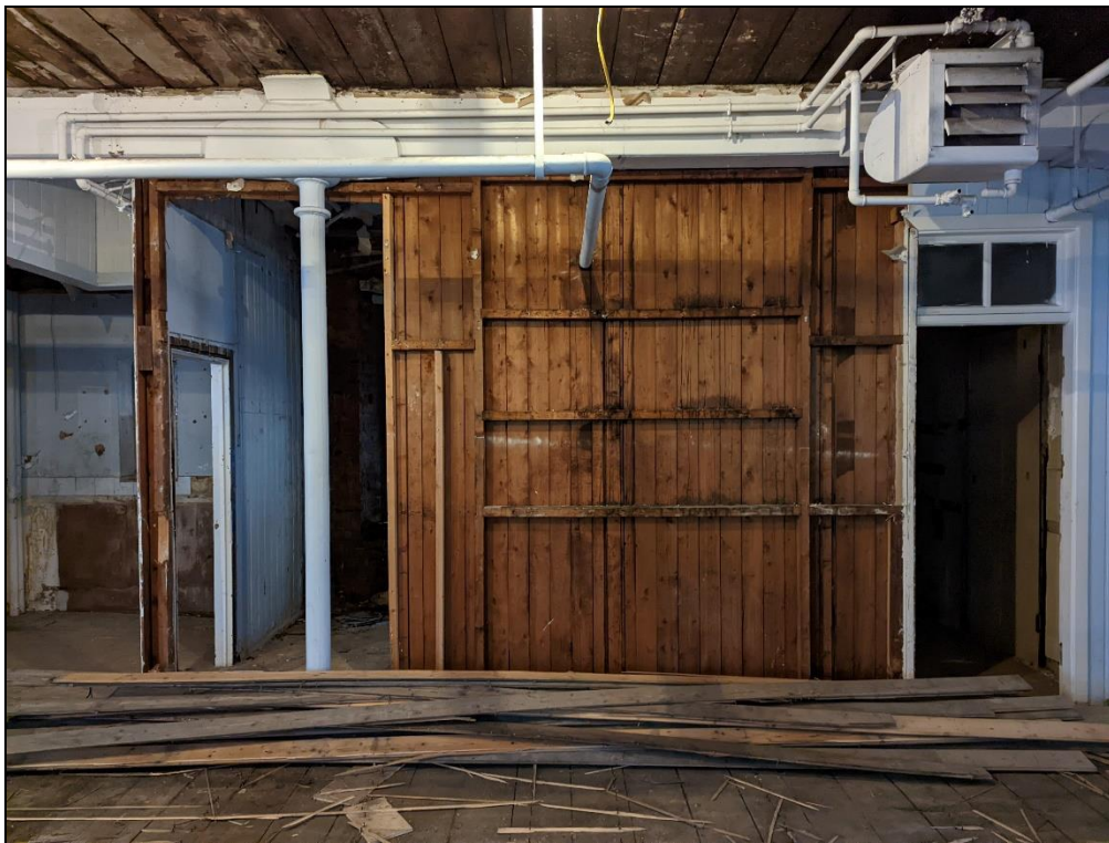
Panelling on first floor
