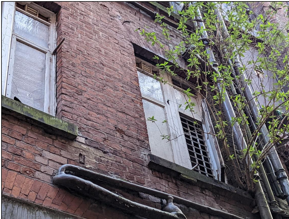
windows as viewed from outside showing inserted timber mullion in centre
