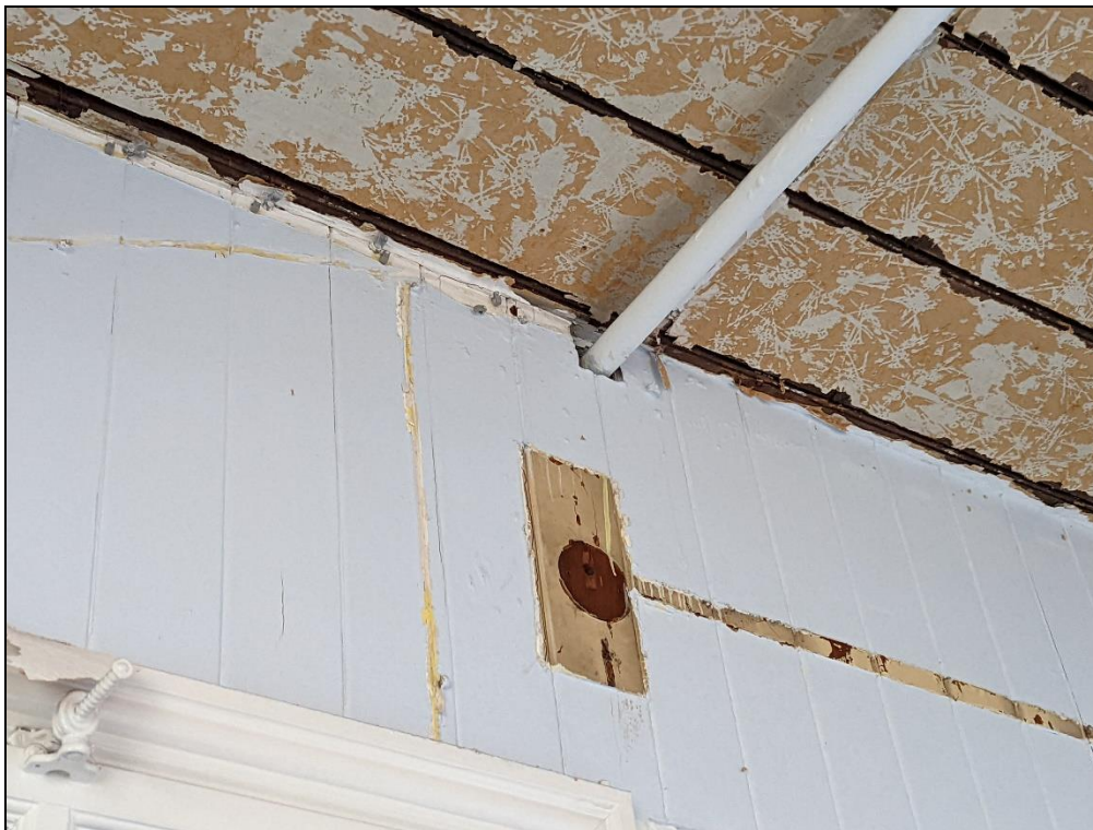
Timber panelling cut around sprinkler system
