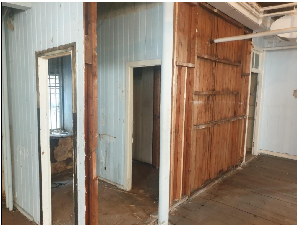
Panelling forming toilets on first floor
