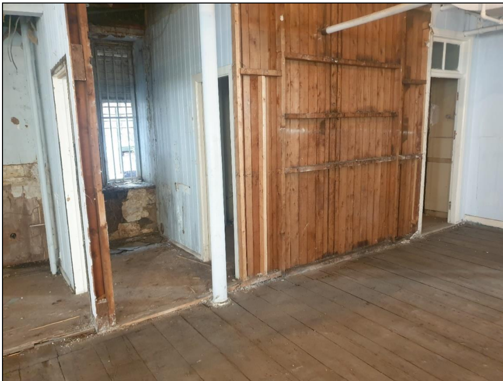
Panelling forming toilets on first floor
