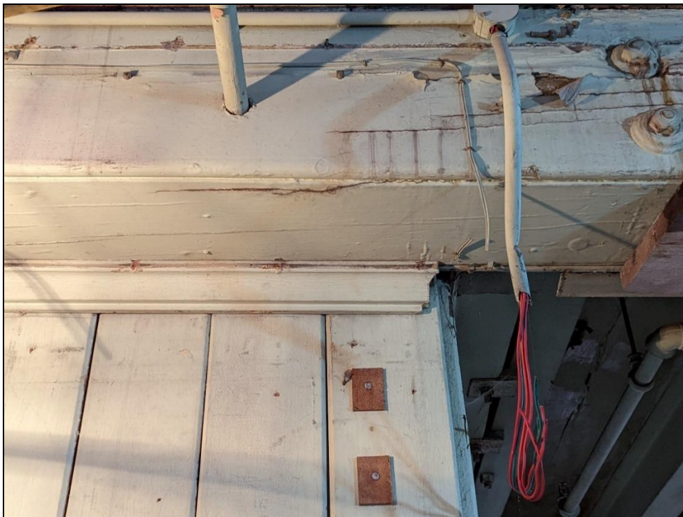
Rough finish of panelling around lift
