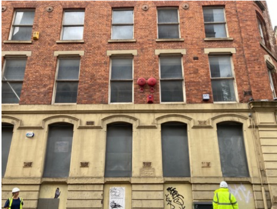
Photo 3B Exterior of building showing red painted rotary alarm gongs
