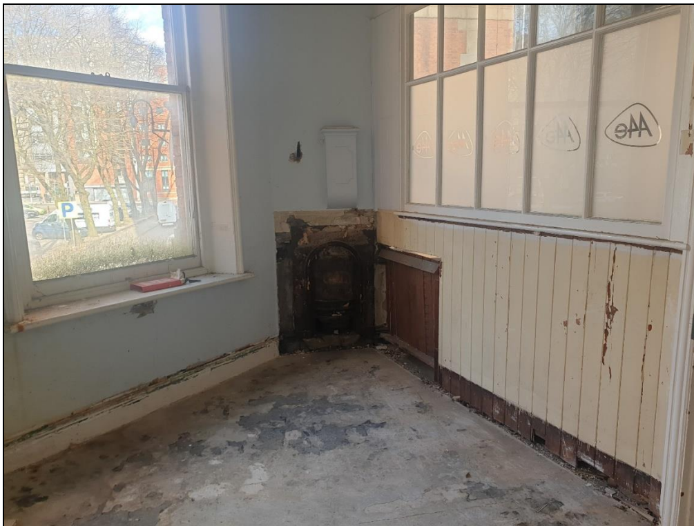
Timber panelling up to revealed fireplace floor
