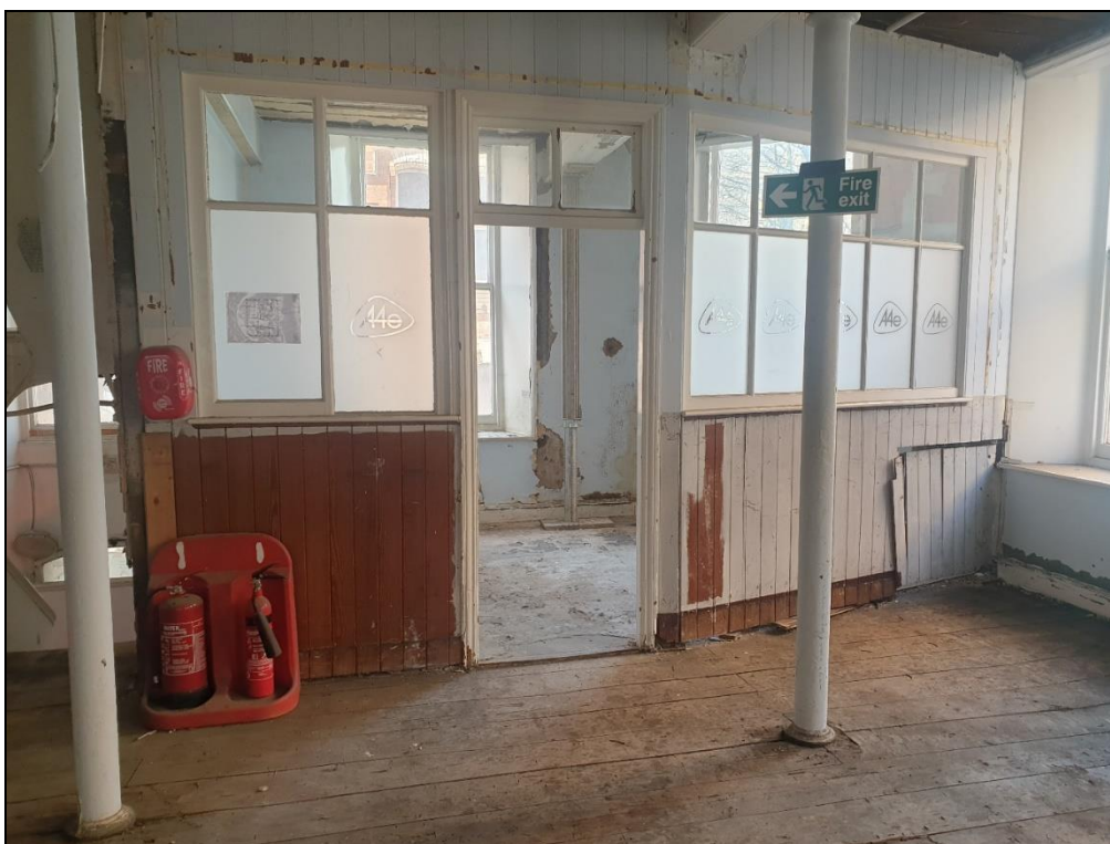
Timber panelling forming office of first floor
