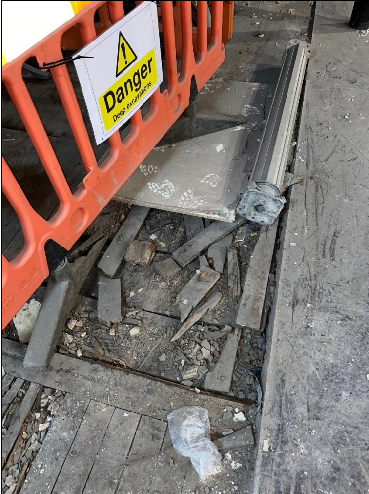
Historic boards around the lift shaft at basement level.
