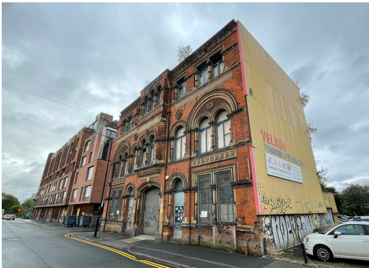
View from the North-west, (2021), showing the metal cladding to the west elevation with cement render visible at low level.
