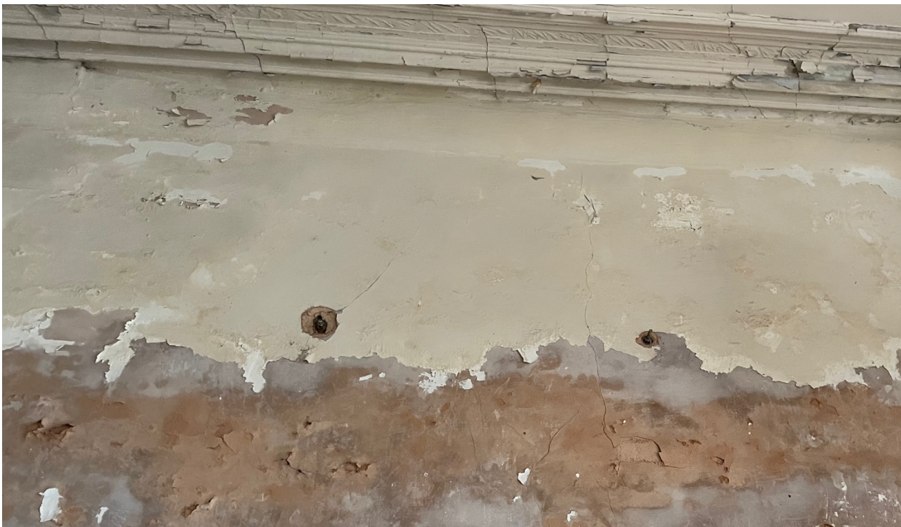
Internal fixings associated with metal sheet cladding (2022).
