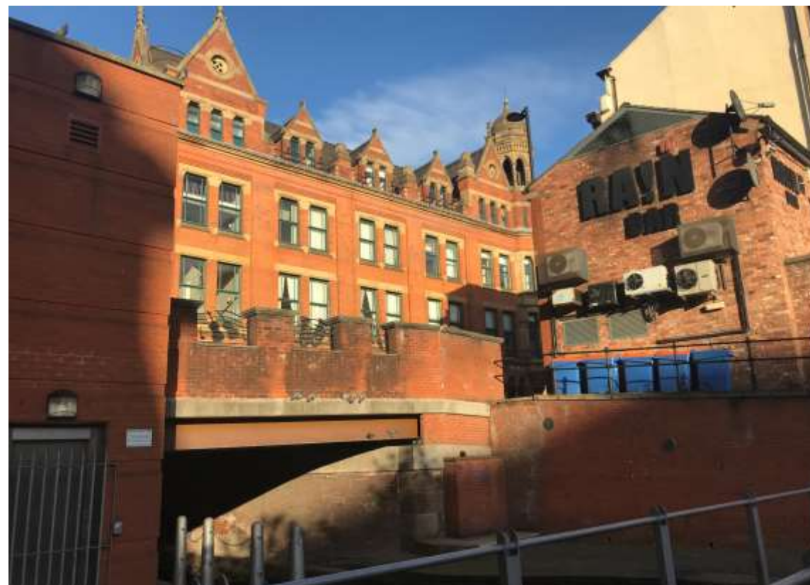
Figure 14: Photograph showing Chepstow House from the lock.
