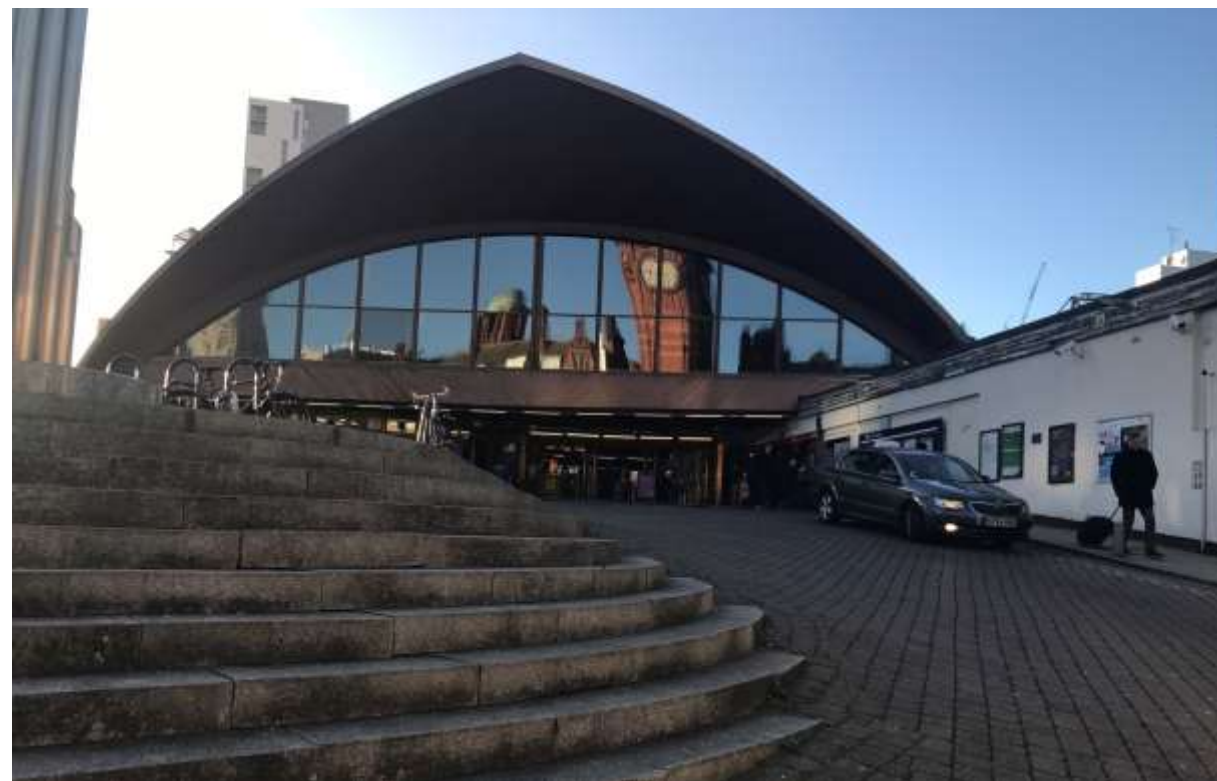
Figure 10: Manchester Oxford Road Station front entrance.
