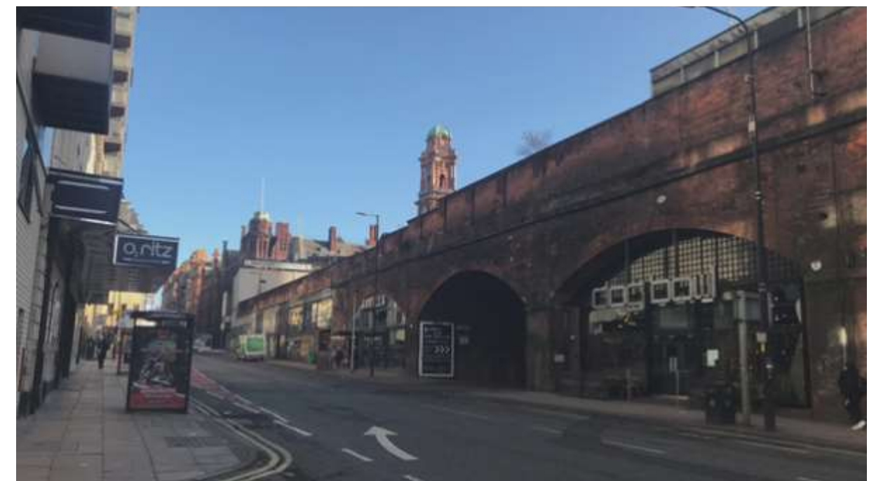
Figure 9: Photograph showing the railway arches near the Ritz Dance Hall, the Oxford Road Station is located on top of the arches, not visible from the street level in close proximity.
