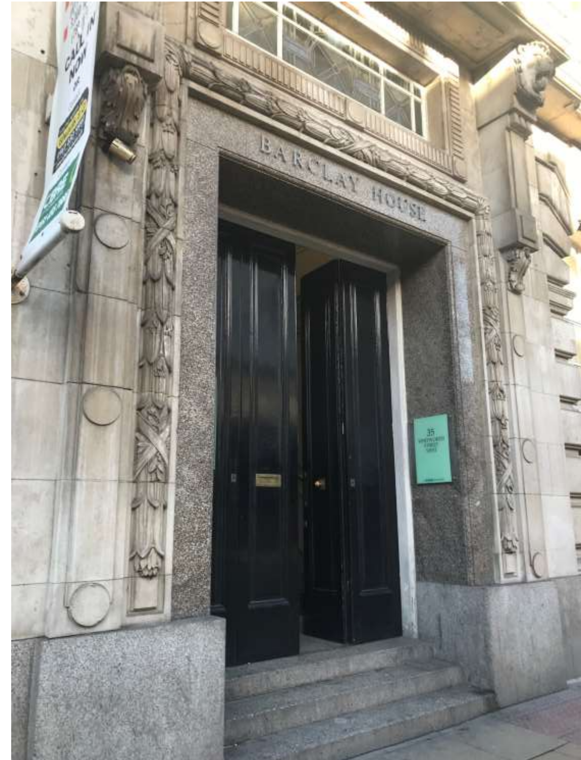
Figure 23: Photograph showing the entrance to Barclay House located on Whitworth Street West.
