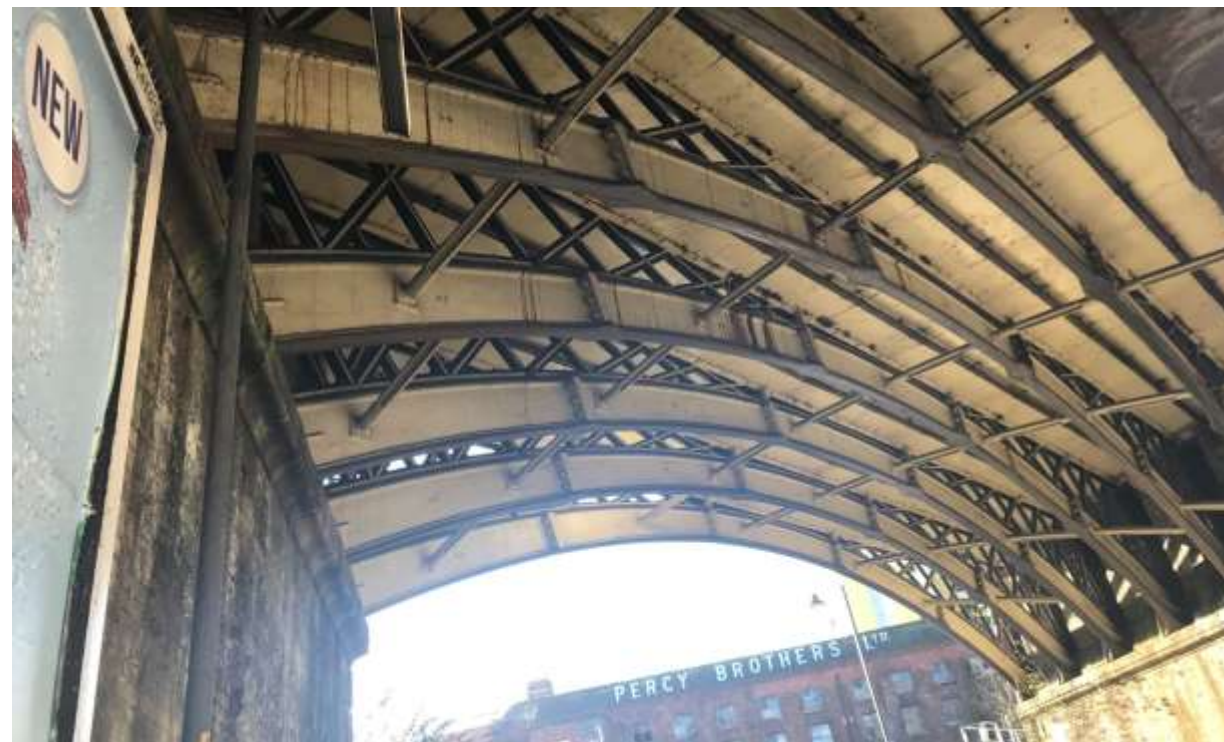
Figure 8: Photograph showing the railway arches over Gloucester Street at the junction with Whitworth Road West, opposite the Site.
