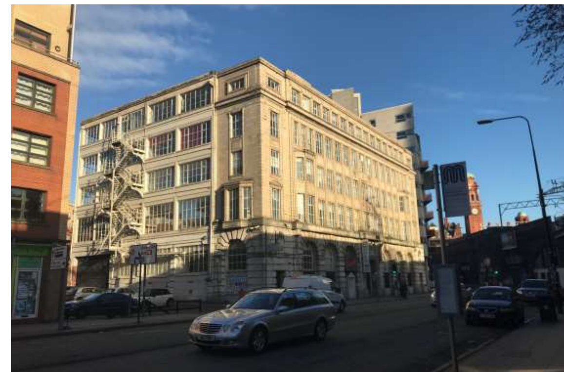
Figure 21: Photograph showing Barclay House viewed from Whitworth Street West, looking east
