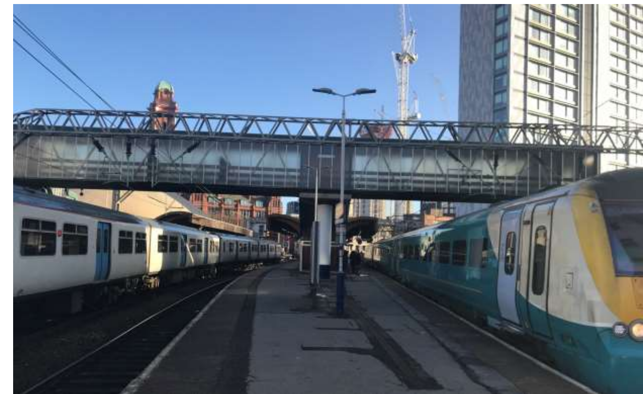
Figure 11: View along the platform of MORS.
