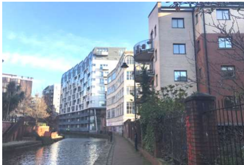
Figure 12: Photograph showing the view from the lock towards the Site
