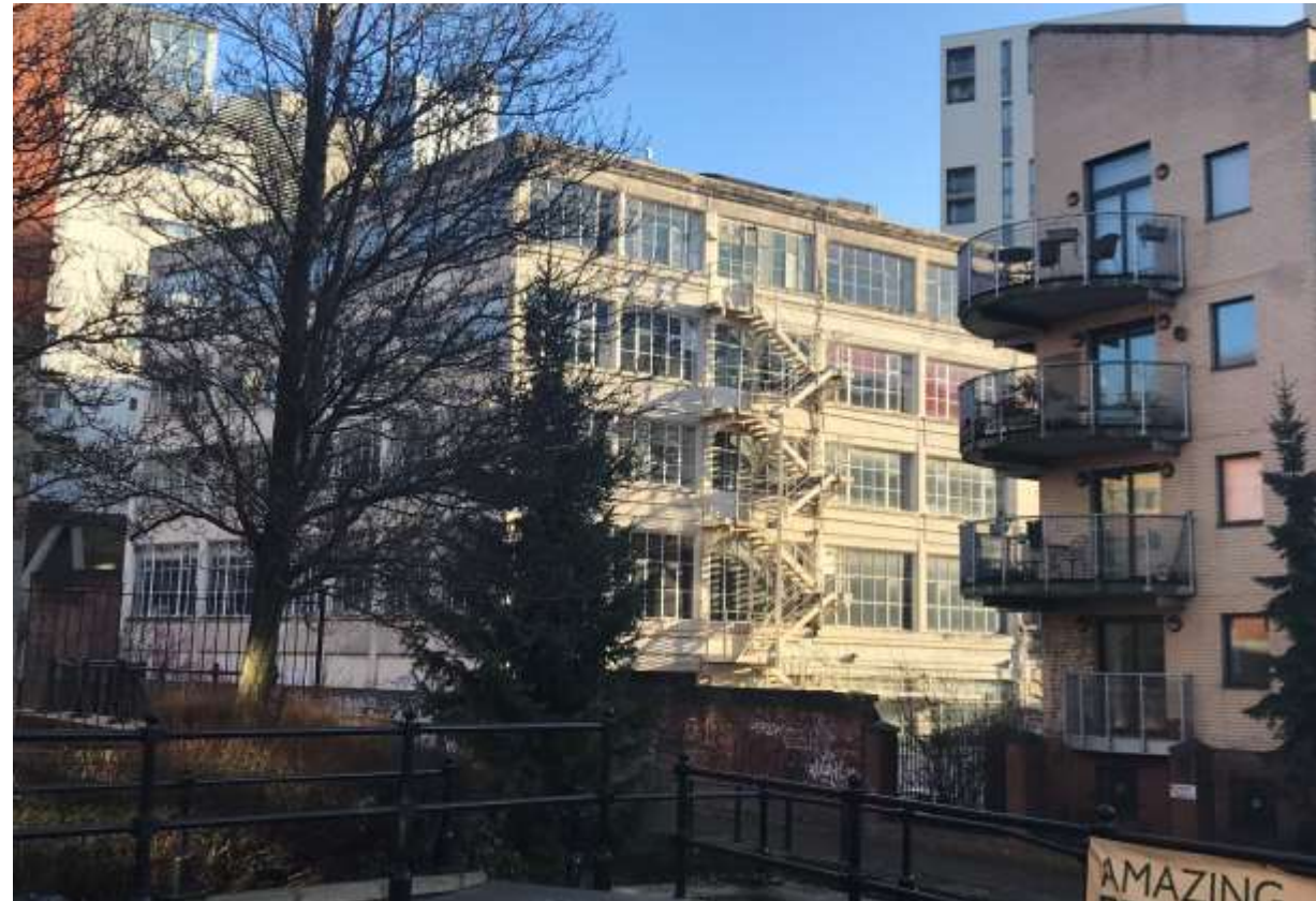
Figure 22: View of the west and north elevations of Barclay House from the Rochdale Canal tow path.
