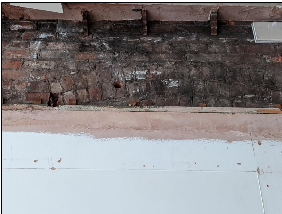
Plate 83: Detail of visible window lintel in former external wall
