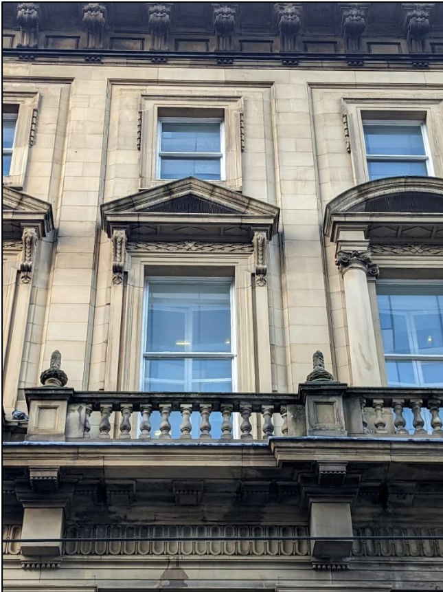
Plate 11: Second and third floor windows
