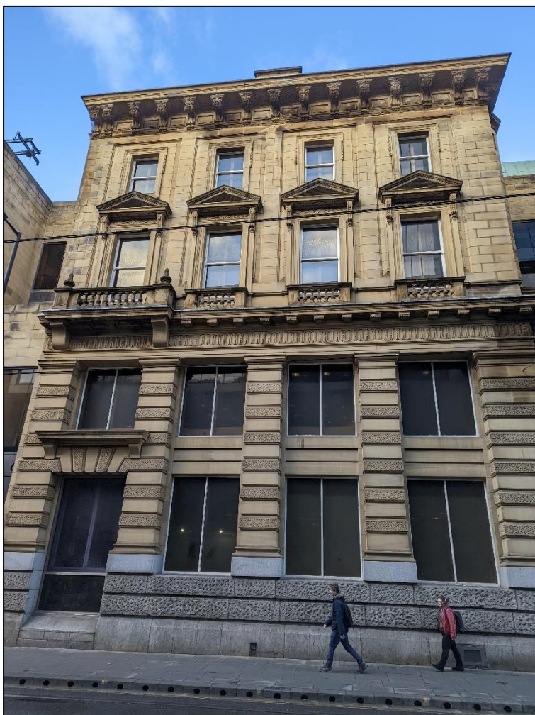
Plate 2: Southern end of elevation showing bays 1 - 4
