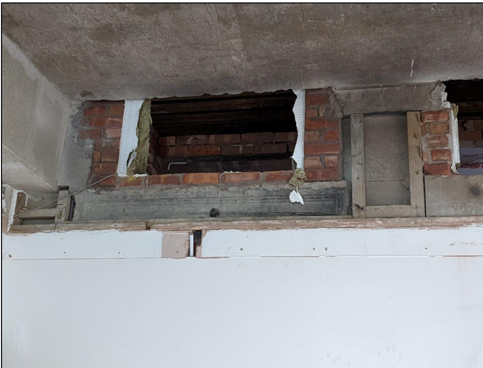
Plate 81: Sandstone lintel of former external window of original building
