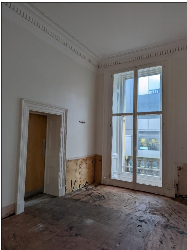
Plate 59: Room as above showing doorway to main central office room
