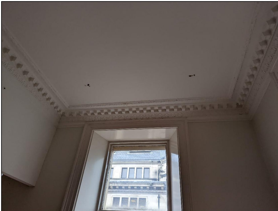
Plate 64: eastern end showing cornice
