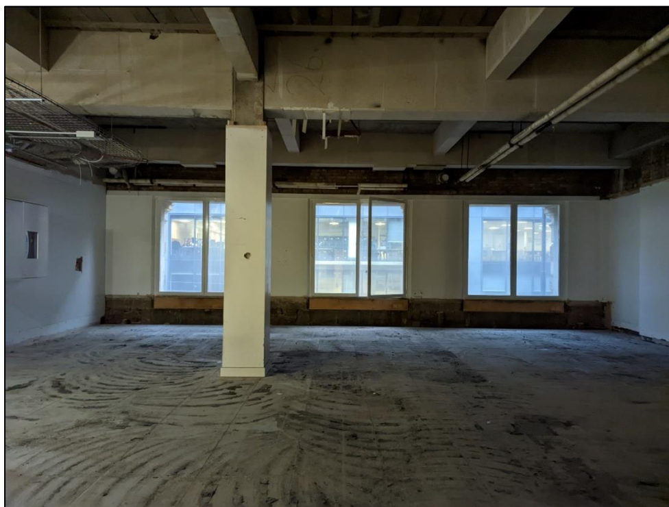
Plate 45: Southern room of extension facing Mosley Street
