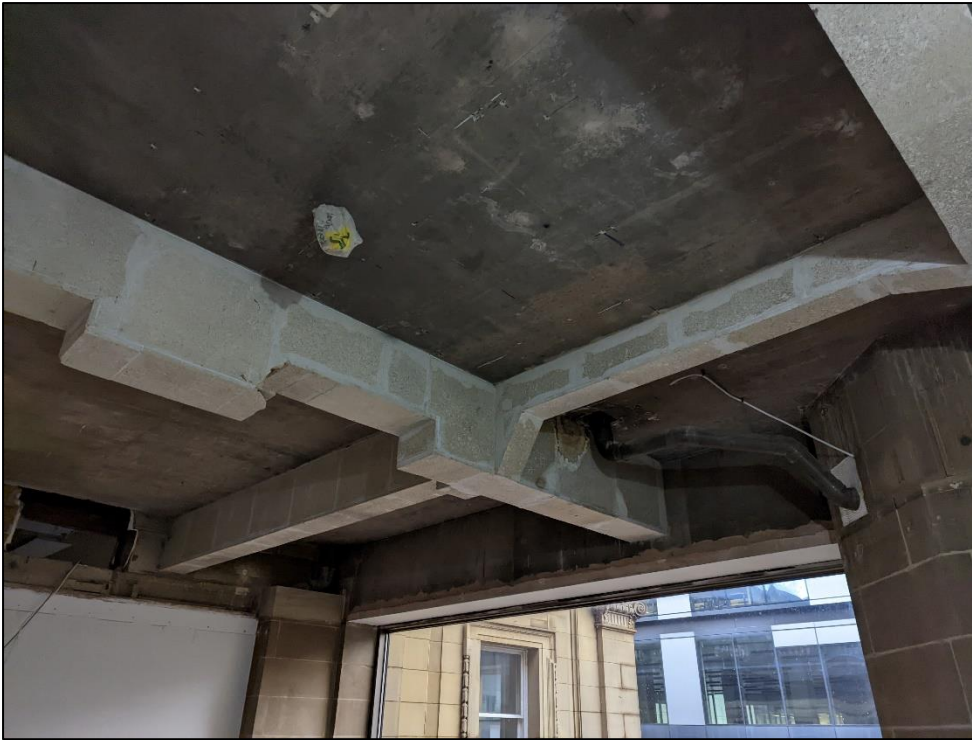
Plate 80: Detail of concrete ceiling construction
