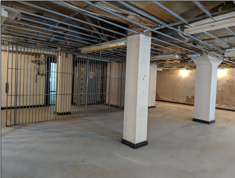
Plate 110: Southern room of original building
