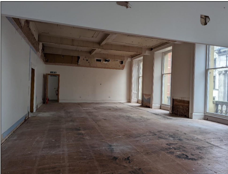
Plate 63: Northern room of original building
