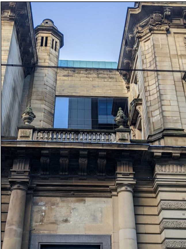
Plate 8: Recessed second and third floors at bay 5
