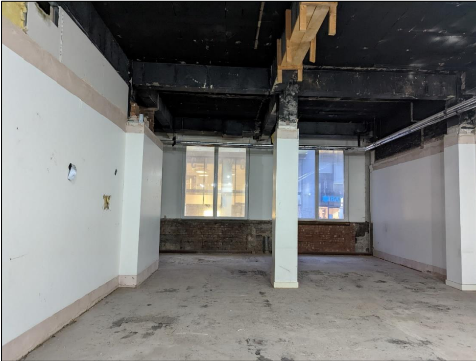
Plate 27: Southern Room showing windows to Mosley Street
