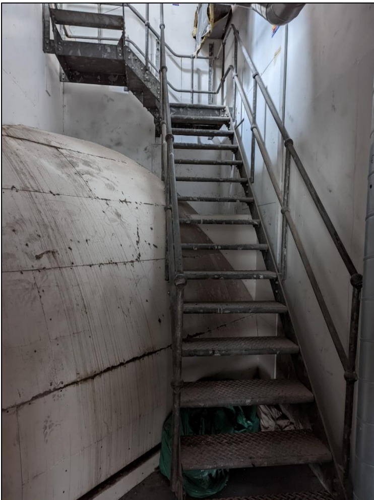
Plate 93: Metal staircase to roof access
