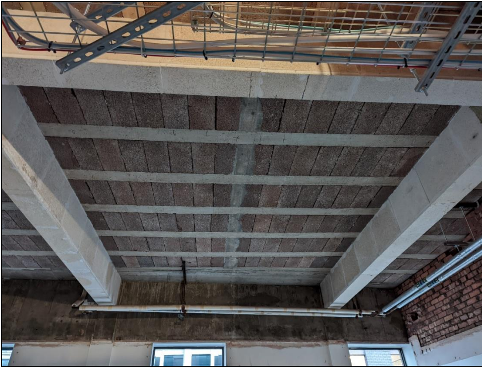
Plate 53: Detail of concrete ceiling construction throughout extension
