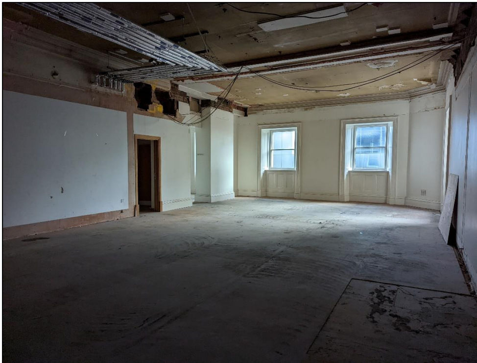
Plate 82: Room to southeast corner of original building
