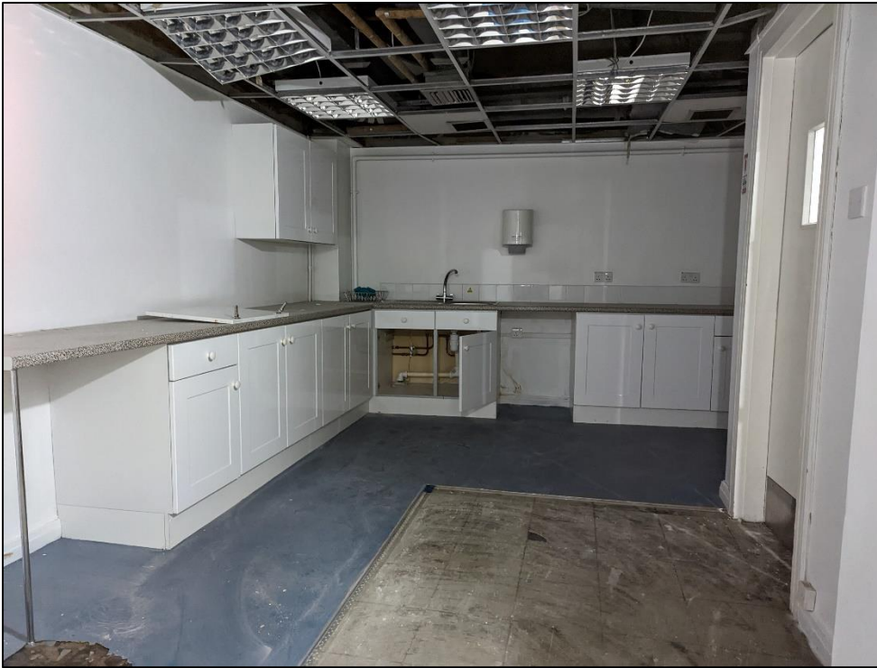
Plate 116: Inserted kitchen to southwest end of extension
