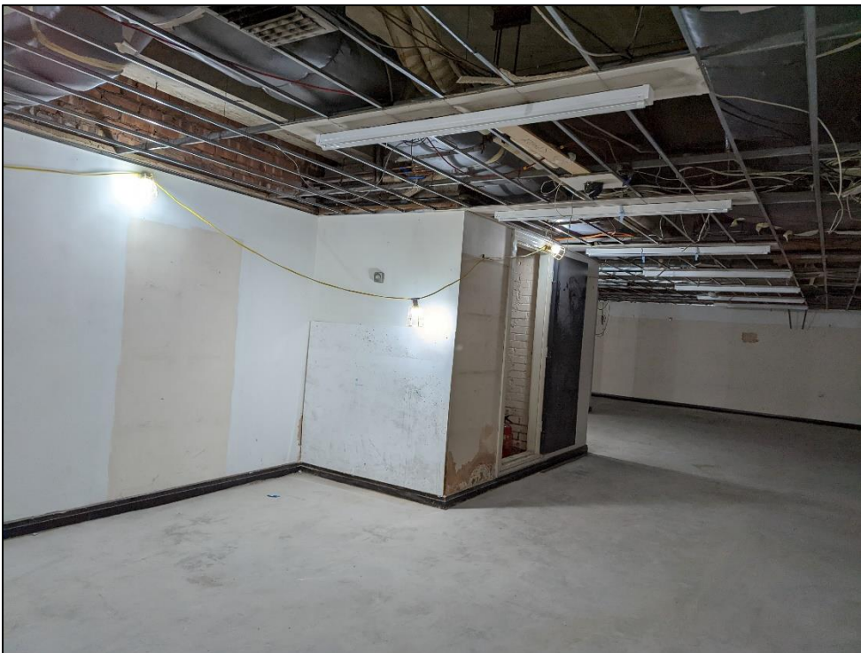
Plate 111: Room to northeast corner of extension
