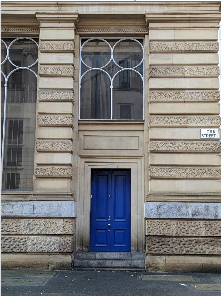
Plate 16: Doorway in bay 6
