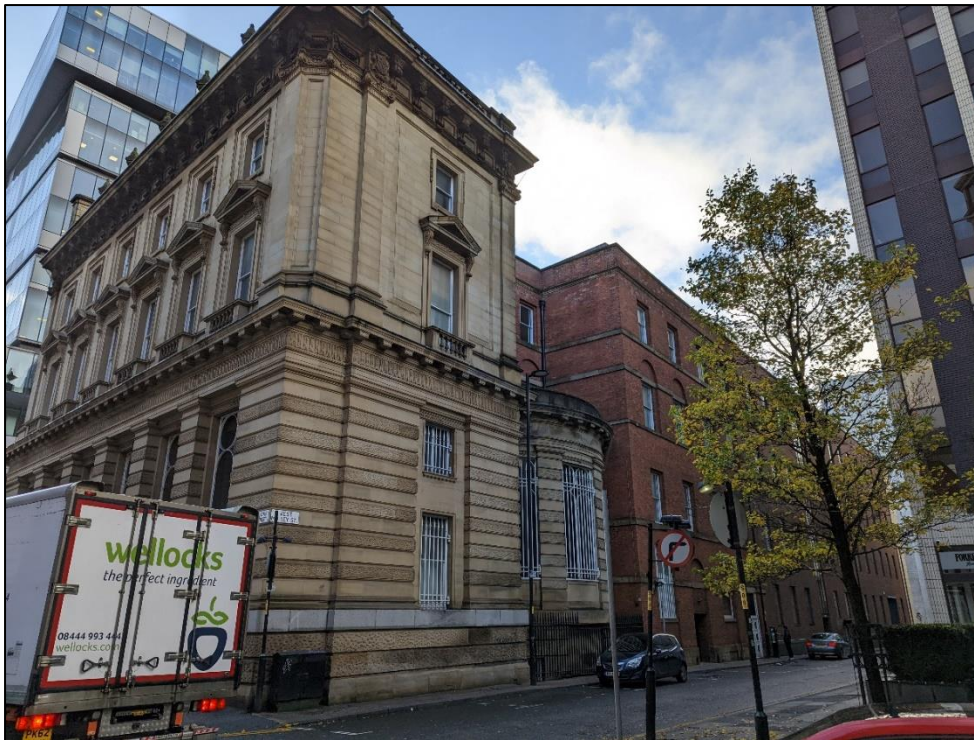
Plate 17: Elevation to West Mosley Street
