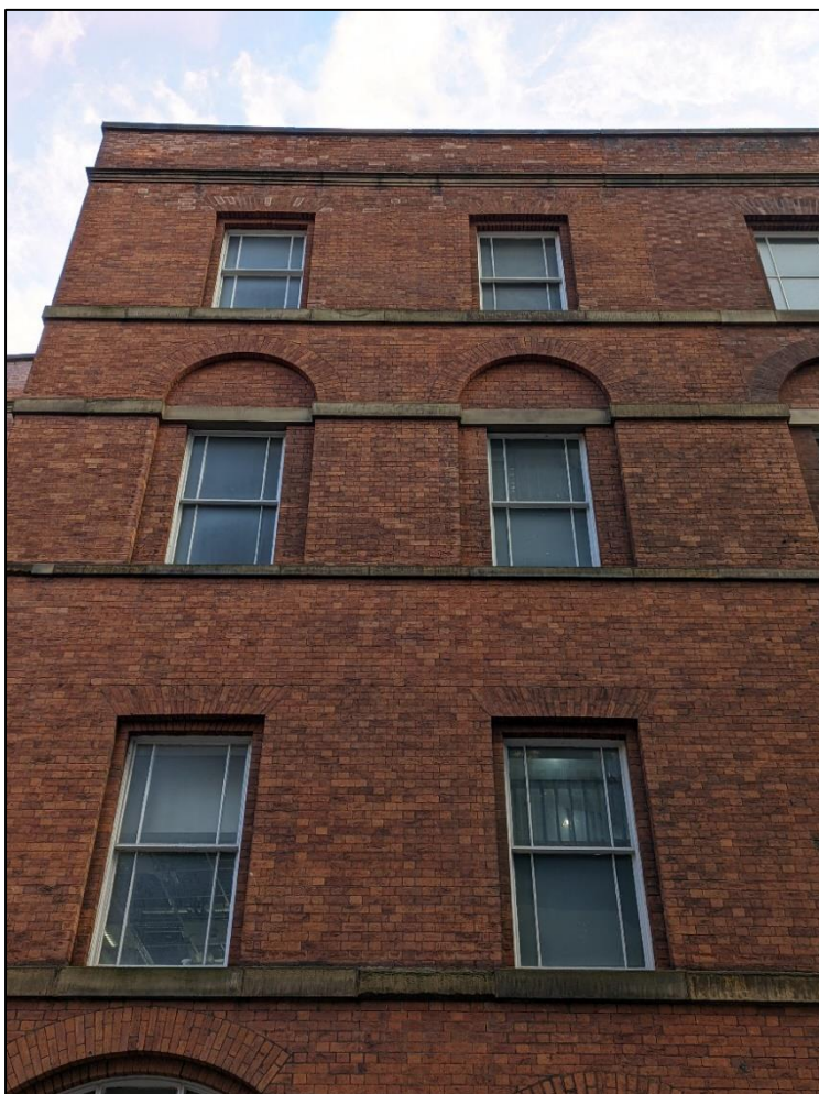
Plate 24: Upper floor windows in bays 5 and 6
