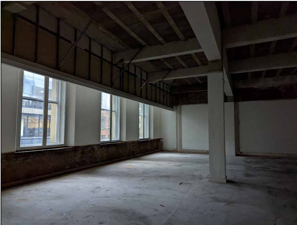
Plate 55: Open area to southeast corner of extension showing windows to Mosley Street
