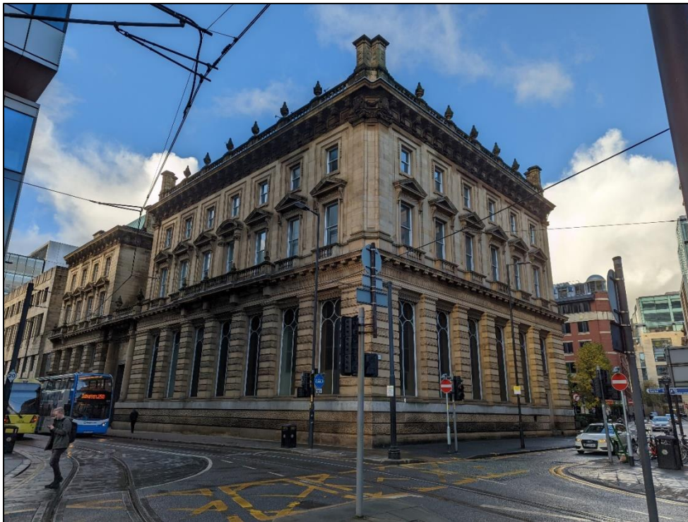
Plate 1: General shot of building showing corner of Mosley Street and York Street
