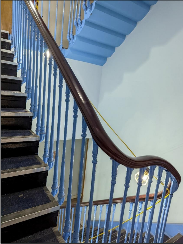
Plate 54: Staircase in southwest corner of original building
