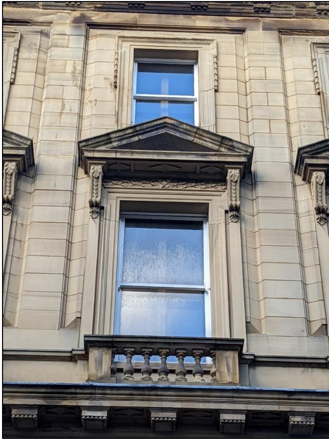
Plate 5: Second floor window detail
