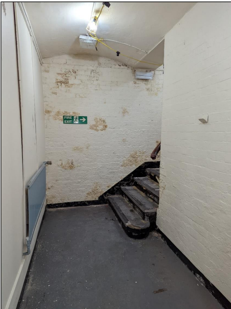
Plate 103: Staircase in northwest corner
