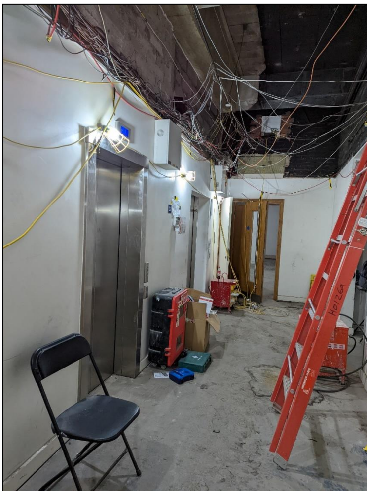
Plate 42: Corridor along west end of the building, running south
