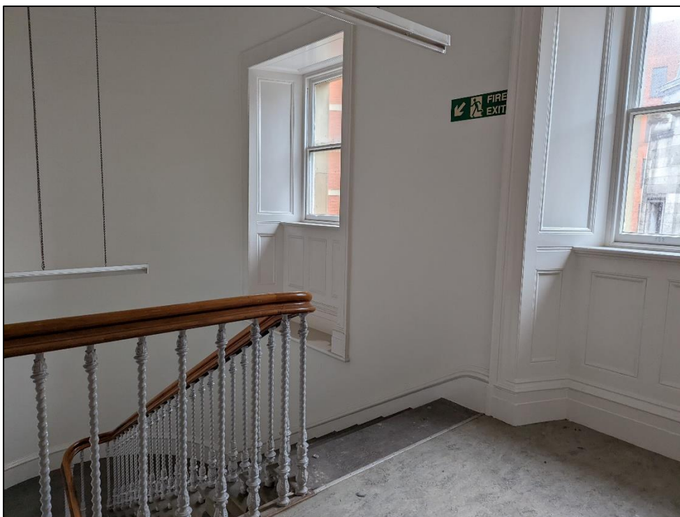
Plate 95: Staircase in northwest corner
