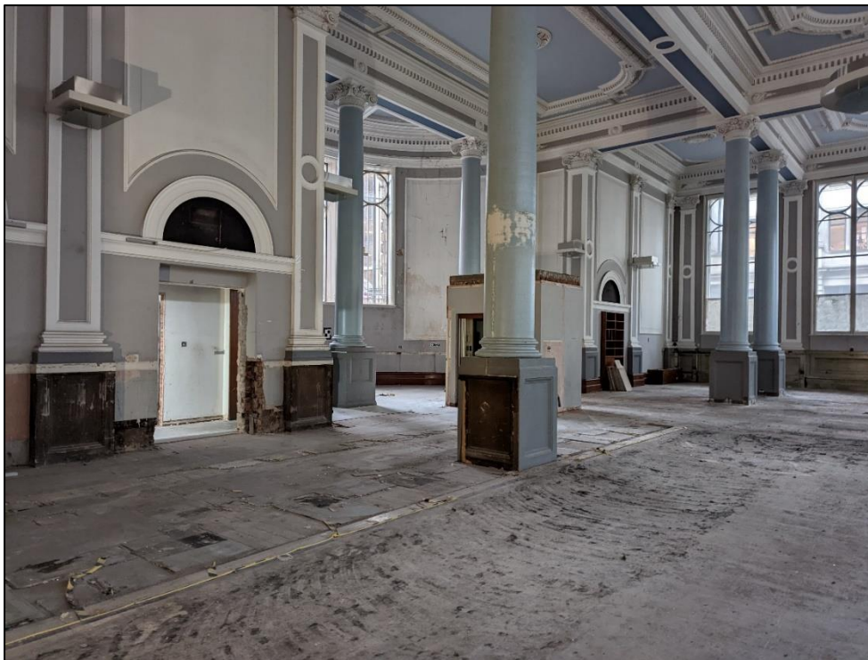
Plate 36: Banking hall looking towards the corner of York Street and West Mosley Street
