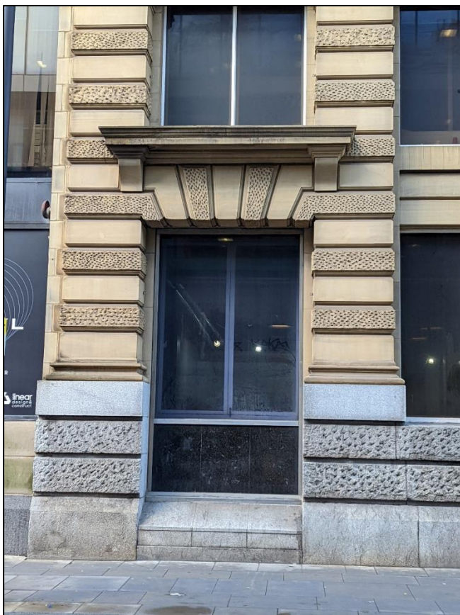
Plate 6: Bay 1 detail showing former doorway
