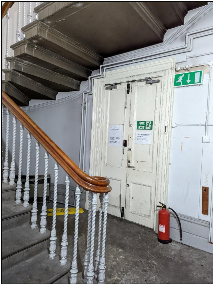
Plate 39: Staircase in northwest corner of building
