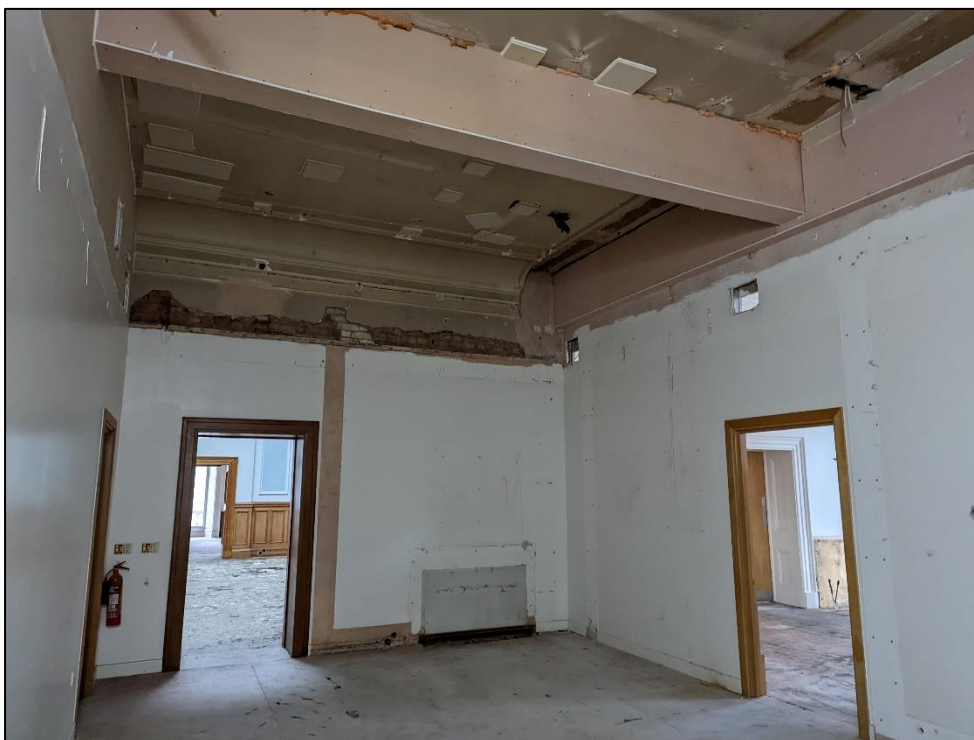
Plate 57: Subdivided room to south end of original building
