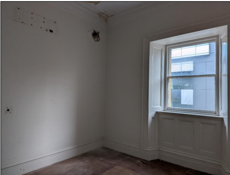
Plate 85: Office to east side
