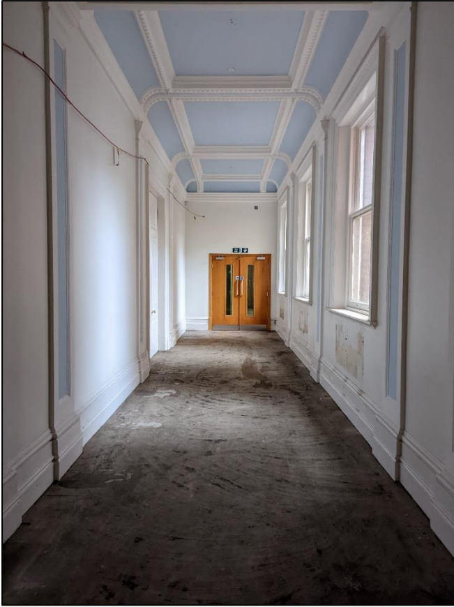
Plate 68: Western corridor linking office rooms
