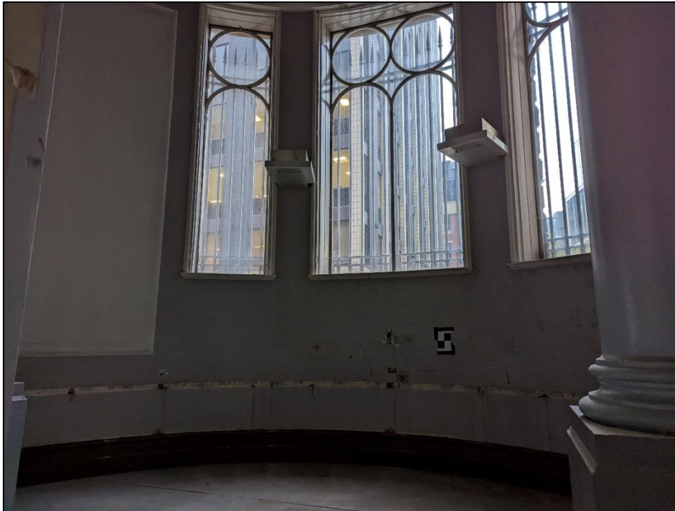
Plate 37: Curved wall to West Mosley Street
