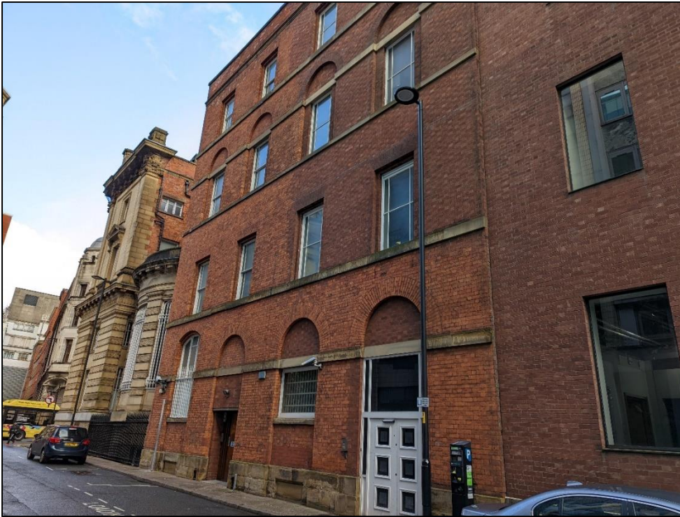
Plate 25: Bays 5 – 8 looking north
