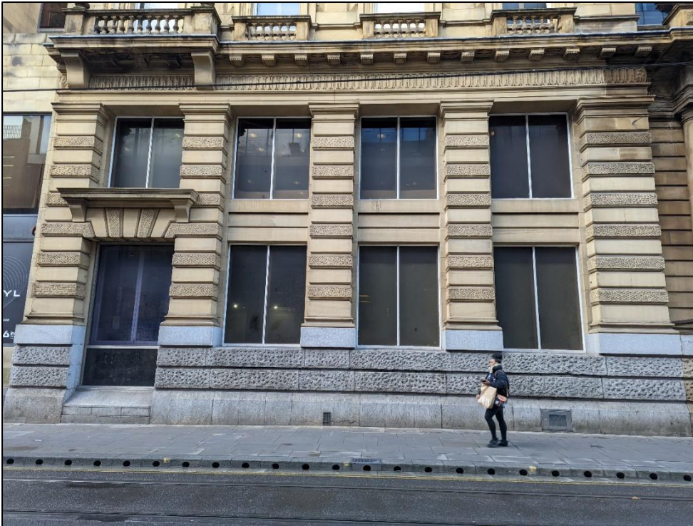
Plate 3: Ground and first floor detail of above
