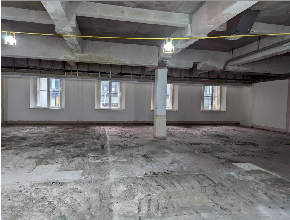
Plate 78: Room to southeast corner of extension
