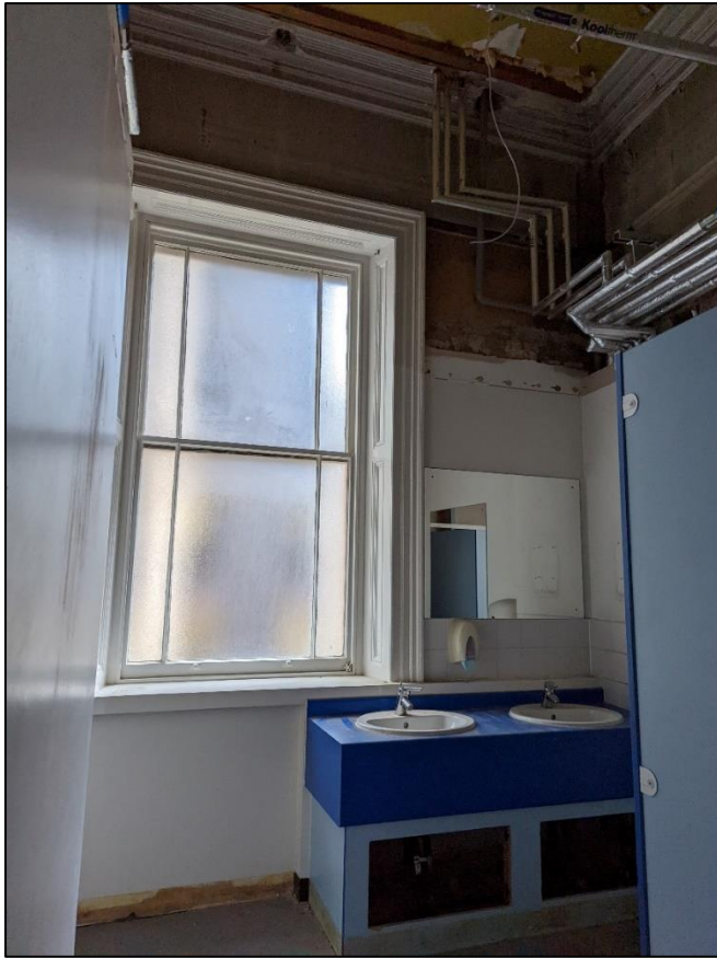
Plate 74: WC off corridor above showing cornice
