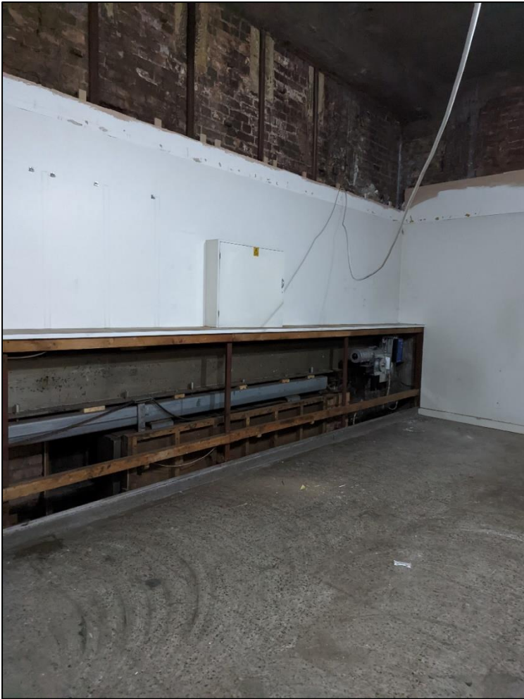
Plate 47: Wall of bay 5 to Mosley Street showing mechanism for opening the sliding doorway below
