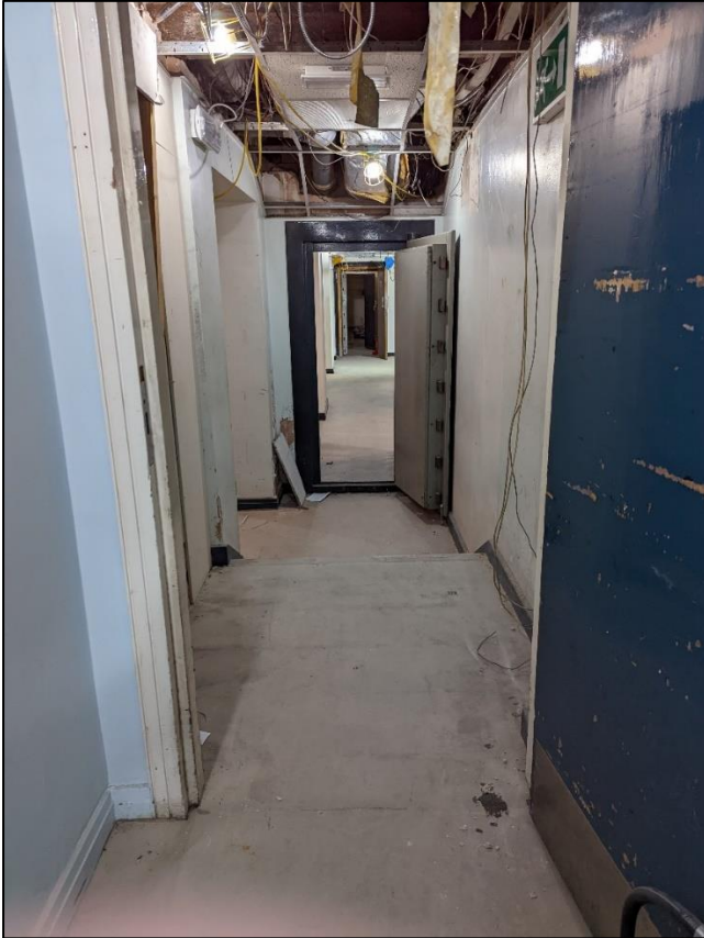
Plate 98: Corridor in southwest corner of original building looking north
