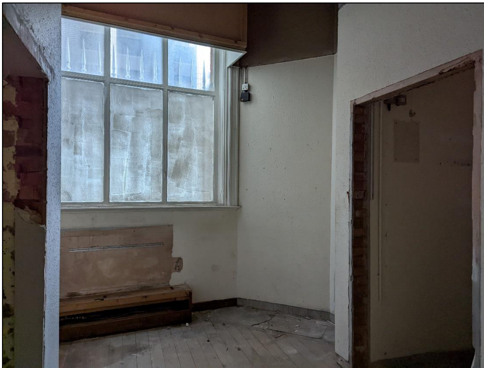
Plate 40: Room to south of curved wall
