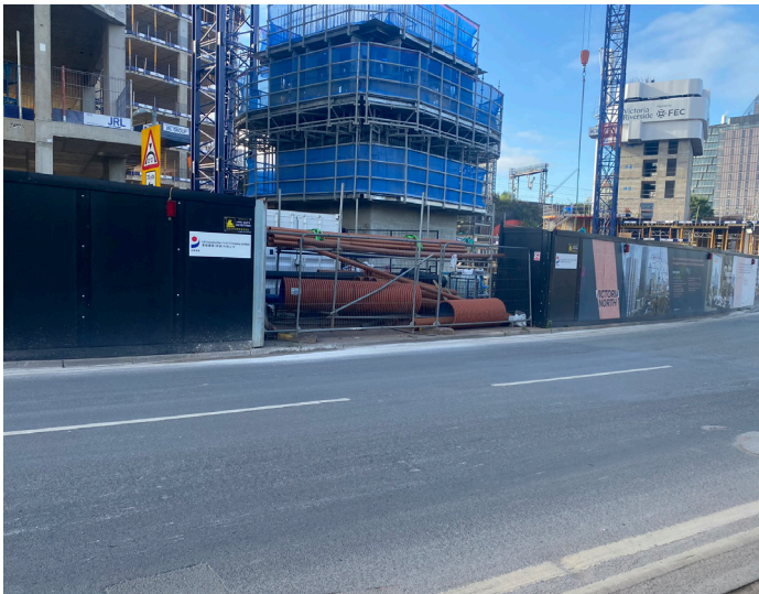
11. Heras fence to hoarding line along Dantzic Street
