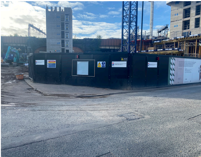
15. Bellmouth from Site Gate No.1 on to Dantzic Street
