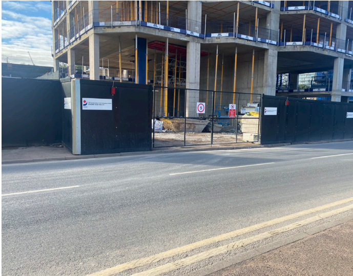
9. Site Gate No.2 on Dantzic Street
