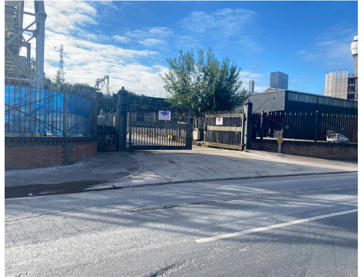
2. Gates of JRL batching plant on Dantzic Street, adjacent to Dulwich Street
