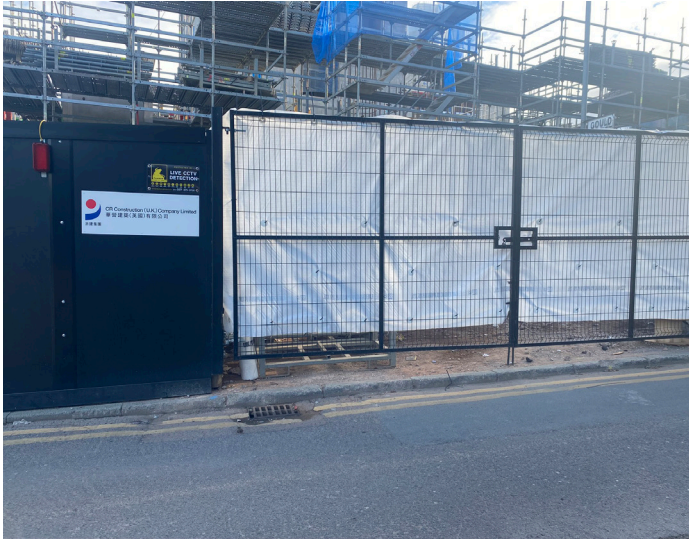
21. Site Gate No.4 on Gould Street
