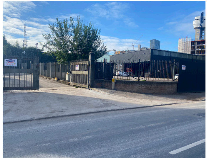
4. Gates of JRL batching plant on Dantzic Street, adjacent to Dulwich Street
