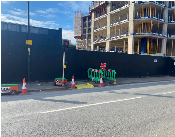
7. Temporary pedestrian crossing across Dantzic Street
