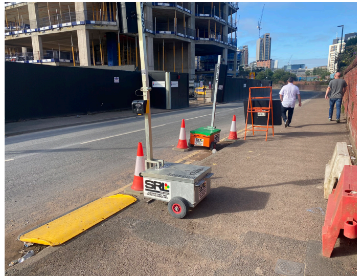
8. Temporary pedestrian crossing onto public footpath on Dantzic Street
