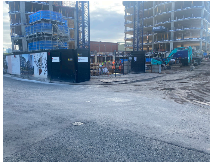
16. Bellmouth from Site Gate No.1 on to Dantzic Street
