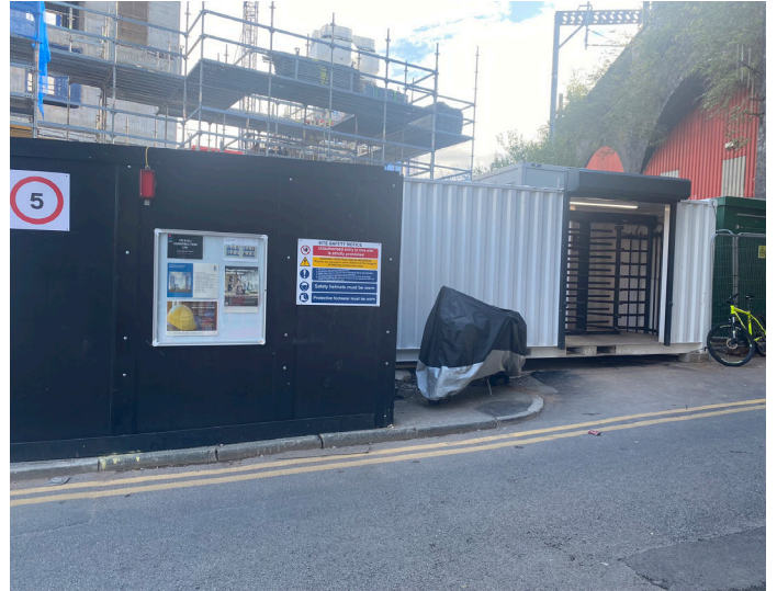
22. Turnstile access to site on Gould Street
