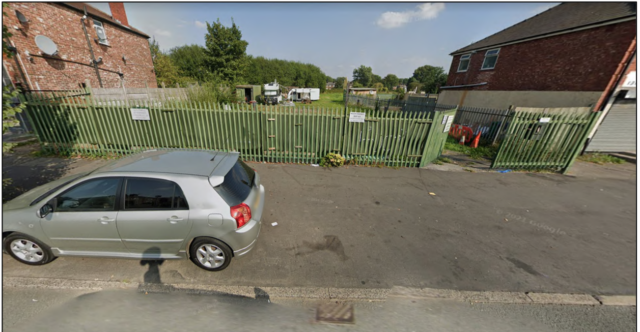
Figure 2.3 – Existing Access off Levenshulme Road
