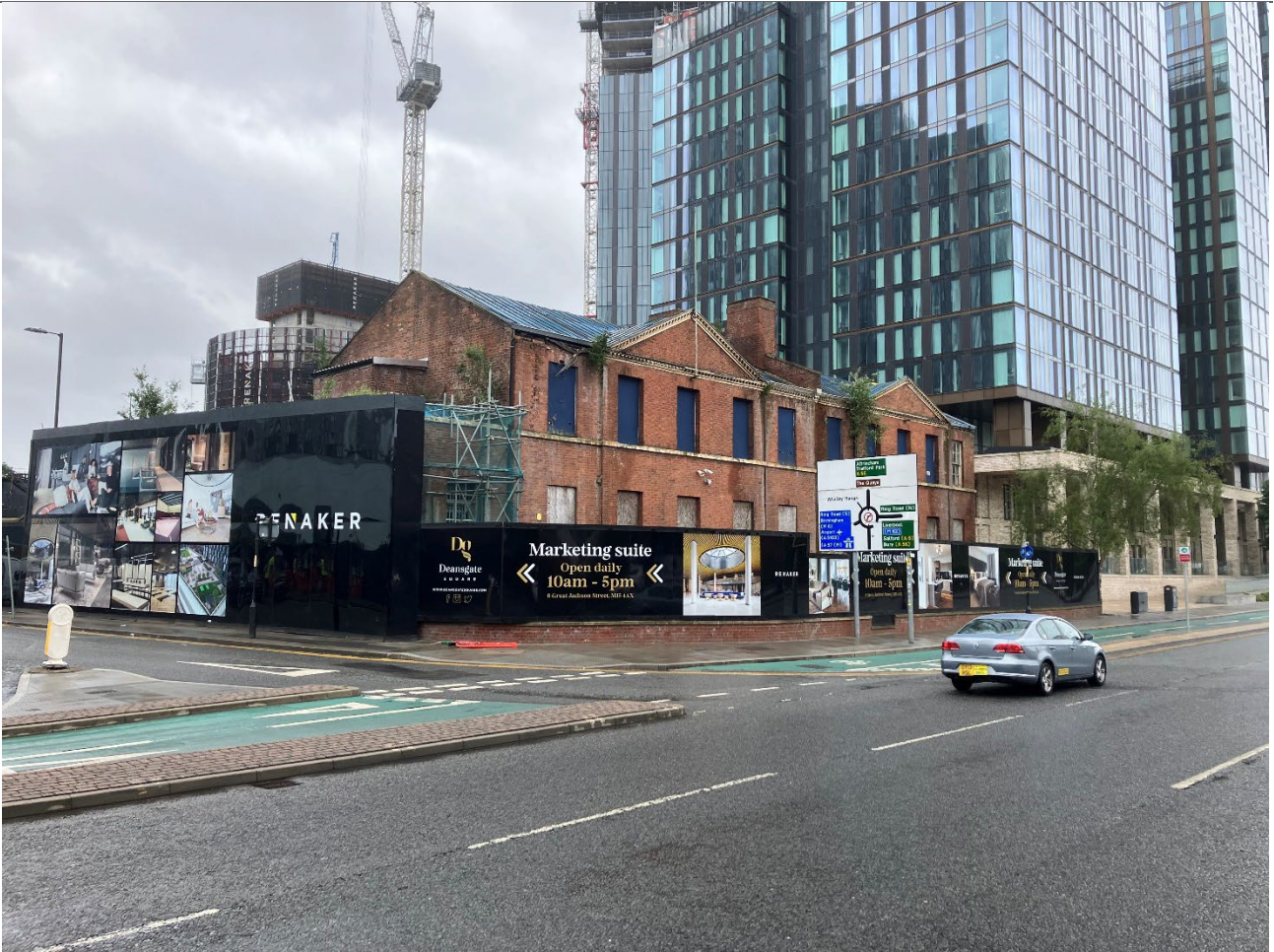
Plate 1: View from Chester Road toward the Grade II Bridgewater Canal Office buildings
