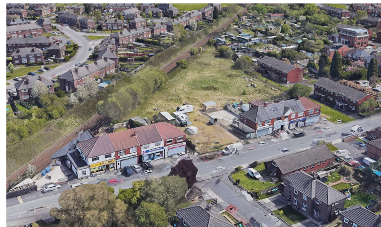
Aerial view of site facing south east
