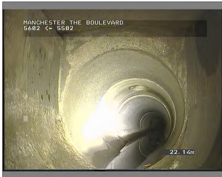
Photo: 1_1_4_A.JPG 22.14m, Finish node type, manhole reference number: 5502
