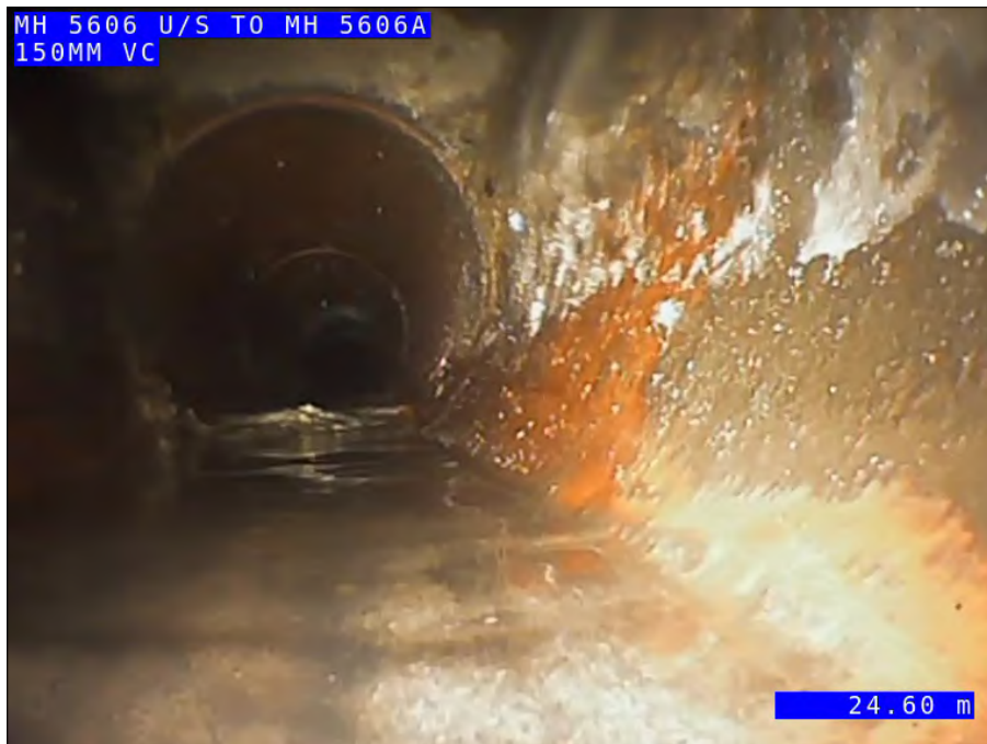
Photo: 6_6_17_A.jpg 24.6m, Finish node type, manhole reference number: 5606A
