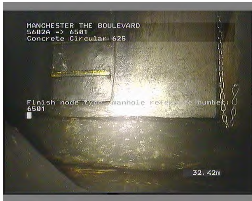
Photo: 4_4_13_A.JPG 32.41m, Finish node type, manhole reference number: 6501
