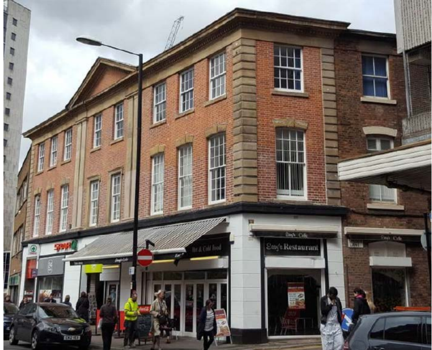
Figure 15: Reedham House, King Street West and Smithy Lane elevations, 2019
