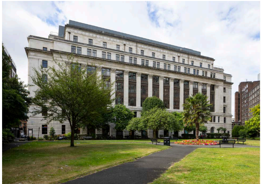
View 9: Looking south from Parsonage Gardens
