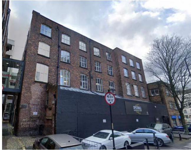
Figure 21: Existing western elevation of the listed building
