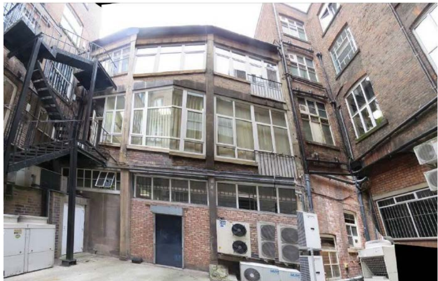
Figure 16: Rear elevation of Reedham House (photomontage, 2019) showing post-war rebuilding and additions
