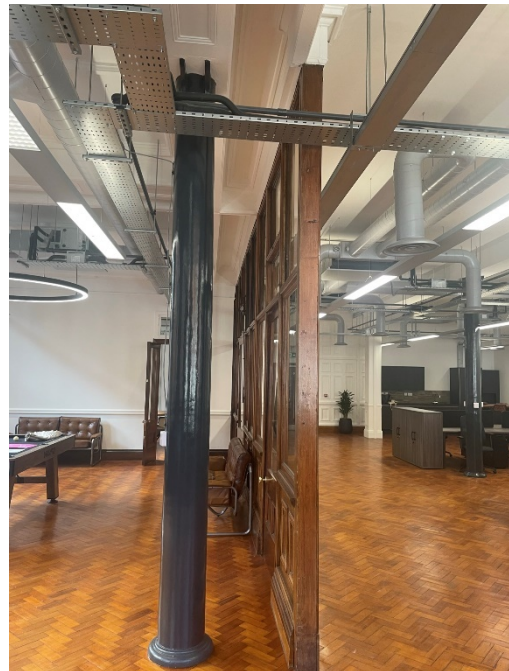
Figure 5: Showing original parquet flooring, end of timber screen and cast-iron column
