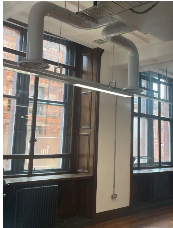
Figure 7: Original timber panelling to window reveals and below cills remain to the windows of the west (Dale Street) elevation
