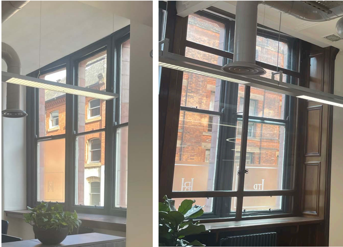
Figure 10: Examples of original sash windows with deep cills. Some windows appear to retain their original etched glass with the Howarth's logo
