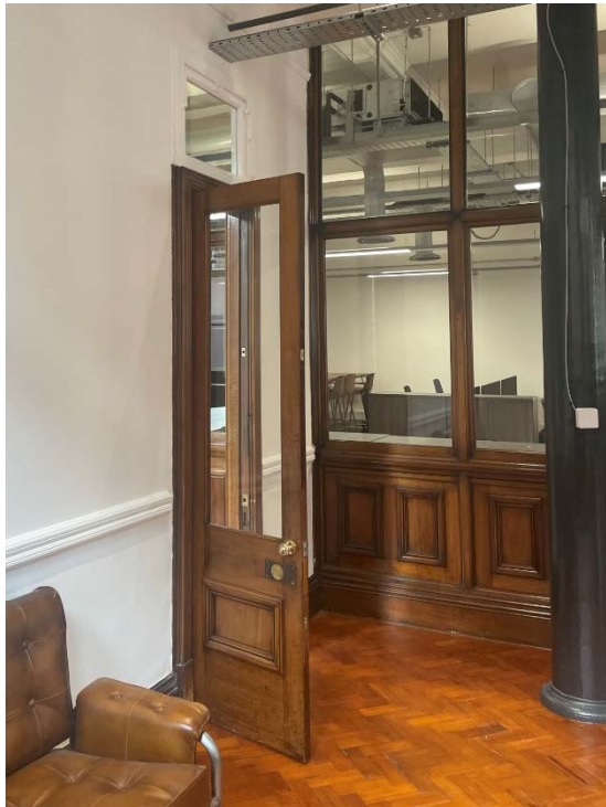
Figure 6: Original glazed timber panelled door, though the timber / glazed partition indicated on original plan has been replaced (or covered) with plaster finish
