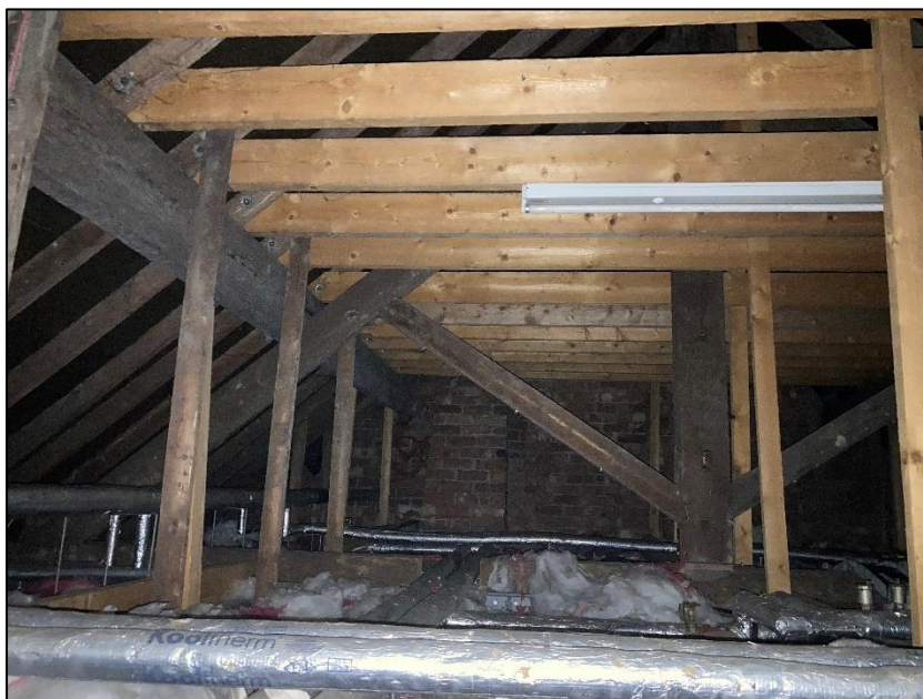
Photograph 37 showing the roof void
