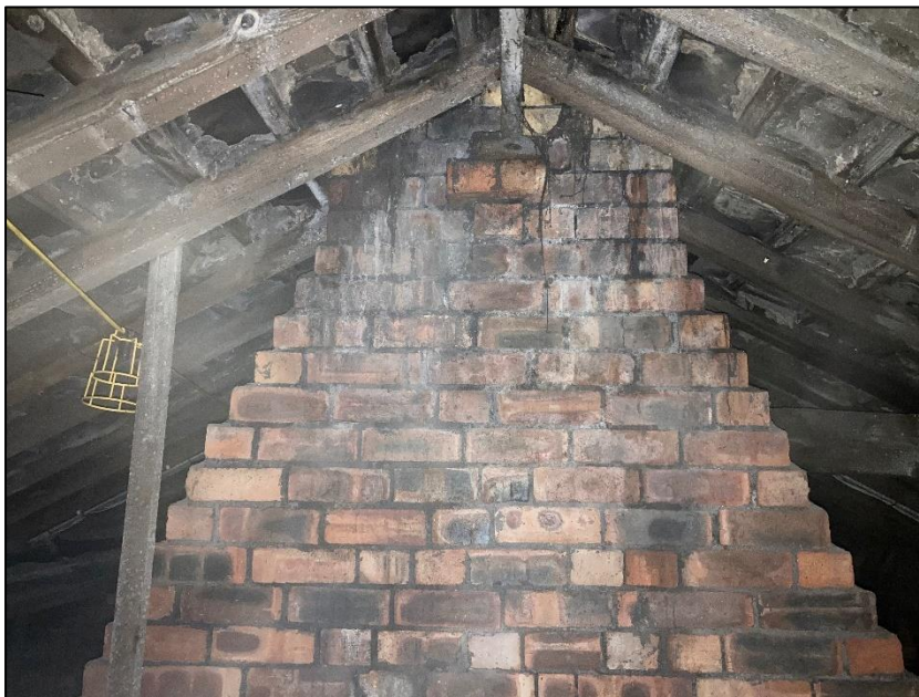
Photograph 24 showing some of the internal brickwork
