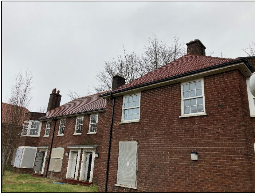
Photograph 33 showing the brickwork
