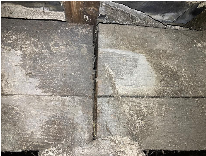
Photograph 22 showing the gap between roof timbers
