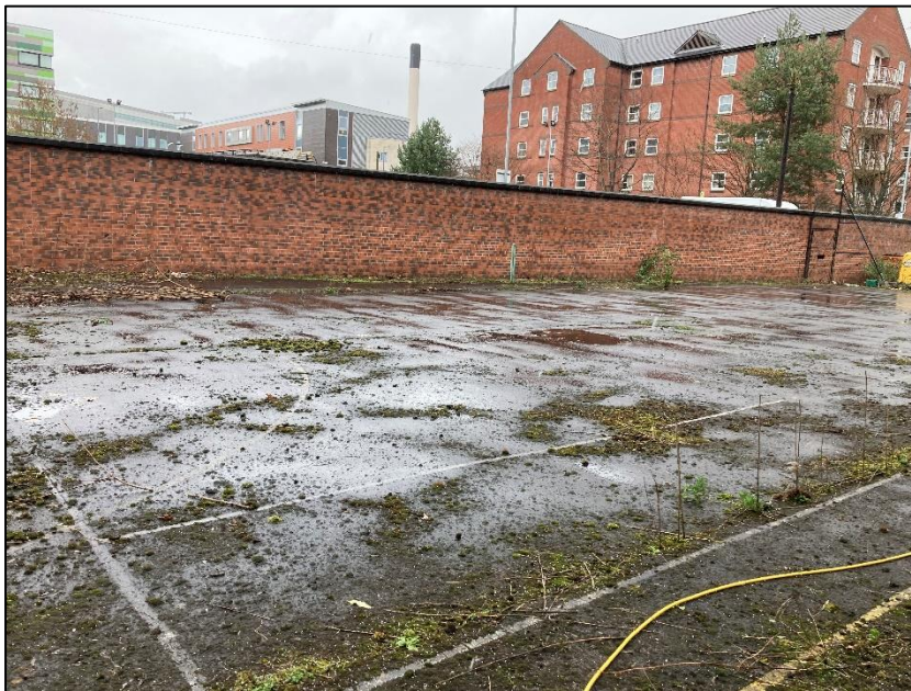
Photograph 1 showing the hardstanding
