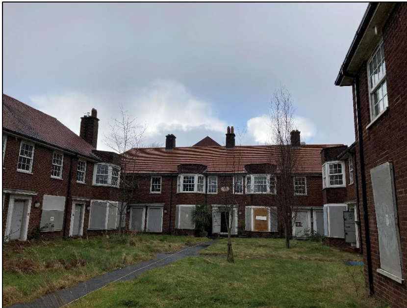
Photograph 32 showing Woodthorpe Hall
