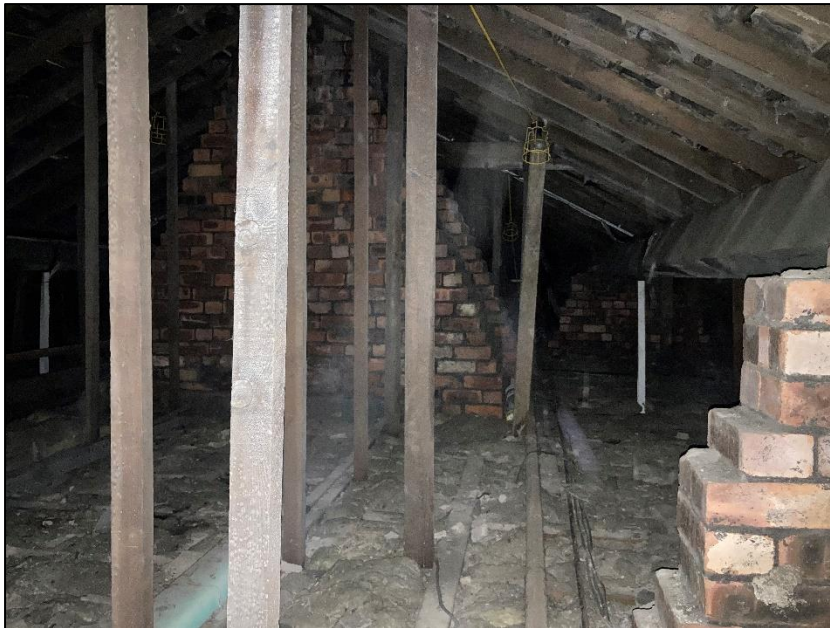
Photograph 20 showing the roof void in the western section of the building
