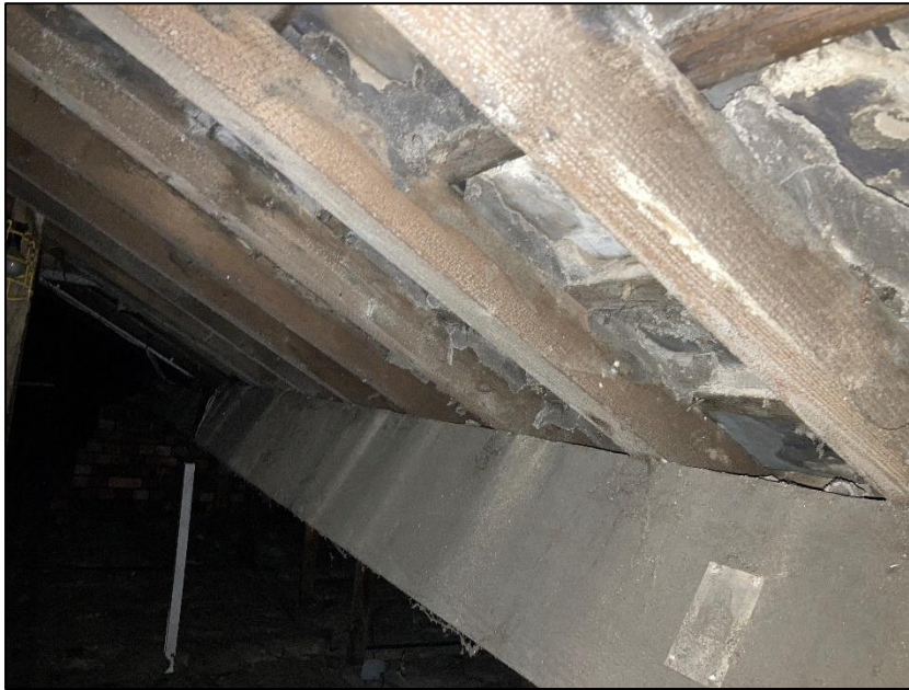
Photograph 21 showing the roof timbers
