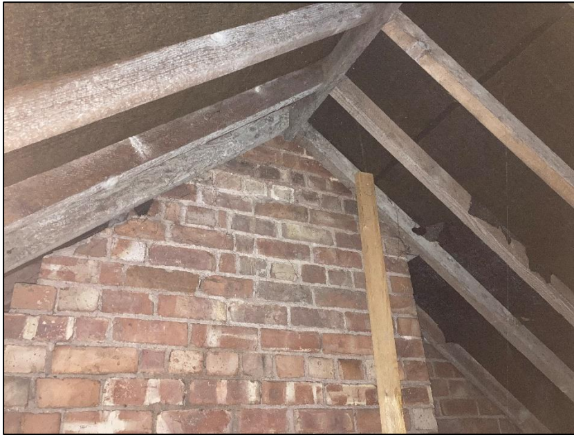
Photograph 39 showing the internal brickwork
