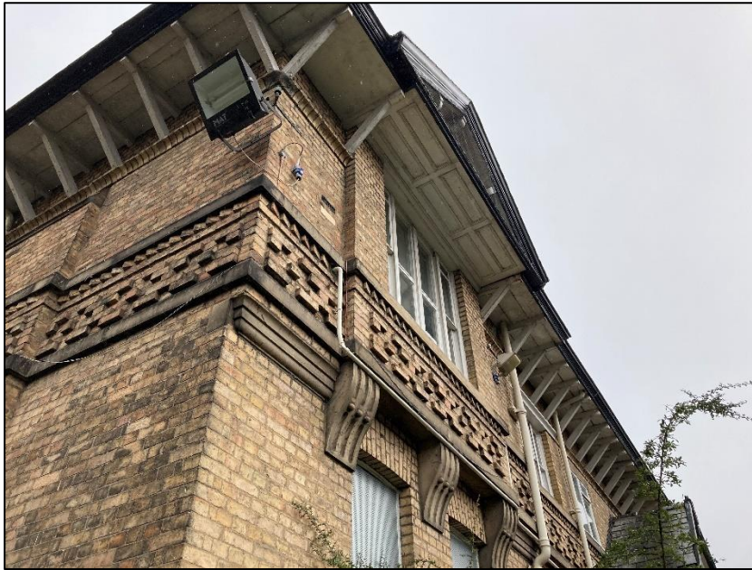
Photograph 17 showing the wooden soffits
