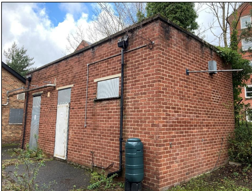
Photograph 46 showing the service building
