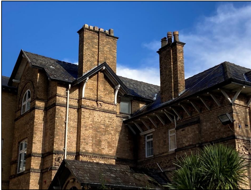
Photograph 13 showing the brickwork
