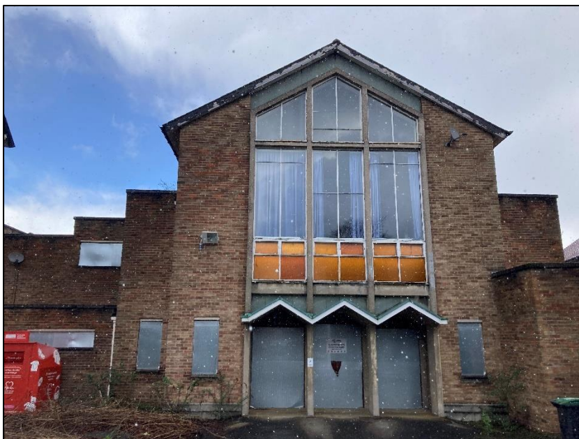
Photograph 26 showing the front facing elevation of The Chapel
