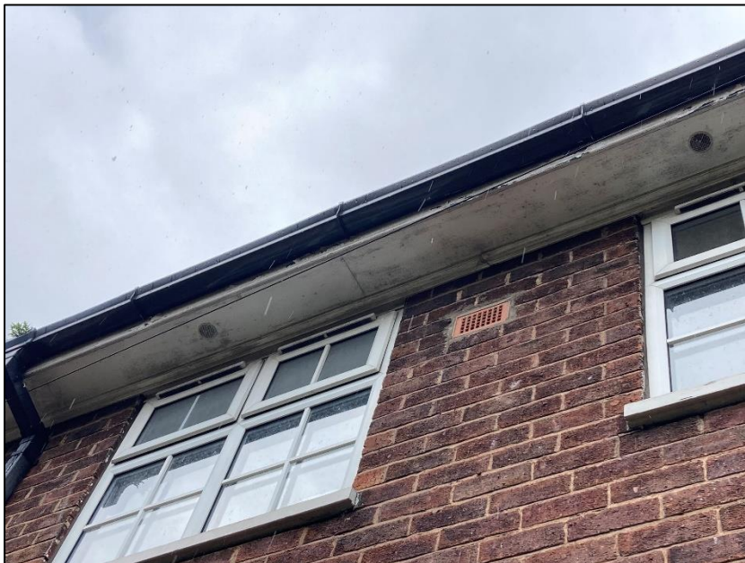
Photograph 36 showing the soffits
