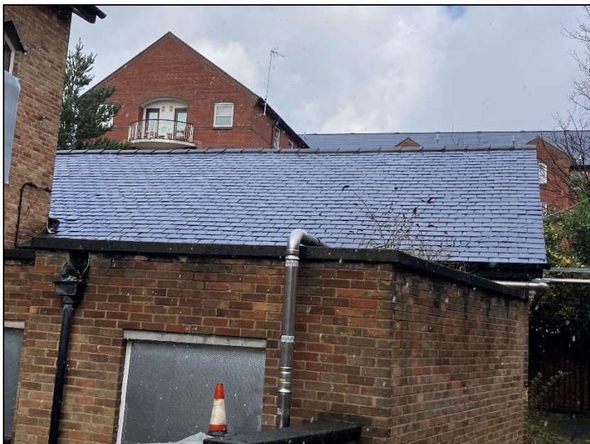
Photograph 28 showing a section of the Chapel roof looking north
