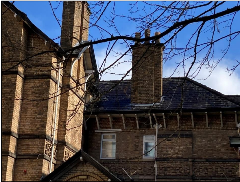
Photograph 15 showing part of the roof of St Gabriel's Hall
