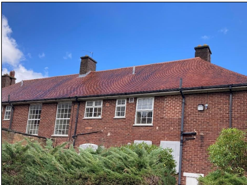
Photograph 34 showing the roof of Woodthorpe Hall
