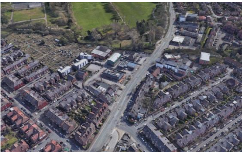
Approach to site from High Lane
