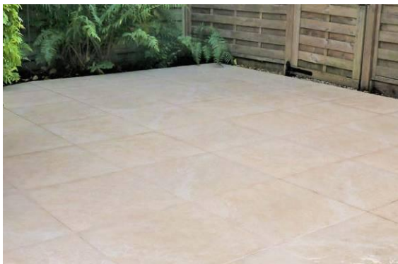
Typical terrace Paving, Ivory colour.
