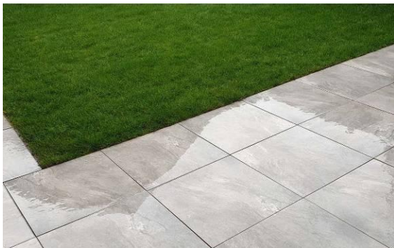
Typical Courtyard Paving, Valencia Grey colour.
