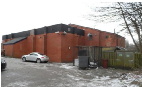
Existing building rear view
