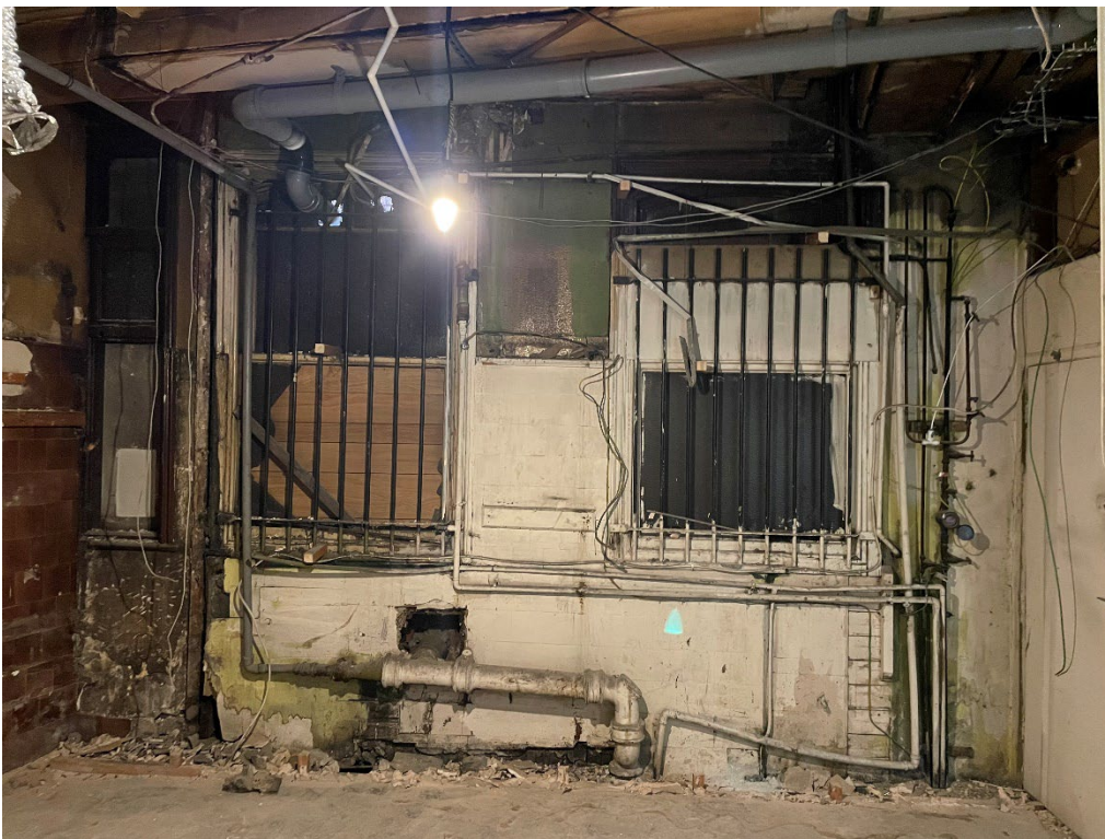
Windows revealed after removing drylining partitioning
