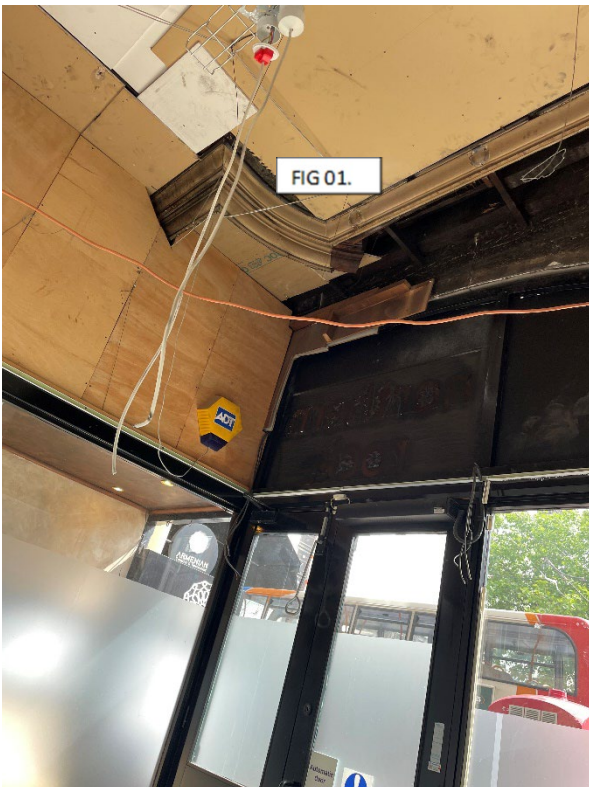
FIG 01 shows aspects of original coving are around perimeter ceiling.
