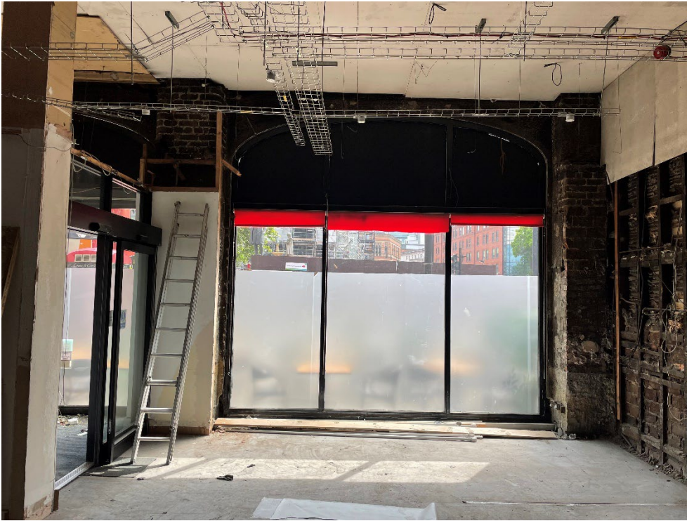
Front window strip-out reveals three centred arches.
