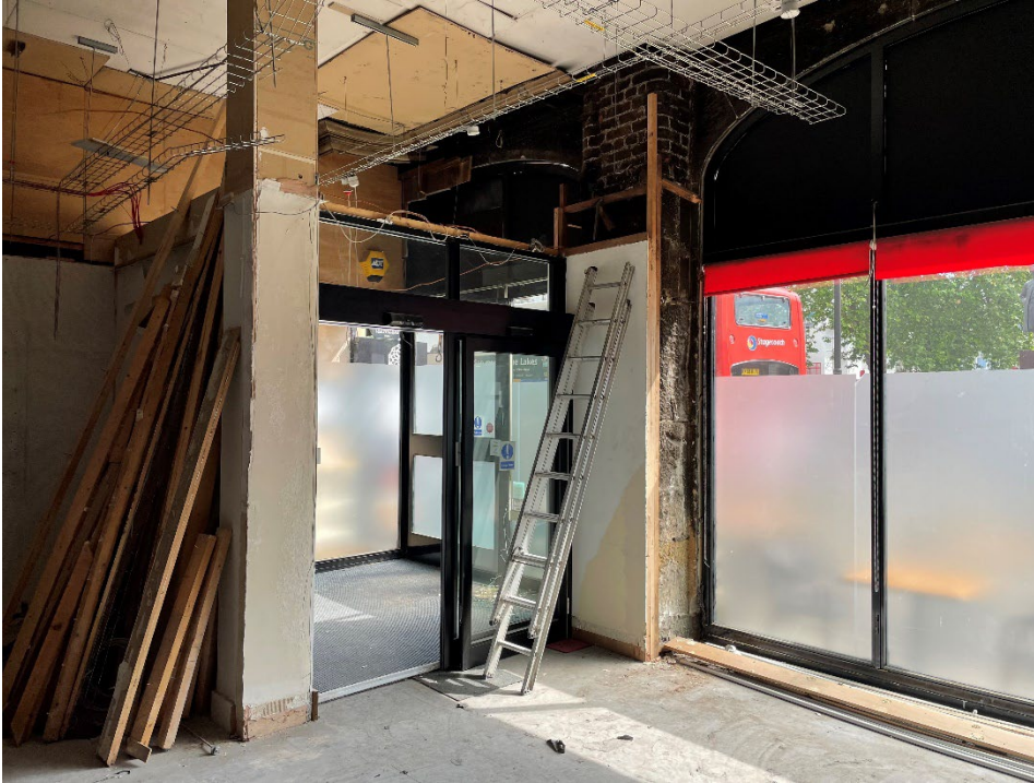
Picture shows main entrance with existing suspended ceiling removed and reveals original height ceiling
