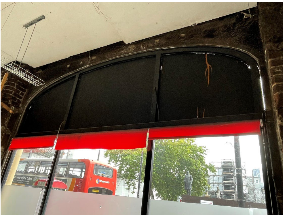
Original stonework cladding around arch, with exposed brickwork.
