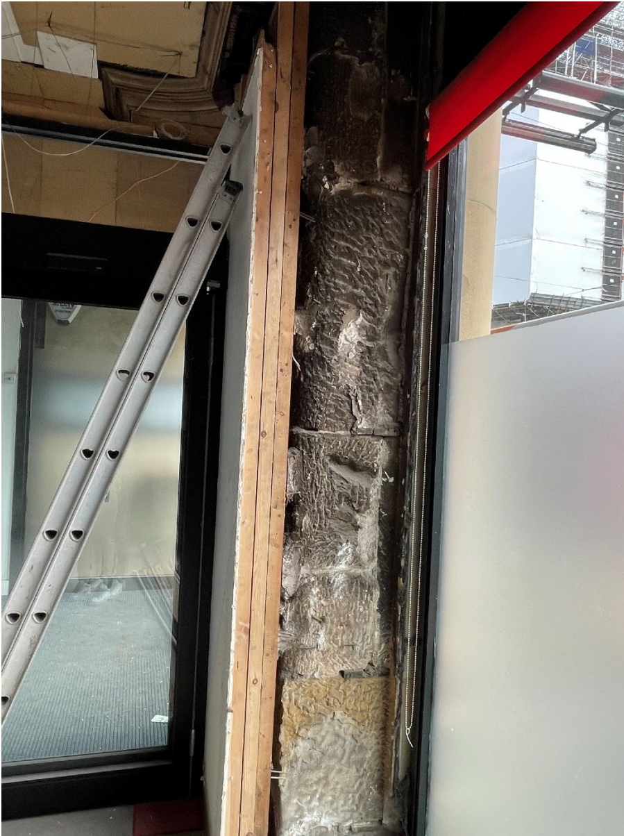
Existing stonework around window reveal.
