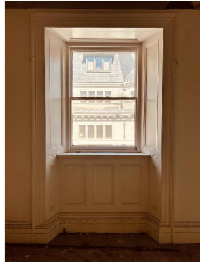
03 THIRD FLOOR EXISTING WINDOW PHOTO 573 SCALE - N/A PHOTOGRAPH
