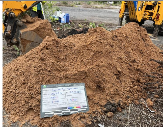
Trial Pit 1: Overview of excavated soils
