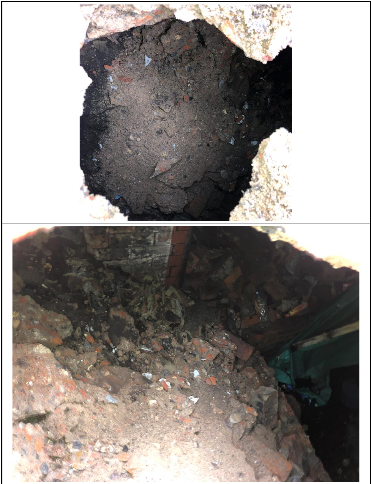
Figure 5: Photographs of Basement Encountered
