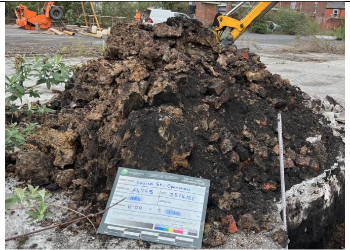
Trial Pit 5: Overview of excavated soils
