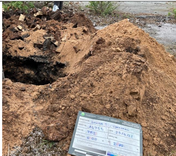
Trial Pit 2: Overview of excavated soils
