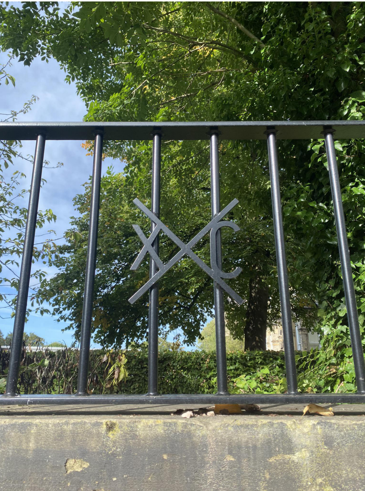
Existing photograph of railing details. Proposed new railing topping to be of similar appearance and height.
