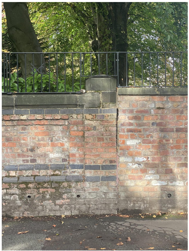
Existing photograph of railing details. Proposed new railing topping to be of similar appearance and height to brick post.
