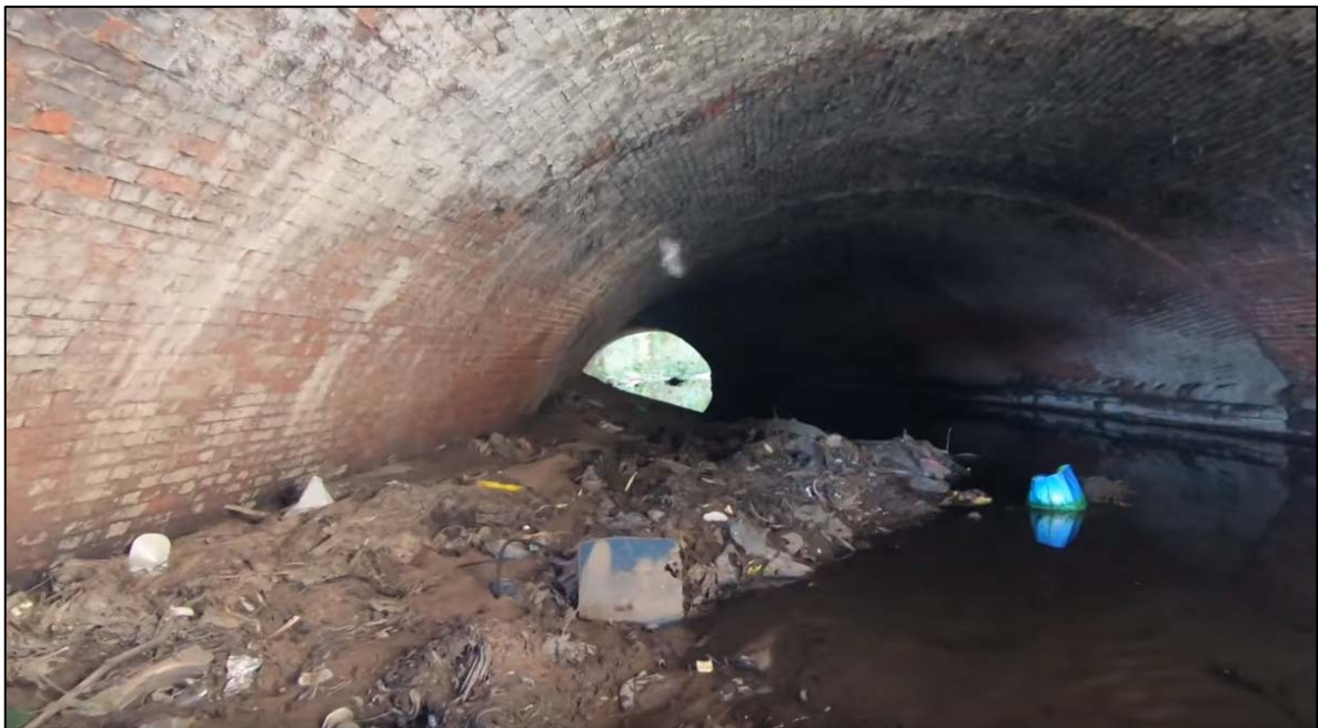
Plate 8 Culvert B26 interior looking downstream, showing brick-built arched structure (Martin Zero 2018)
