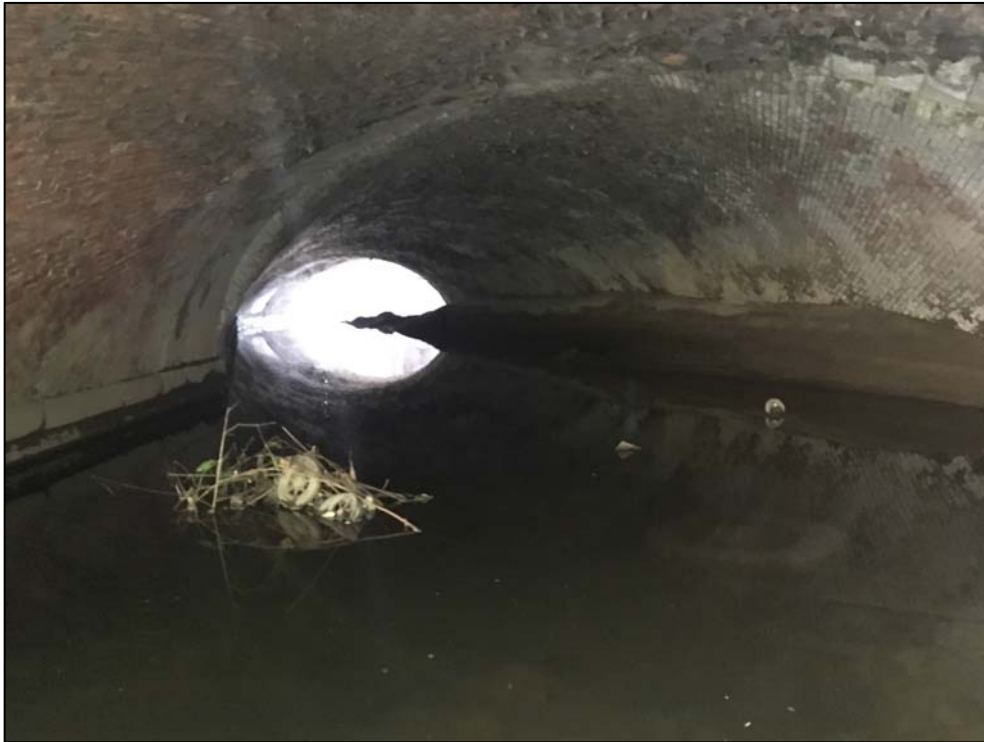
Plate 9 Culvert B26 looking upstream. Brickwork largely intact with few crevices (July 2017)
