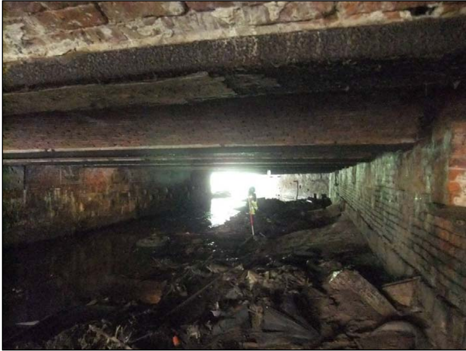
Plate 3 Culvert B24 box section culvert over River Medlock
