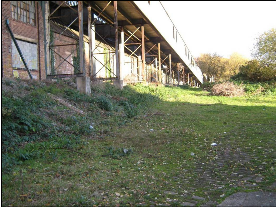
Plate 1 Southern side of B2 – roost entrance identified towards end of ramp during earlier survey work undertaken by other consultants during 2014
