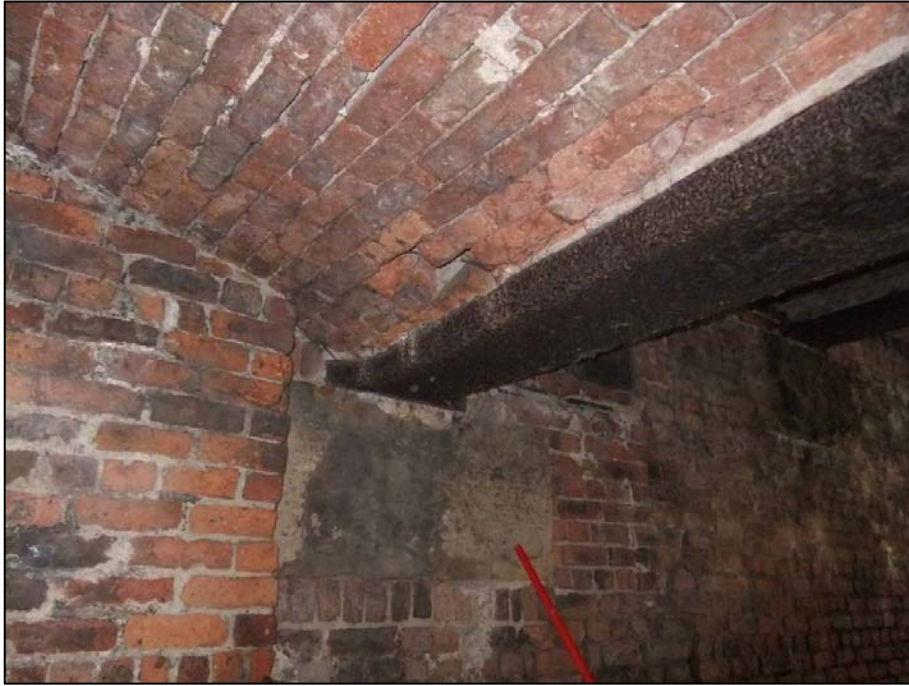
Plate 5 Culvert B24 wall of mixed materials
