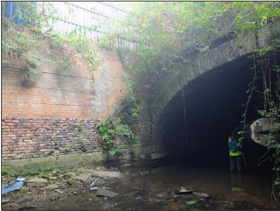
Plate 7 Culvert B26 downstream end, left bank looking upstream showing stone lintel and brick head and sidewalls
