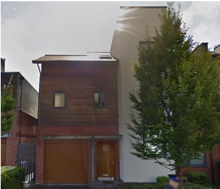
Photograph 1 Front elevation as viewed from Clearwater Drive, Source: www.google.com/maps accessed 05.10.2022
