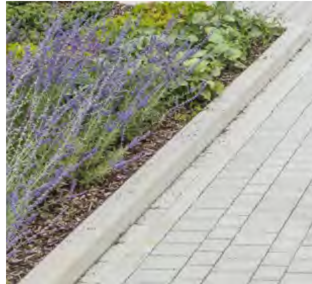
Exposed aggregate kerb upstands to planting areas
