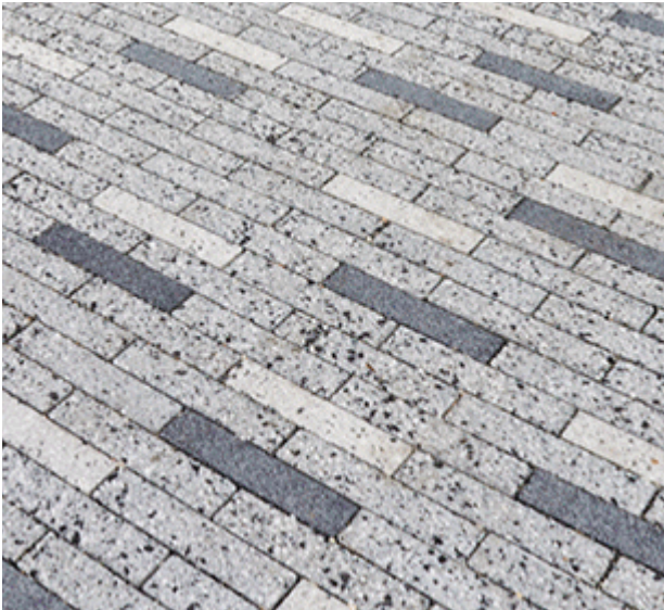
High quality exposed aggregate concrete block paving
