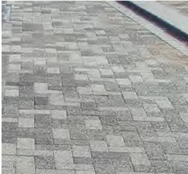
Block paved vehicle parking layby
