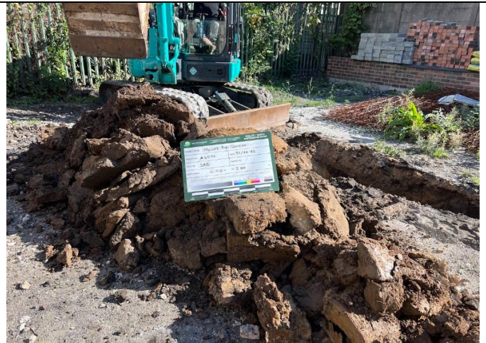
Soakaway Pit 2: Overview of excavated soils
