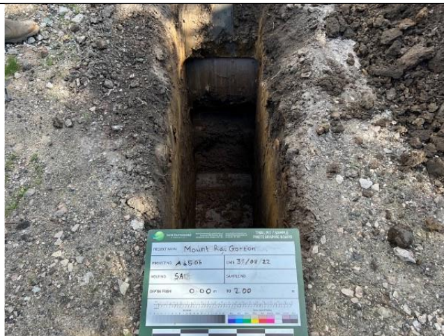
Soakaway Pit 1: Overview of excavation
