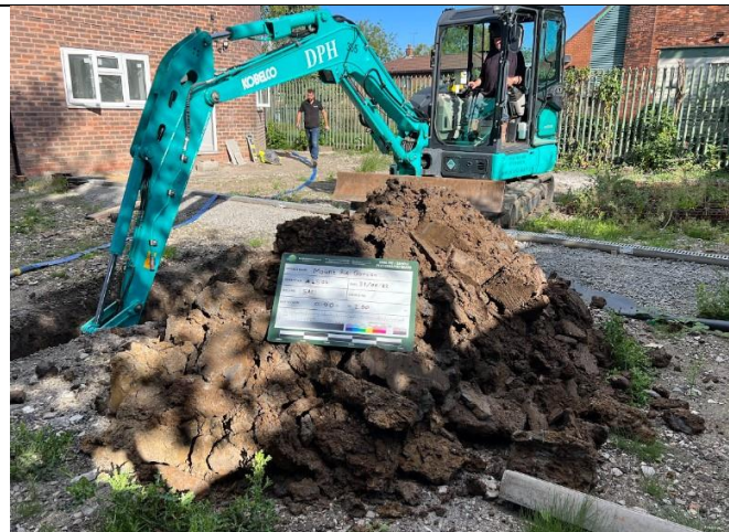
Soakaway Pit 1: Overview of excavated soils
