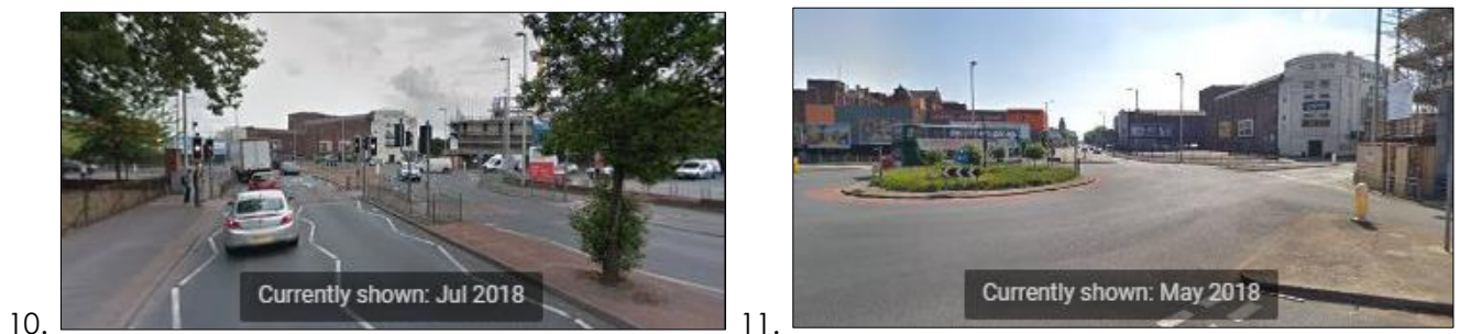
Figures 10 – 11. Longer range views of the site and proposed display would be dominated by the massing of the theatre building, the prominence of the façade, and the existing advertising displays adjacent to the site.
