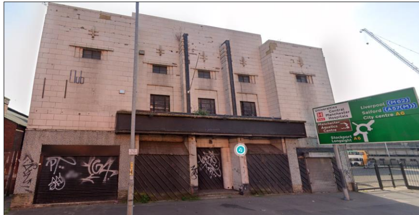
6. Figure 6. The Apollo theatre art deco façade facing Hyde Road
