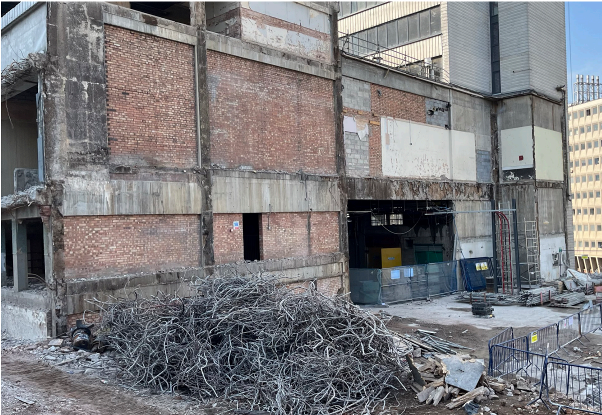
View from Deansgate to future service yard entrance
