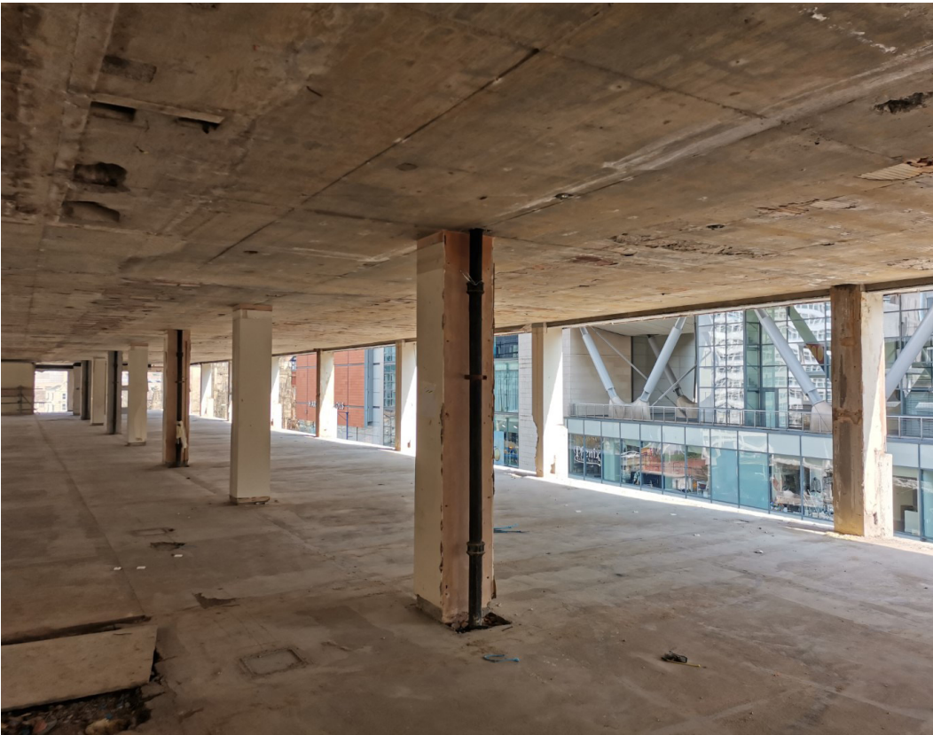
Existing structural frame
