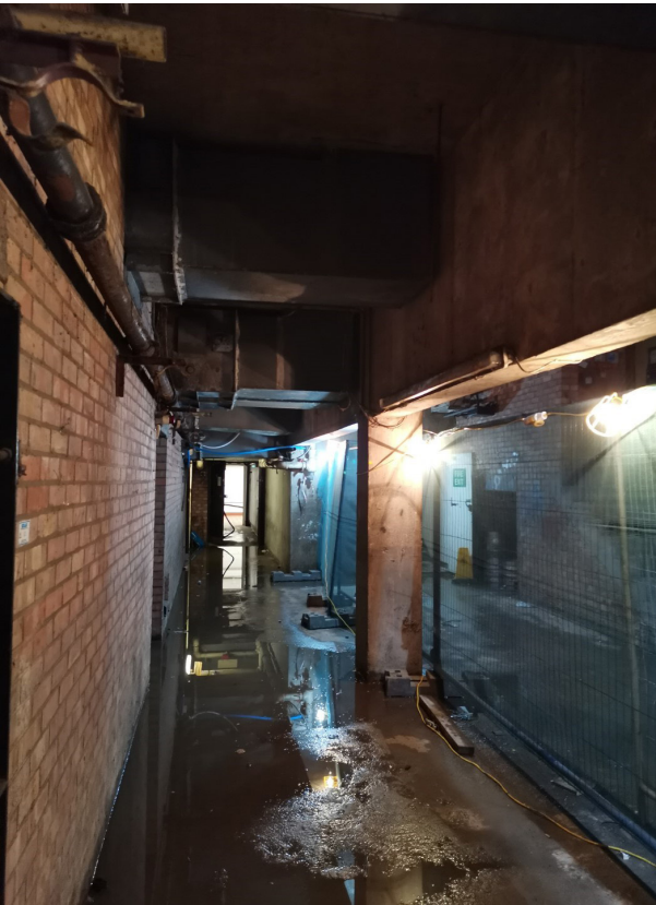
Internal view of Service Yard
