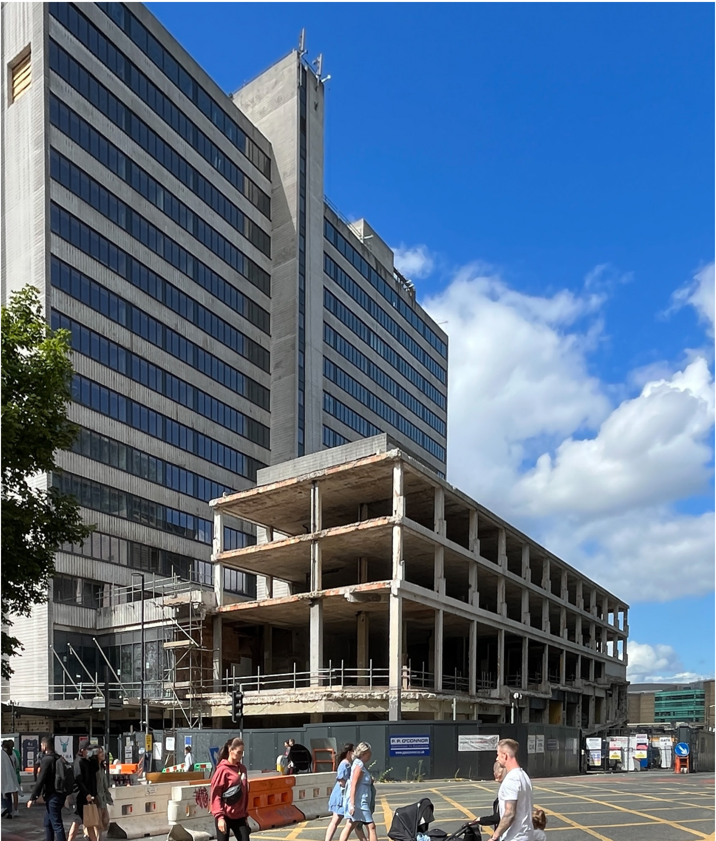
Existing Premier House looking north-west along Deansgate/ Blackfriars Street
