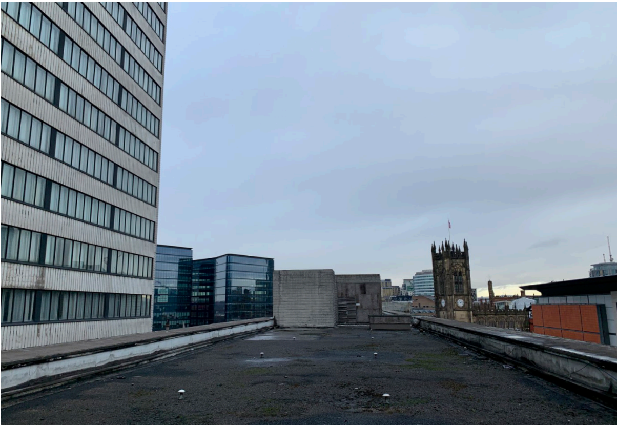
Existing roof and circulation shafts
