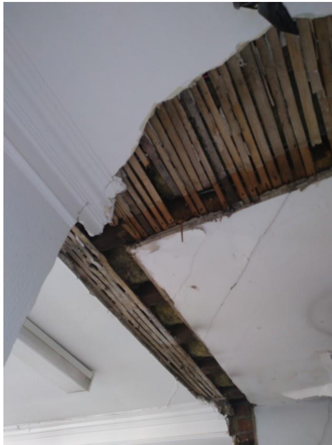
Figure 2: Ceiling on First floor
