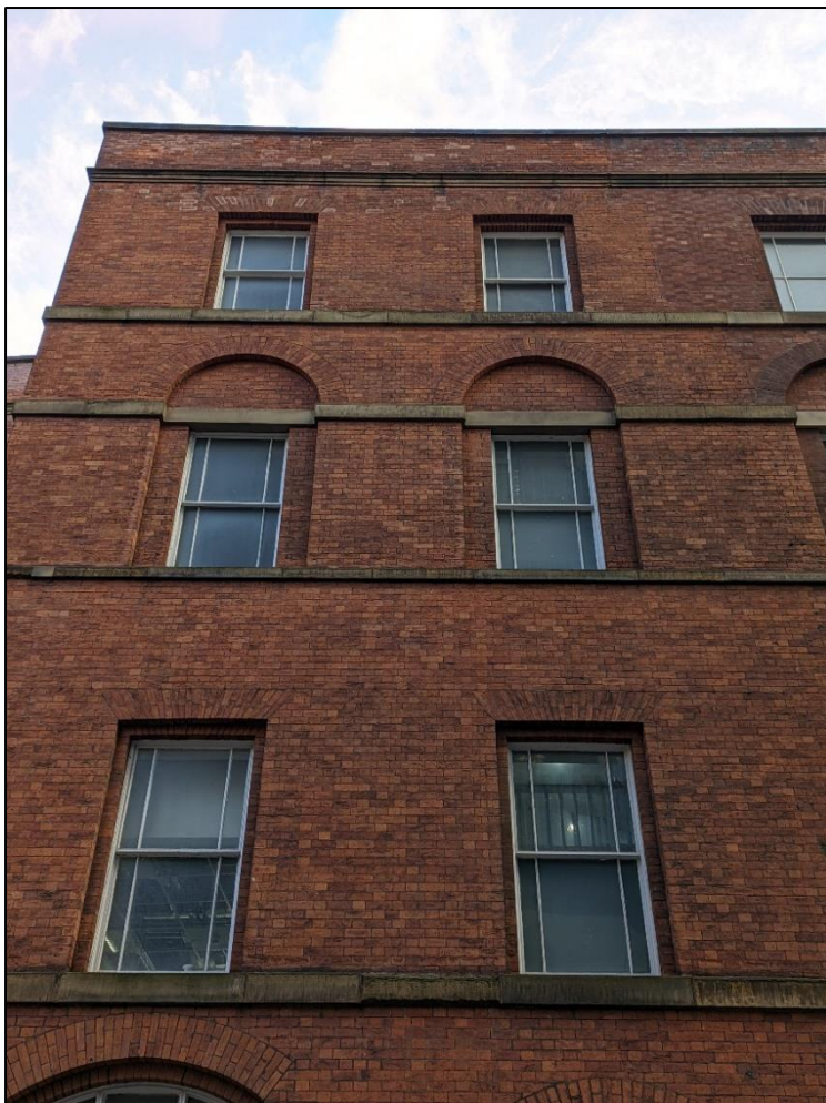
Plate 24: Upper floor windows in bays 5 and 6
