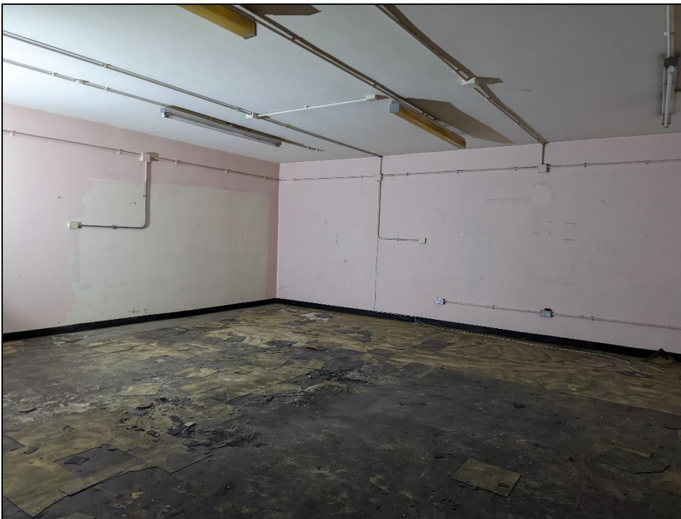
Plate 109: Eastern end of room shown above
