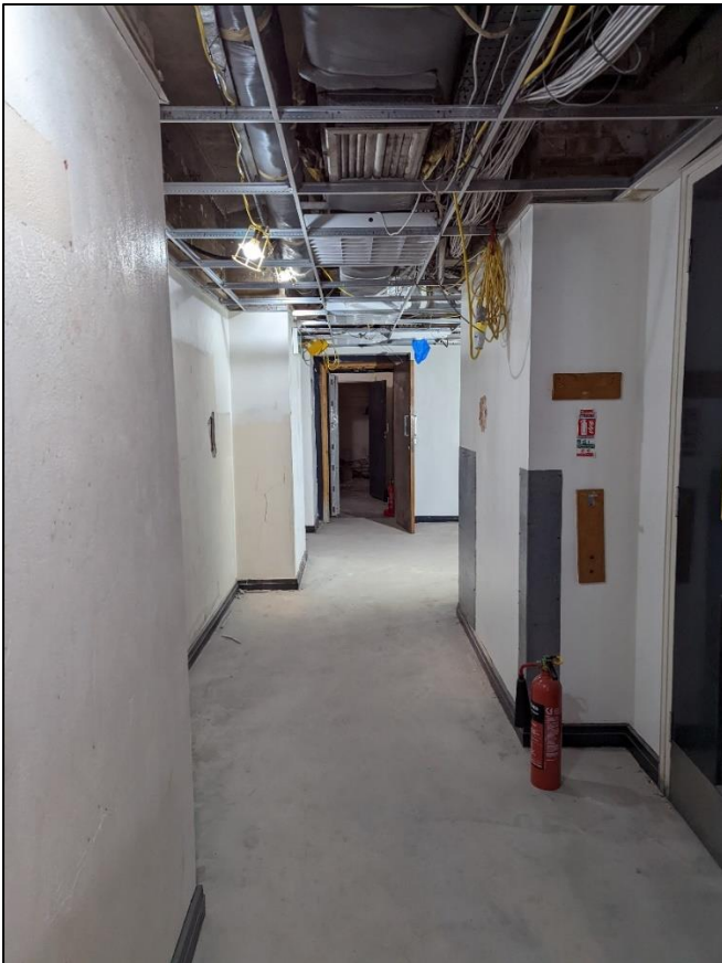
Plate 101: Corridor into vault area
