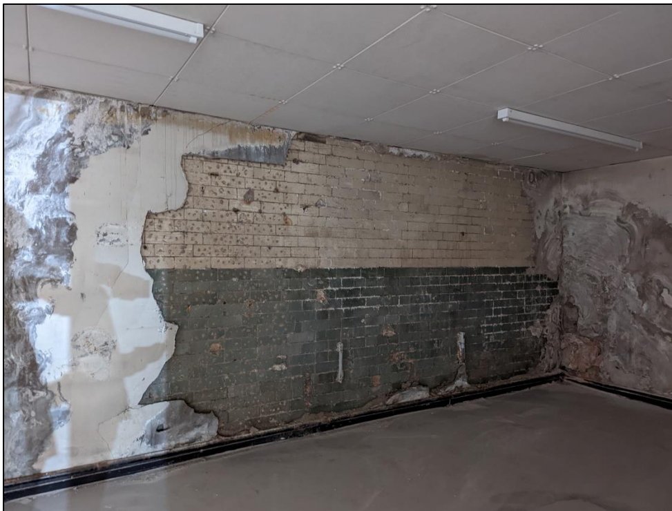
Plate 115: Glazed brick behind plasterboard in room to southeast corner of extension
