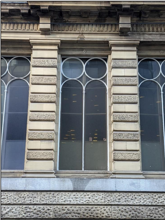
Plate 10: Ground and first floor window detail
