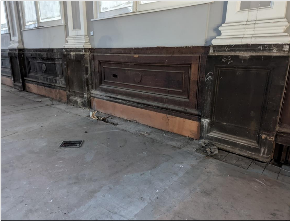
Plate 33: Panelling detail on timber at base of wall and base of columns
