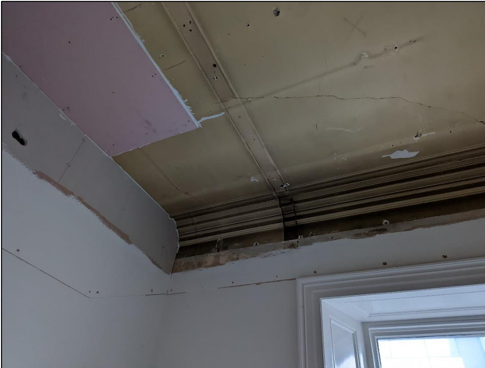
Plate 88: Ceiling detail of inserted office, showing cornice
