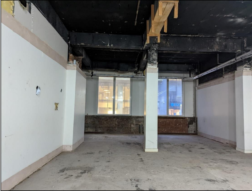
Plate 27: Southern Room showing windows to Mosley Street
