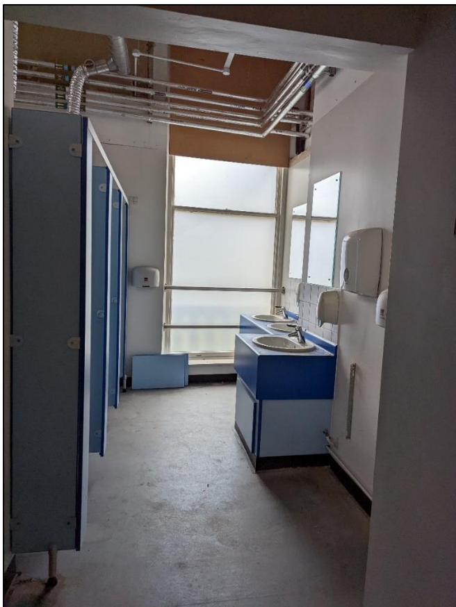
Plate 71: WC to west side of original building
