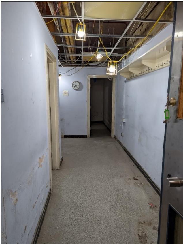
Plate 99: Corridor into rooms below arched wall area
