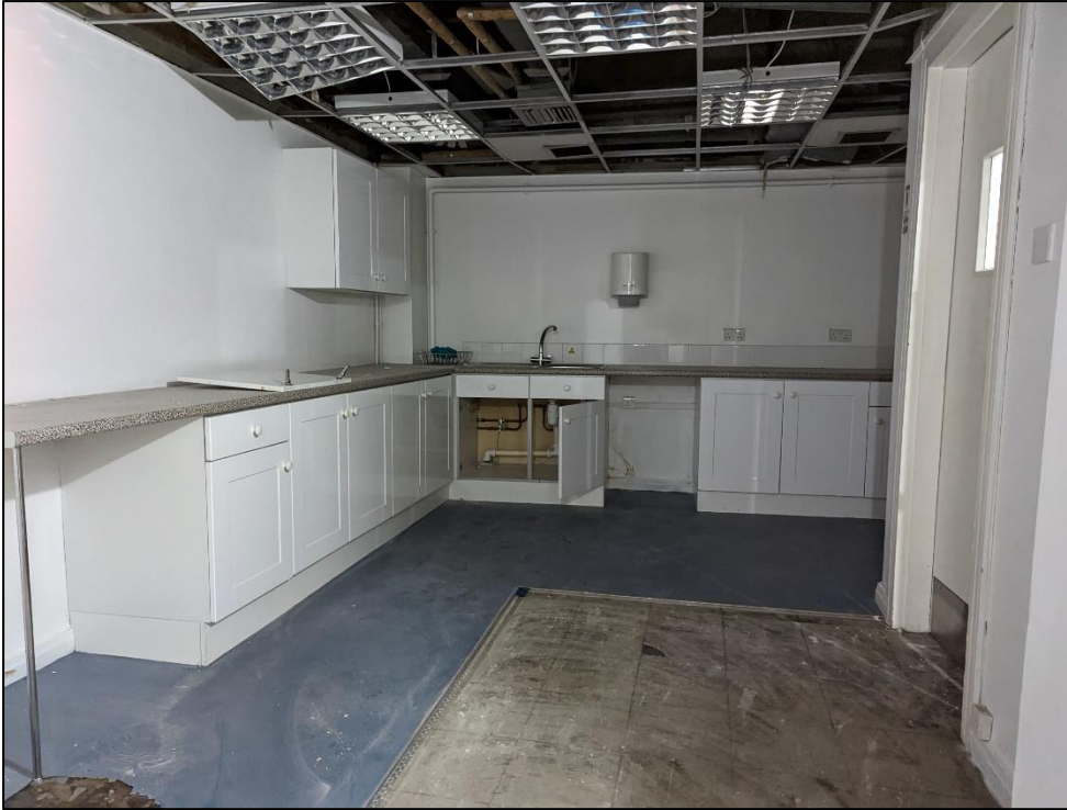
Plate 116: Inserted kitchen to southwest end of extension
