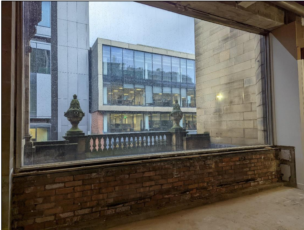
Plate 56: Recessed second floor to bay 5 showing large window
