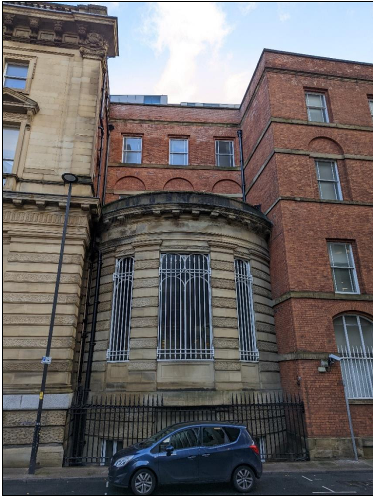
Plate 19: Bays 2 – 4 with rounded face and recessed brick section above
