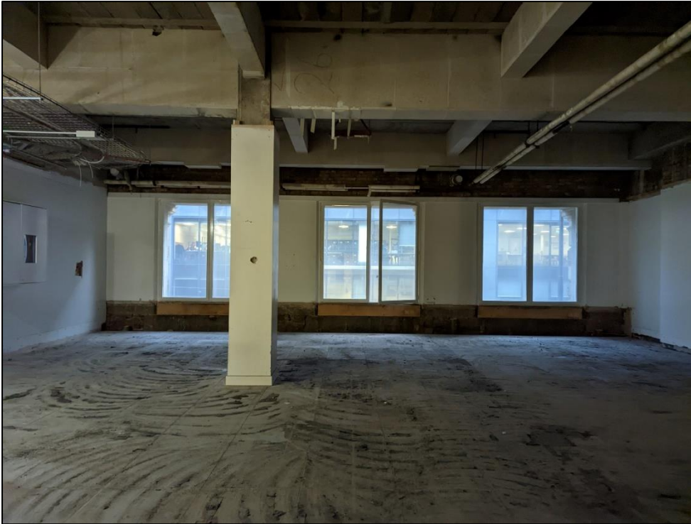
Plate 45: Southern room of extension facing Mosley Street
