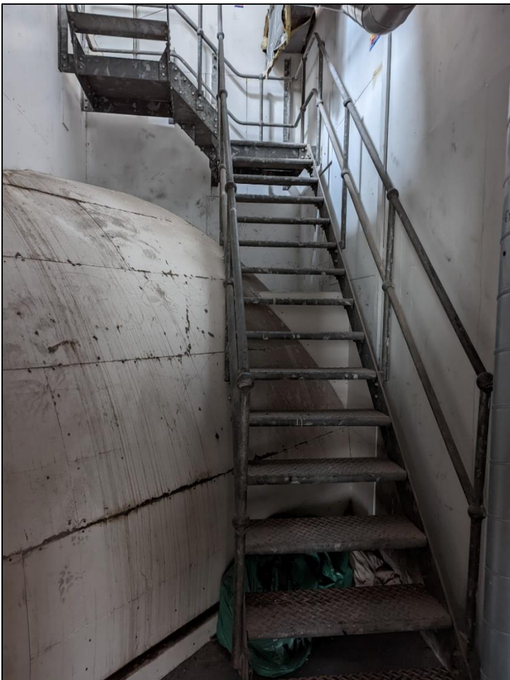
Plate 93: Metal staircase to roof access
