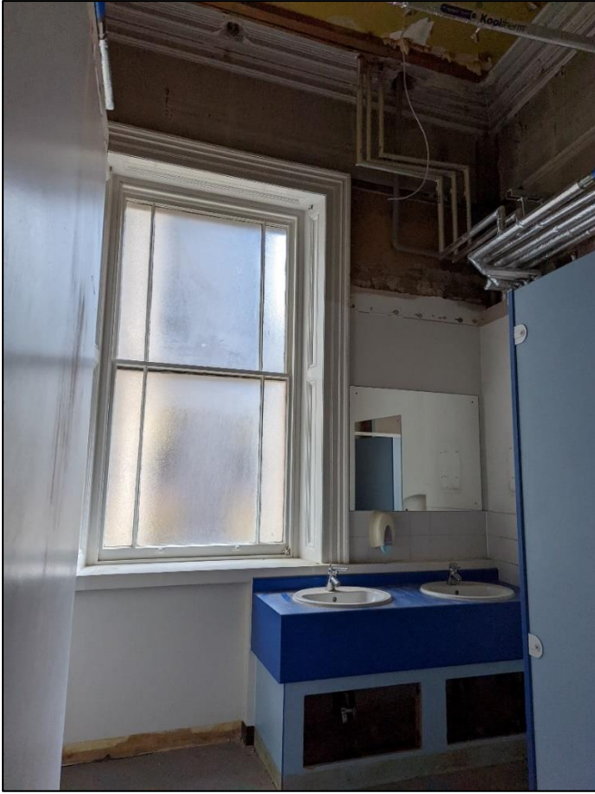
Plate 74: WC off corridor above showing cornice
