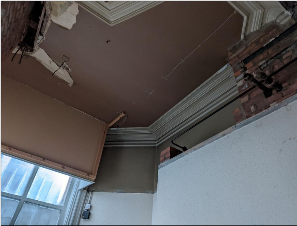
Plate 41: As above showing cornice
