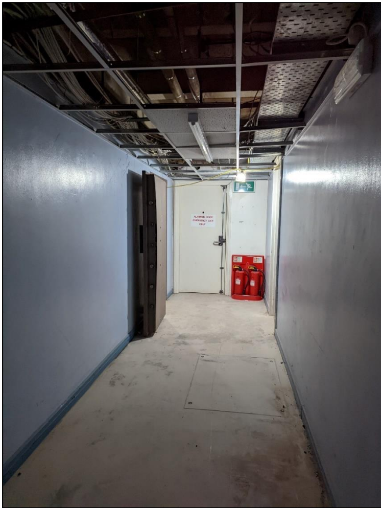
Plate 114: Corridor to west end of extension
