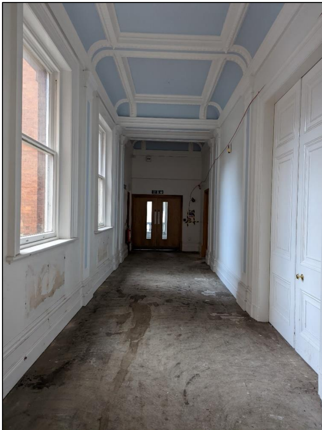
Plate 70: General shot of corridor looking north
