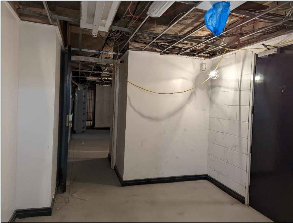
Plate 102: Northern vault area of original building
