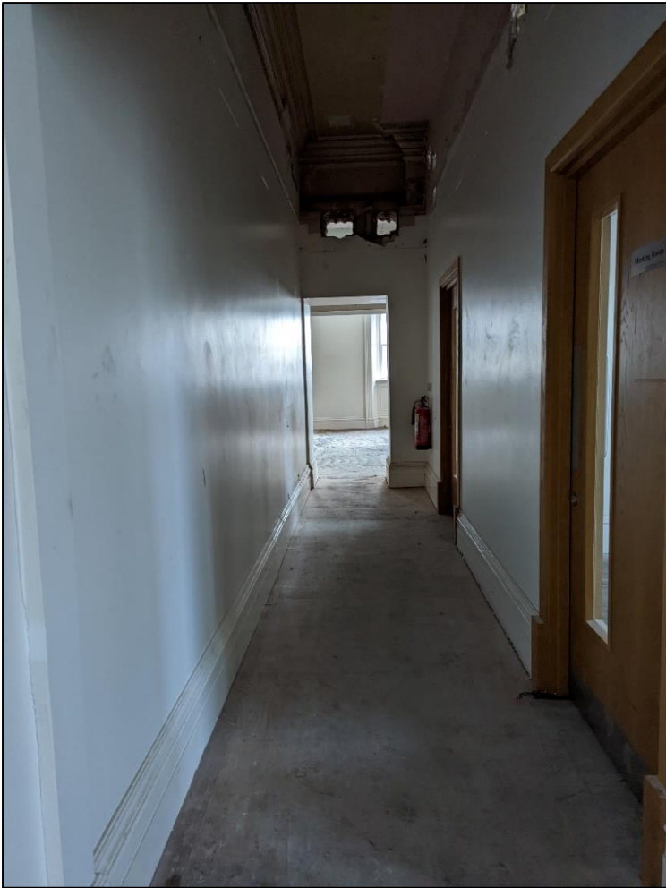
Plate 86: Corridor linking inserted offices to east side
