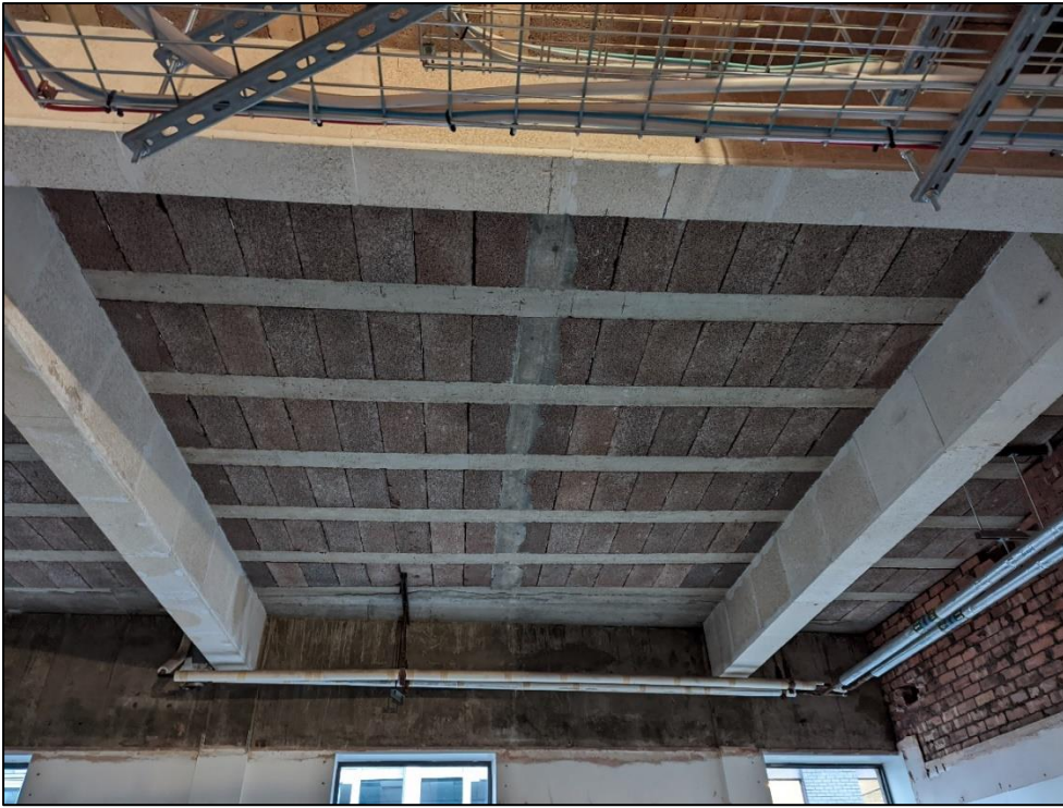
Plate 53: Detail of concrete ceiling construction throughout extension
