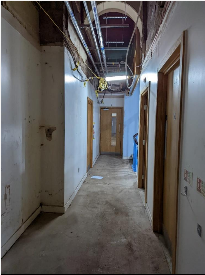
Plate 72: Continuation of corridor shown above to the south, into extension
