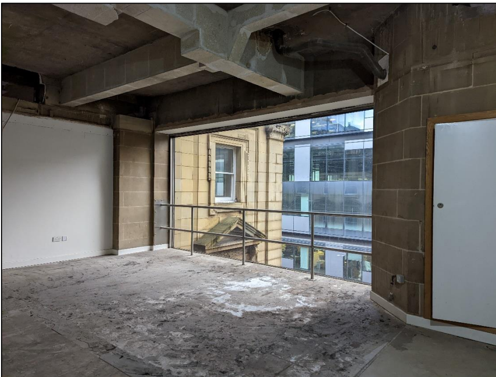
Plate 79: Room above bay 5 to Mosley Street showing large window
