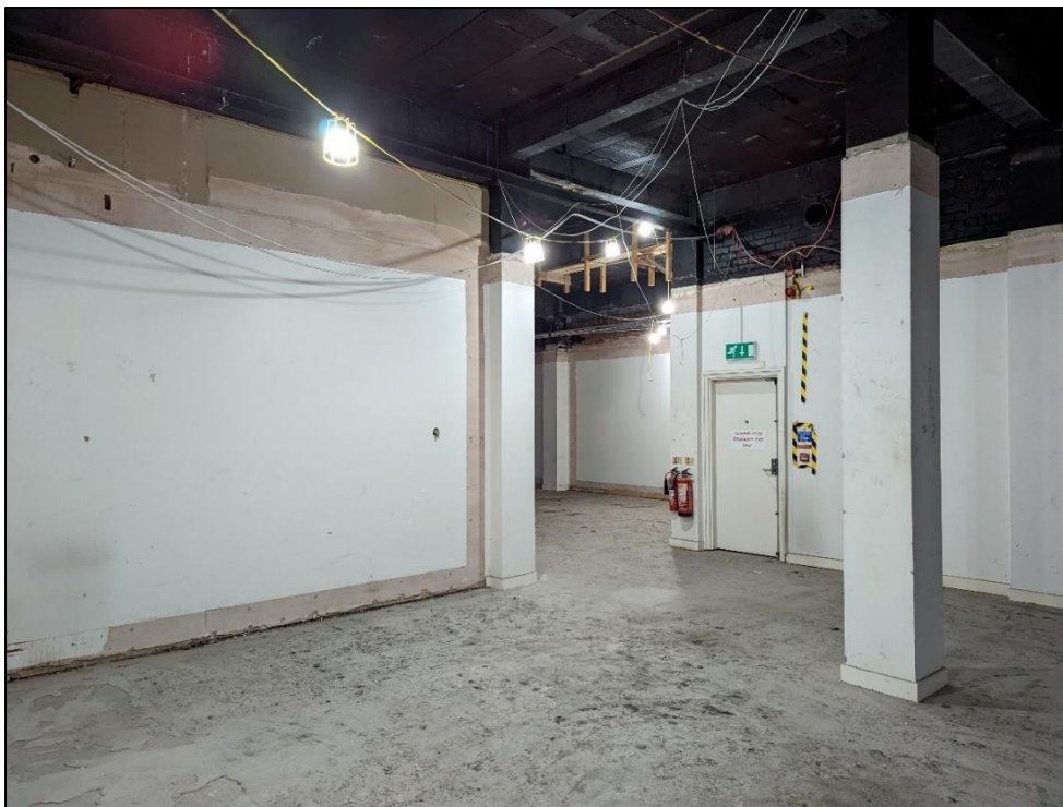
Plate 44: Large room towards southern end of extension
