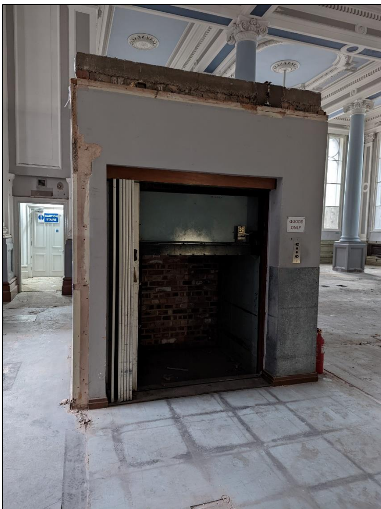
Plate 38: Goods lift to basement
