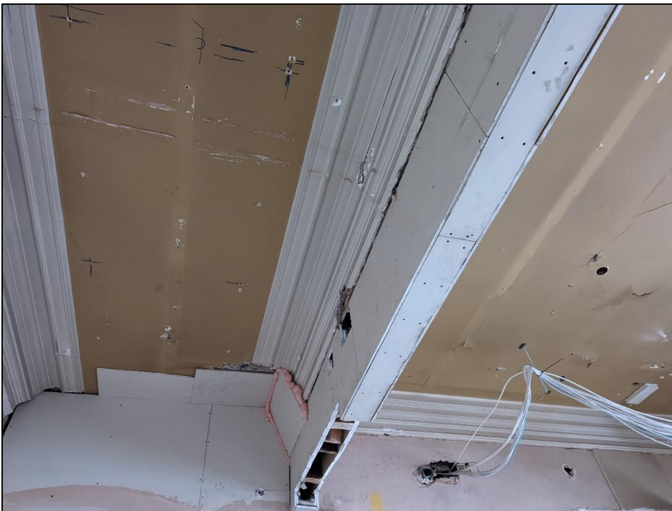
Plate 91: Ceiling detail of room above showing cornice indicating former corridor
