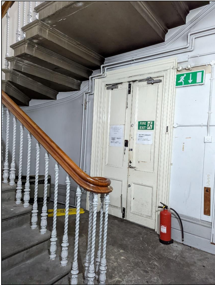
Plate 39: Staircase in northwest corner of building
