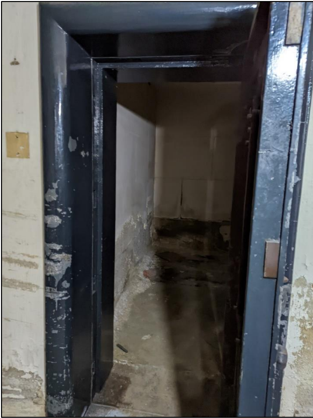
Plate 106: Further vault door
