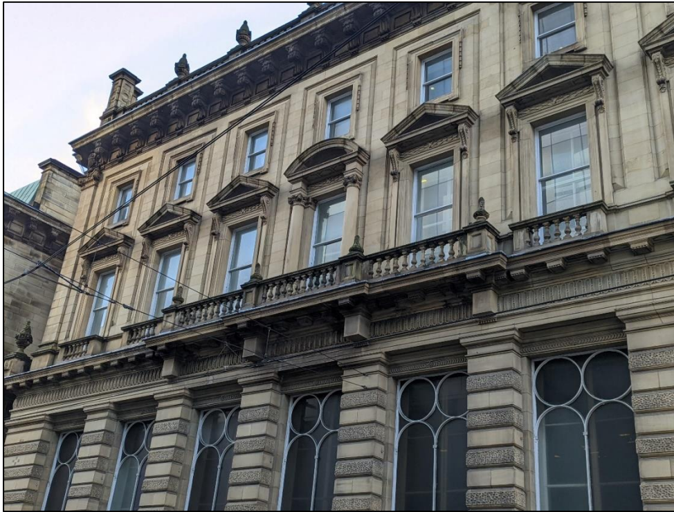
Plate 13: Second floor windows showing differing central window
