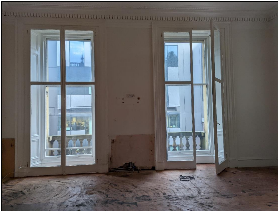
Plate 58: Windows to Mosley Steet in south end of original building
