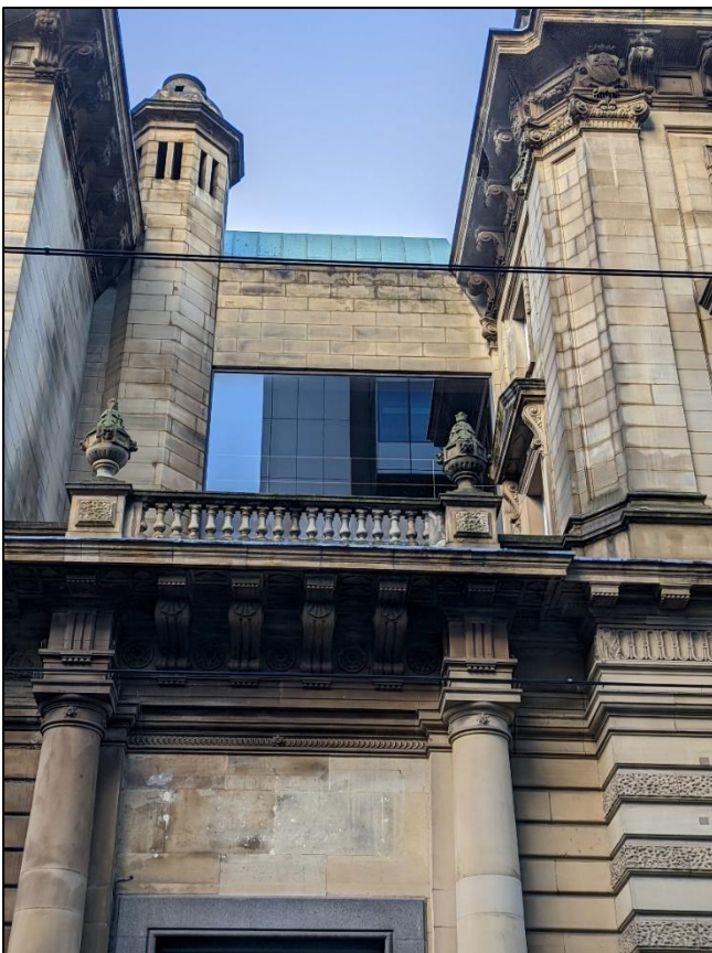
Plate 8: Recessed second and third floors at bay 5
