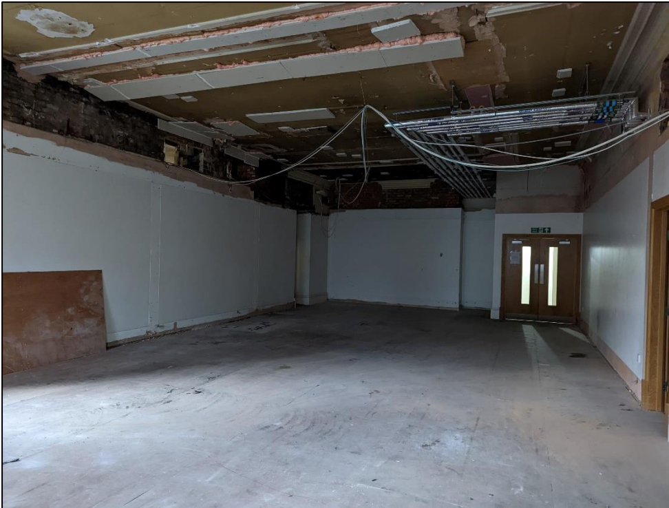
Plate 84: General shot of room shown above
