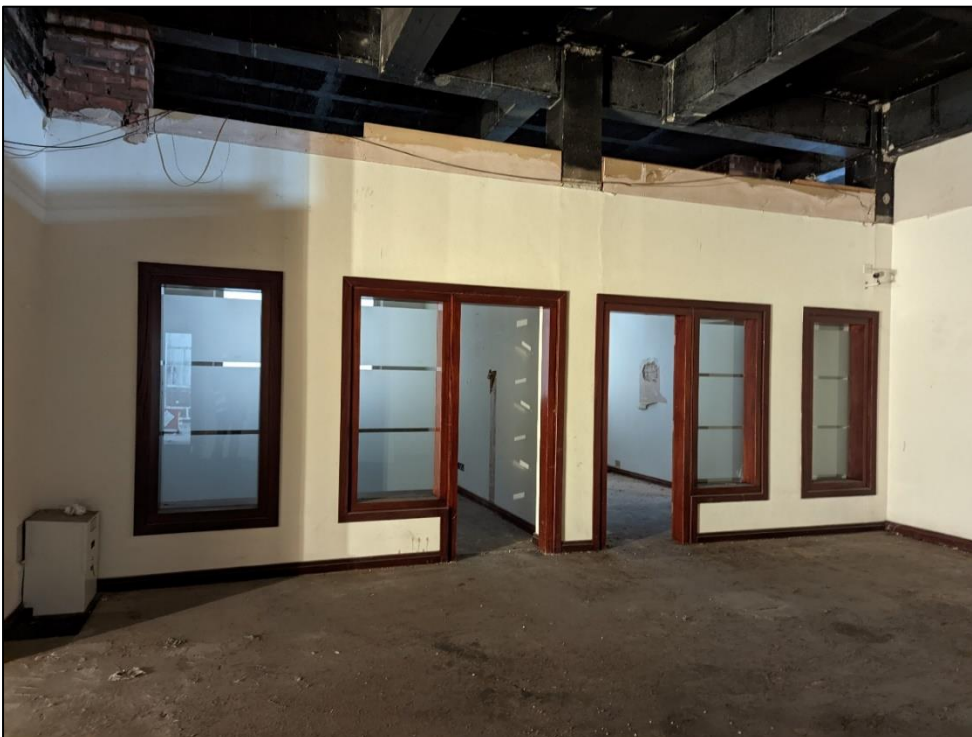
Plate 28: Room to the north of the above, showing offices close to lifts
