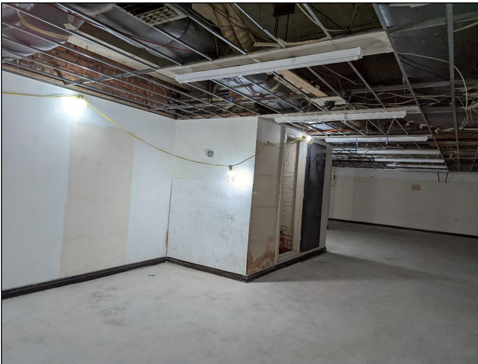
Plate 111: Room to northeast corner of extension
