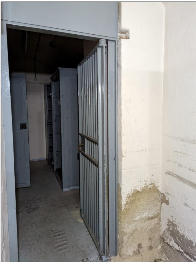
Plate 105: As above showing vault door
