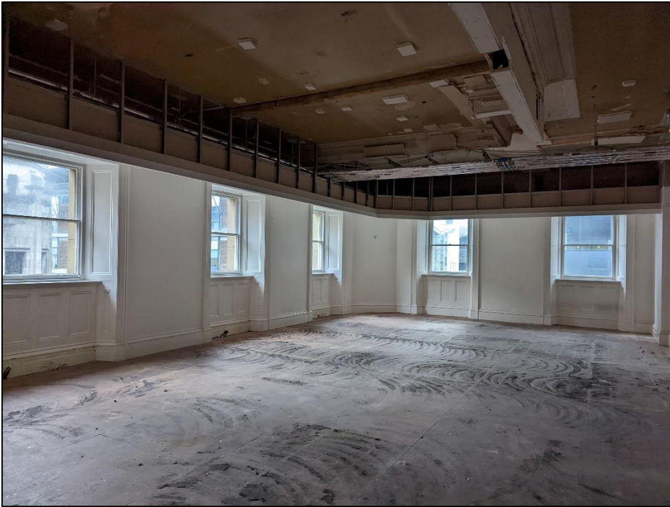
Plate 92: General shot of room shown above
