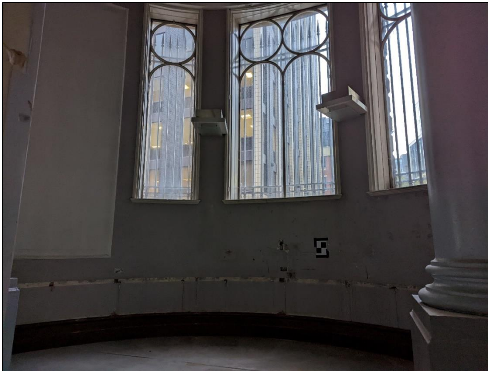
Plate 37: Curved wall to West Mosley Street
