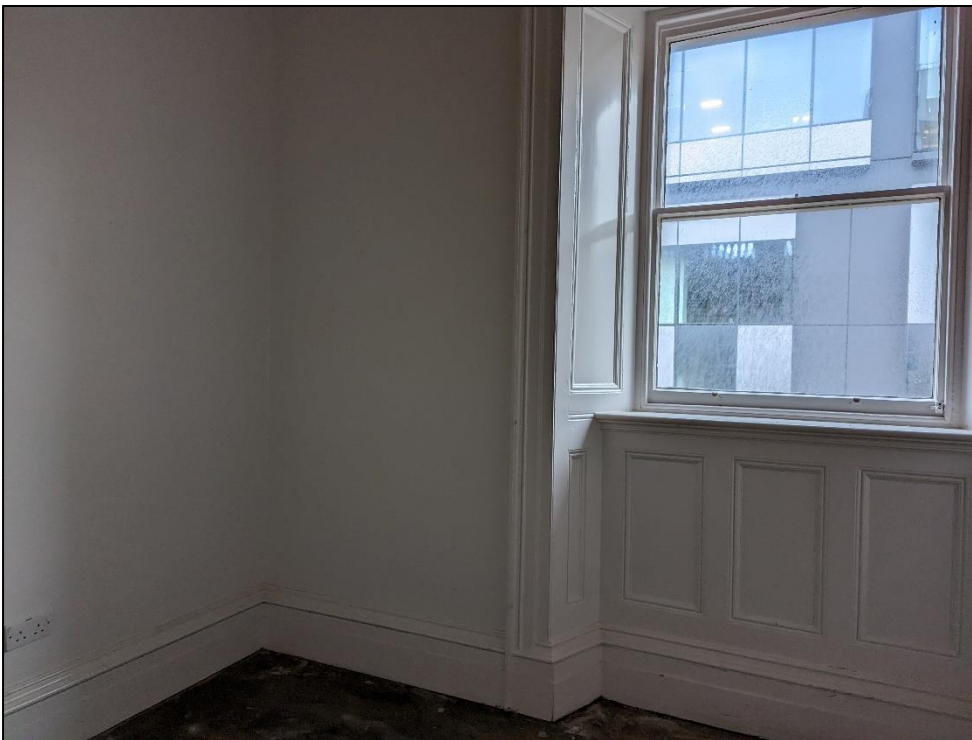
Plate 87: Detail of office window showing surround
