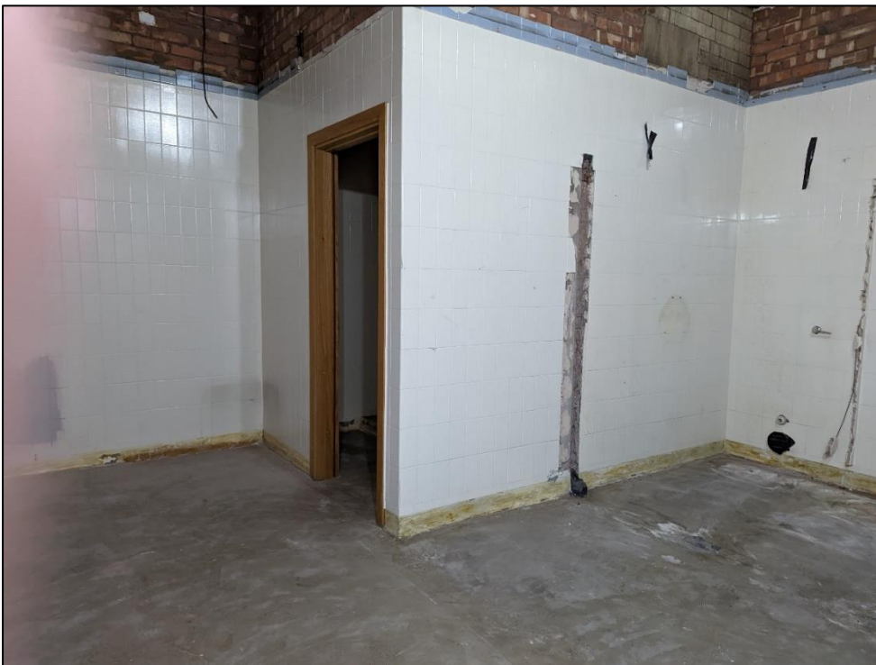
Plate 46: Stripped out WC no north end of extension
