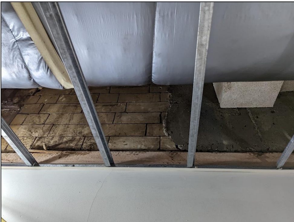
Plate 113: Detail of glazed bricks
