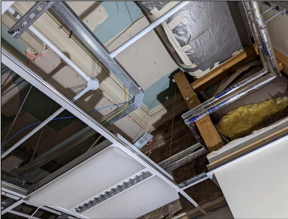
Plate 51: Detail of ceiling showing cornice in room shown above
