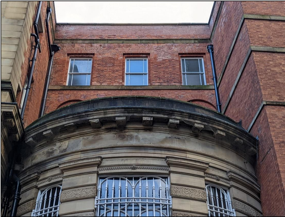
Plate 21: Detail of second and third floors
