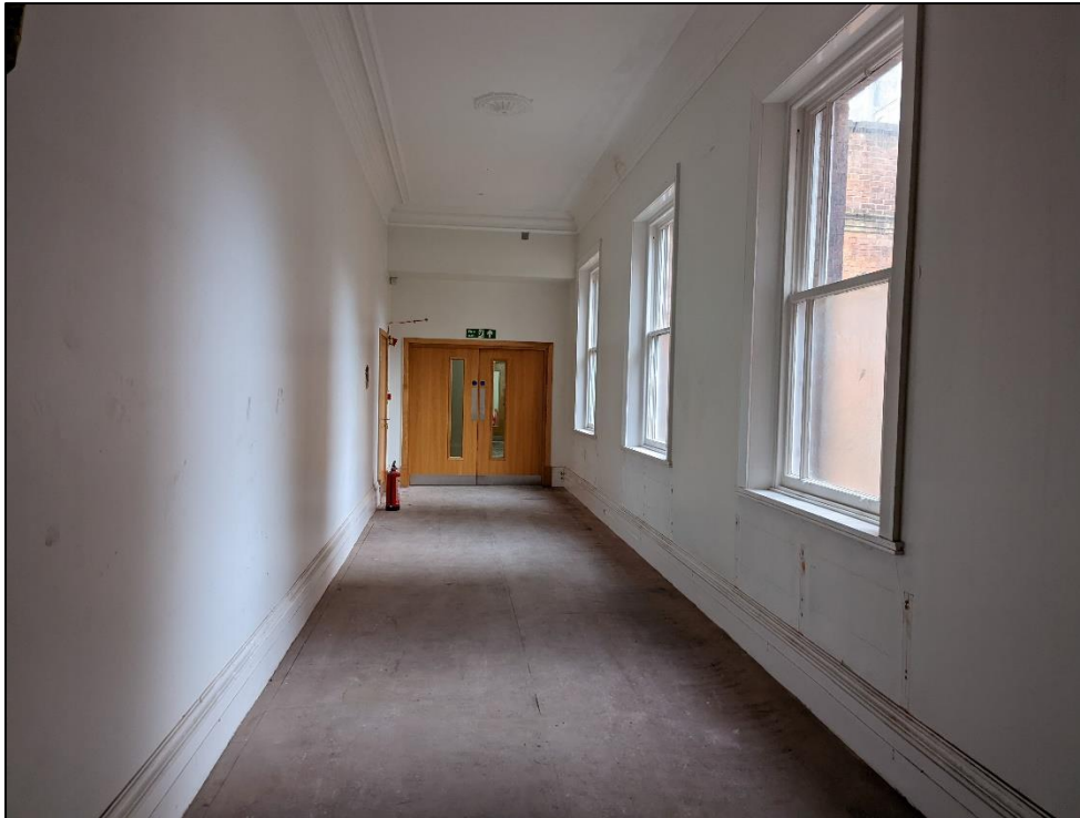
Plate 94: Corridor to west end of original building
