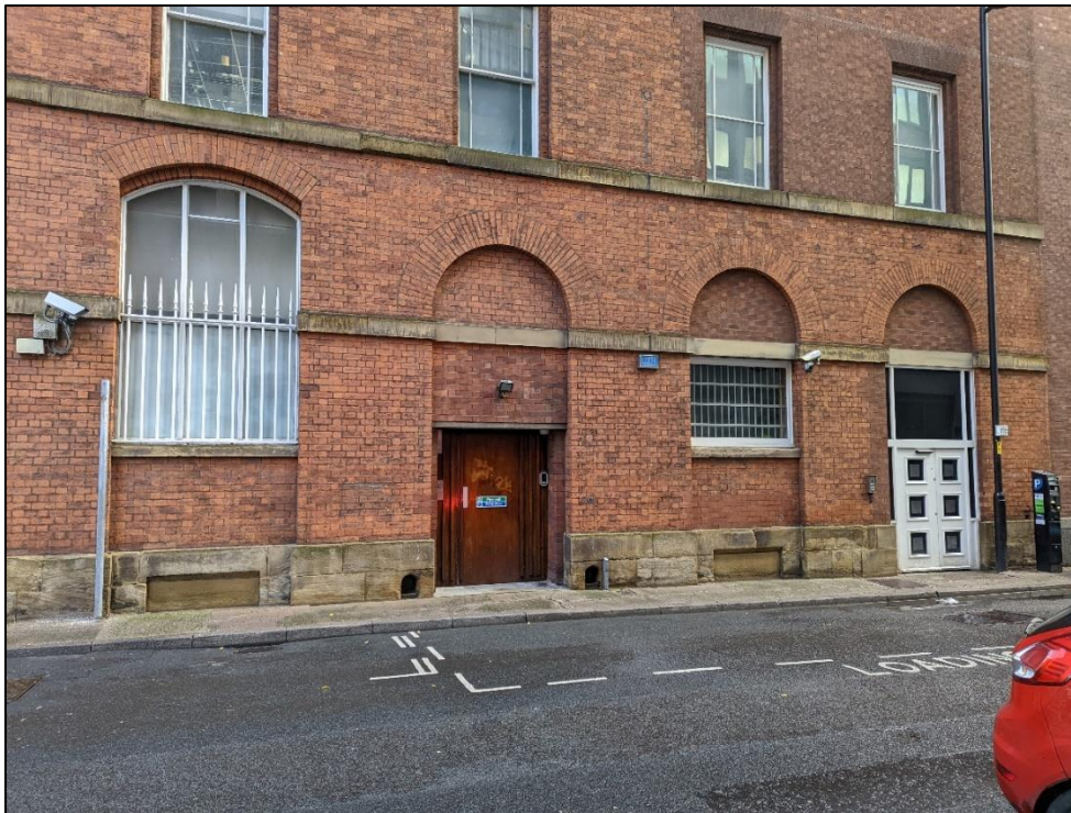
Plate 23: Ground floor detail
