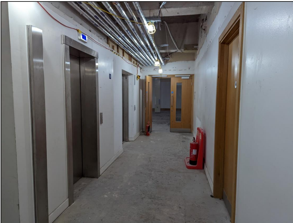
Plate 75: Inserted lift bank to extension
