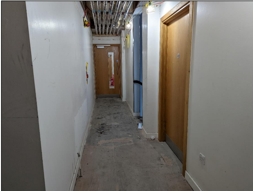
Plate 96: Corridor continuing south from corridor shown above
