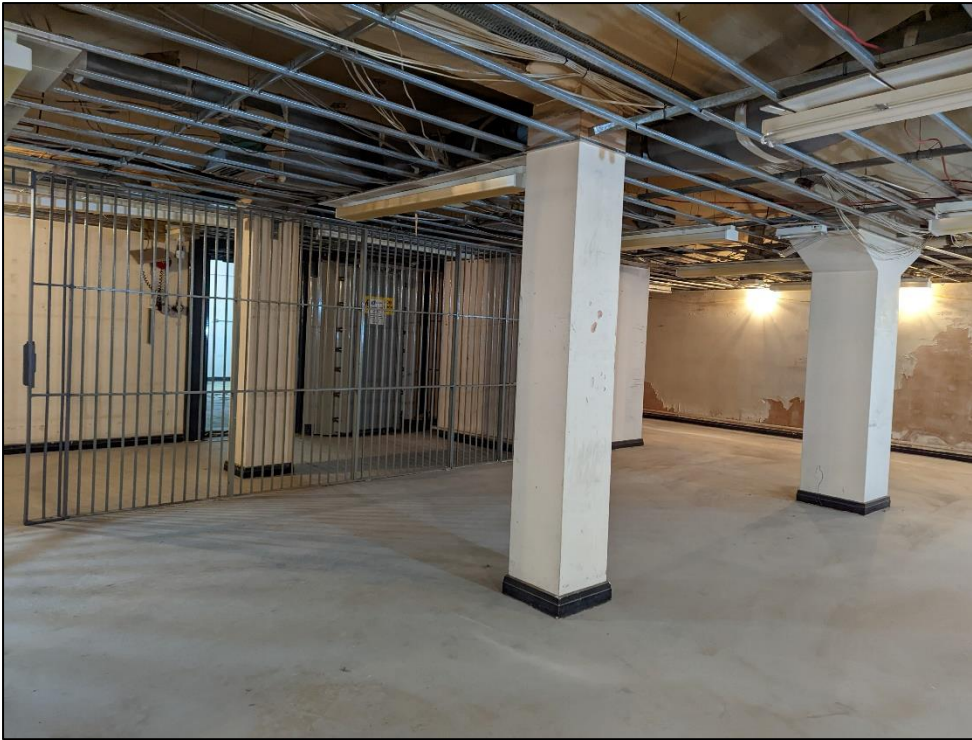
Plate 110: Southern room of original building
