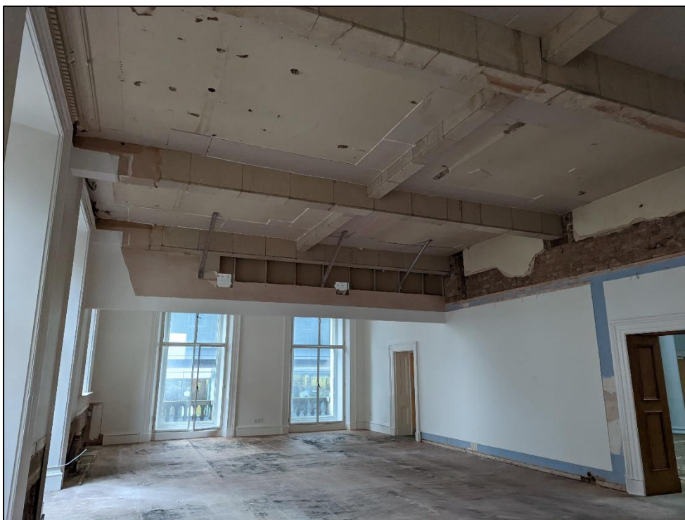
Plate 65: General shot of room
