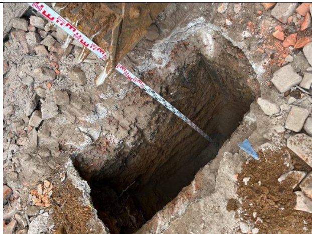
Trial Pit 01: Overview of excavation
