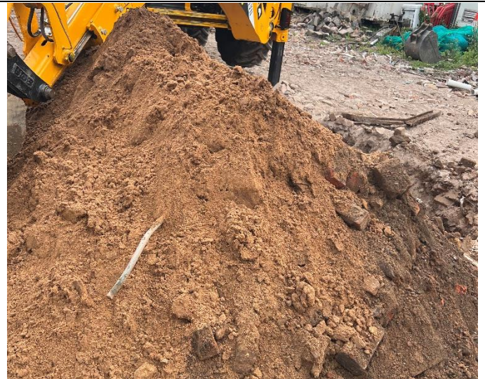
Trial Pit 03: Overview of excavated soils
