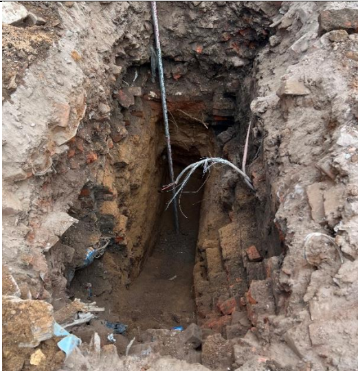
Trial Pit 03: Overview of excavation
