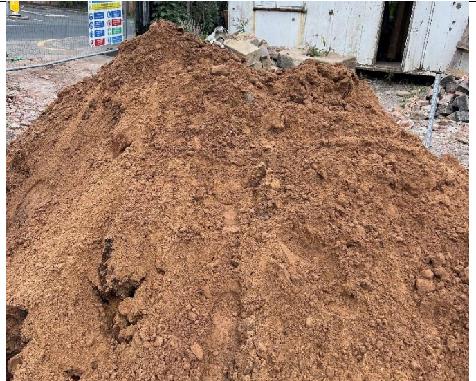
Trial Pit 04: Overview of excavated soils
