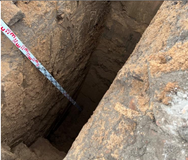
Trial Pit 04: Overview of excavation
