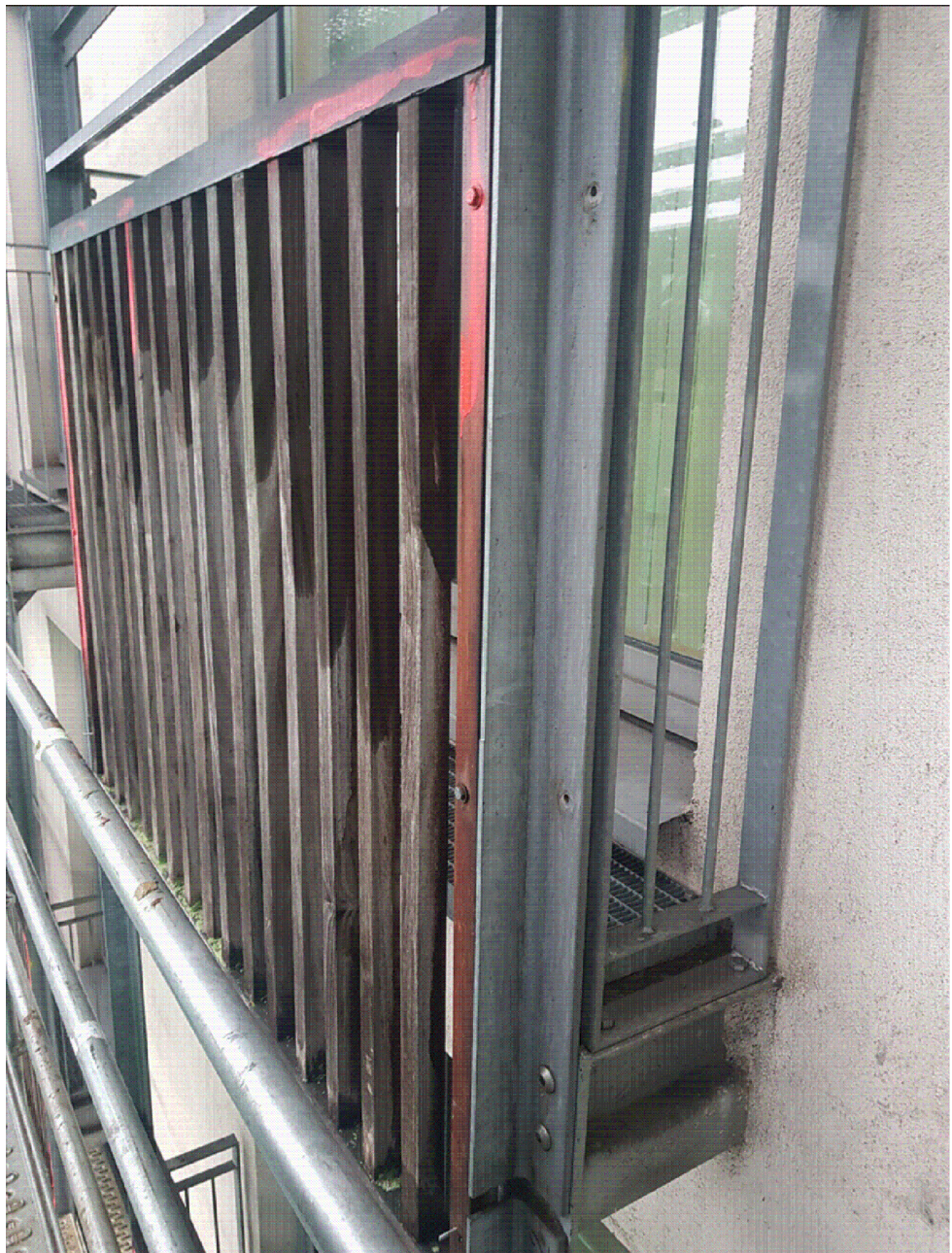
Photograph showing existing timber trellis and fixing
